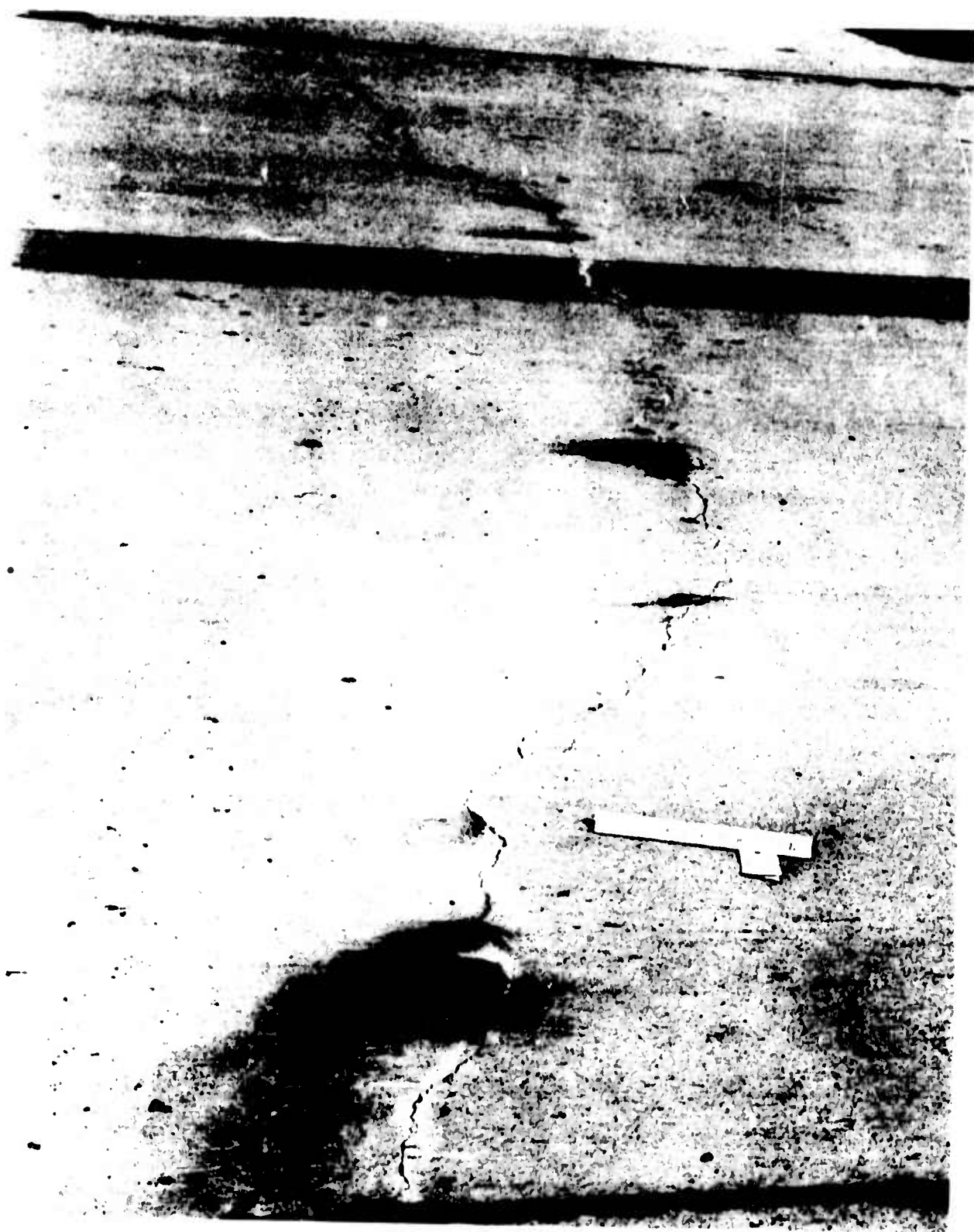
Figure A-15. Typical unsealed transverse crack in Hardstand Taxiway 1, Ban U-Tapao Airfield.
