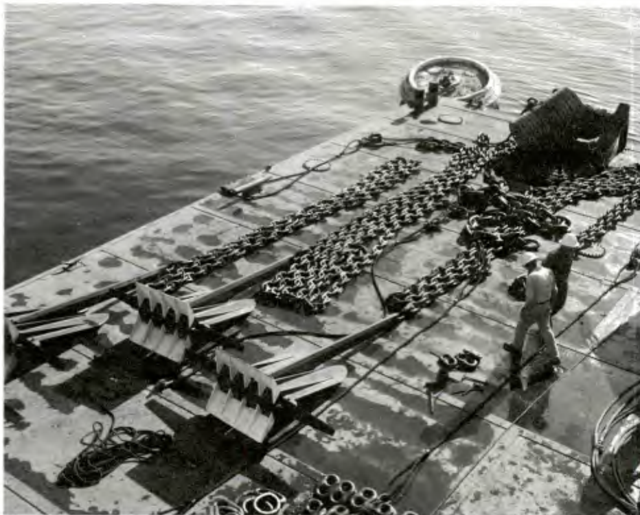
Figure 5. Installing 3,000-pound anchors in BM 18 at San Diego Bay.
