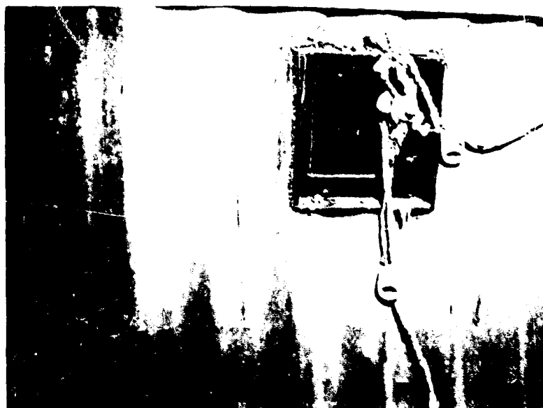
Figure 9. Closeup view of window to the photography tunnel after the fire (Trial 1).
