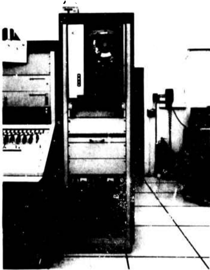
Figure 2.53 Incremental recorder interface and power supply equipment.
