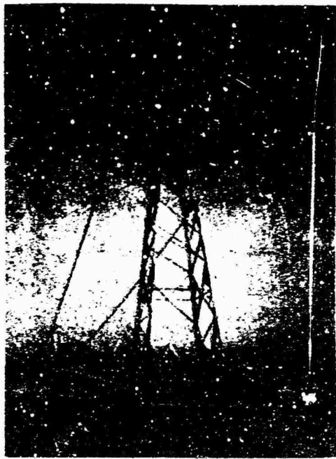
(a) 800-kV dc Test Line
