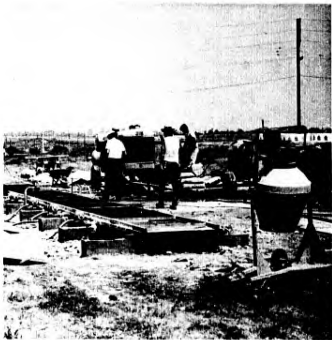
Figure 2-4 Turbo-Vibrators Attached to Form Bed
