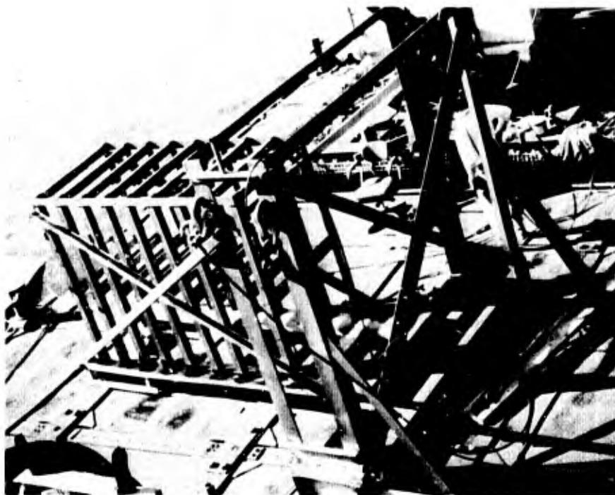
Figure 3-16 Structural Steel Support Frame For Panels and Pier Simulator
