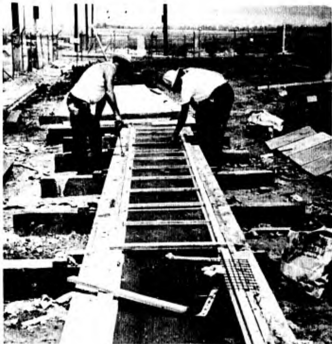
Figure 2-3 Multi-Panel Form Bed, 27½"x27½"x1" Panel Forms
