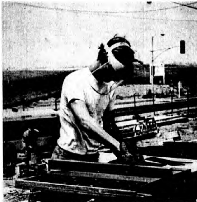
Figure 2-1 Cutting of Reinforcement
