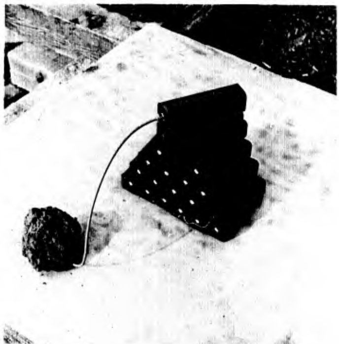
Figure 3-6 Placement of Surface Blast Charge
