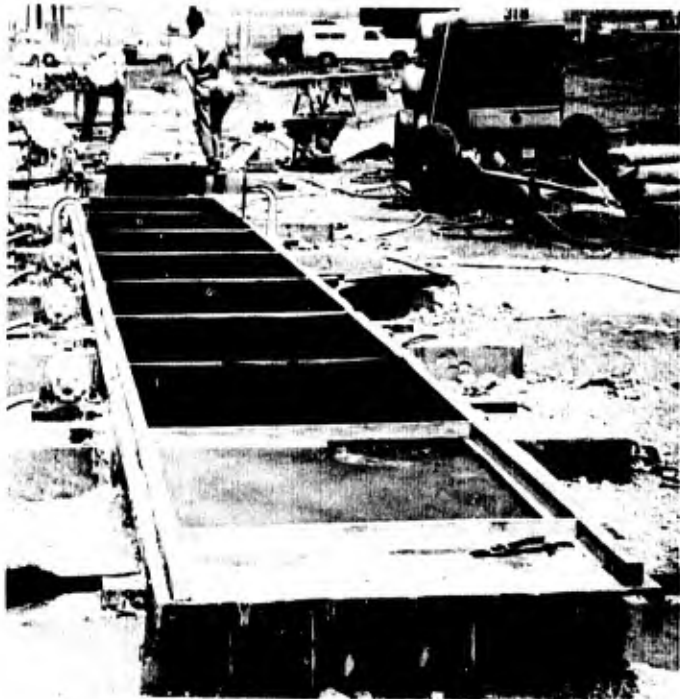
Figure 2-2 Multi-Panel Form Bed, 41½"x41½"x2" Panel Forms
