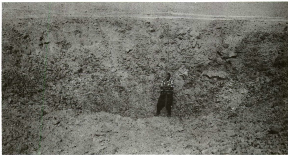
FIG. 6. Crater Formed by Detonation of Single 10,000-Pound Charge.
