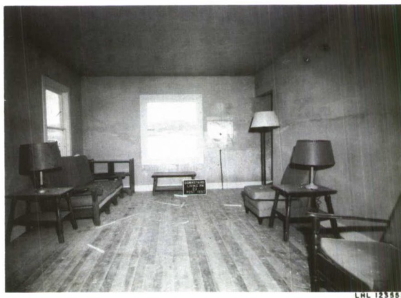
FIG. 13. Living Room Damage, Test No. 1.
