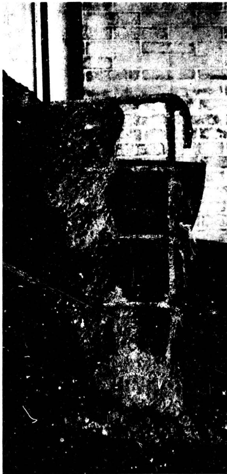
Figure 11. Ferrous oxide on zinc-coated steel bars - east end of Wall 101.
