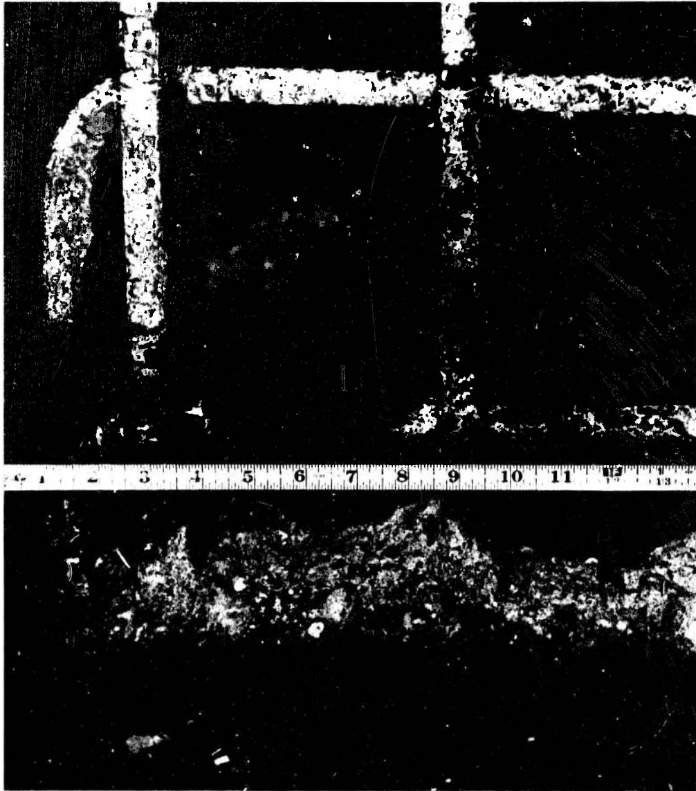
Figure 13. Steel exposed for Wall 103. Dark areas are ferrous oxide. Lower bar is opposite horizontal crack in Figure 12.
