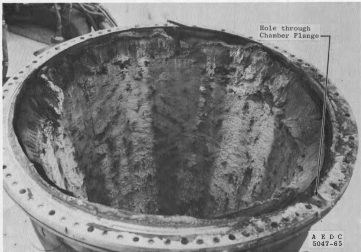
Fig. 24 Postfire Condition, Chamber S/N 213
