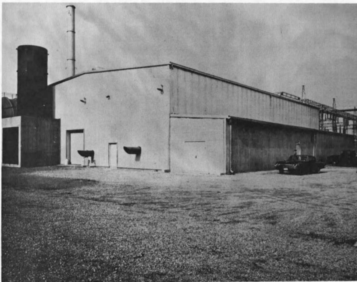
Fig. 88 External View of LORHO Pilot Facility
