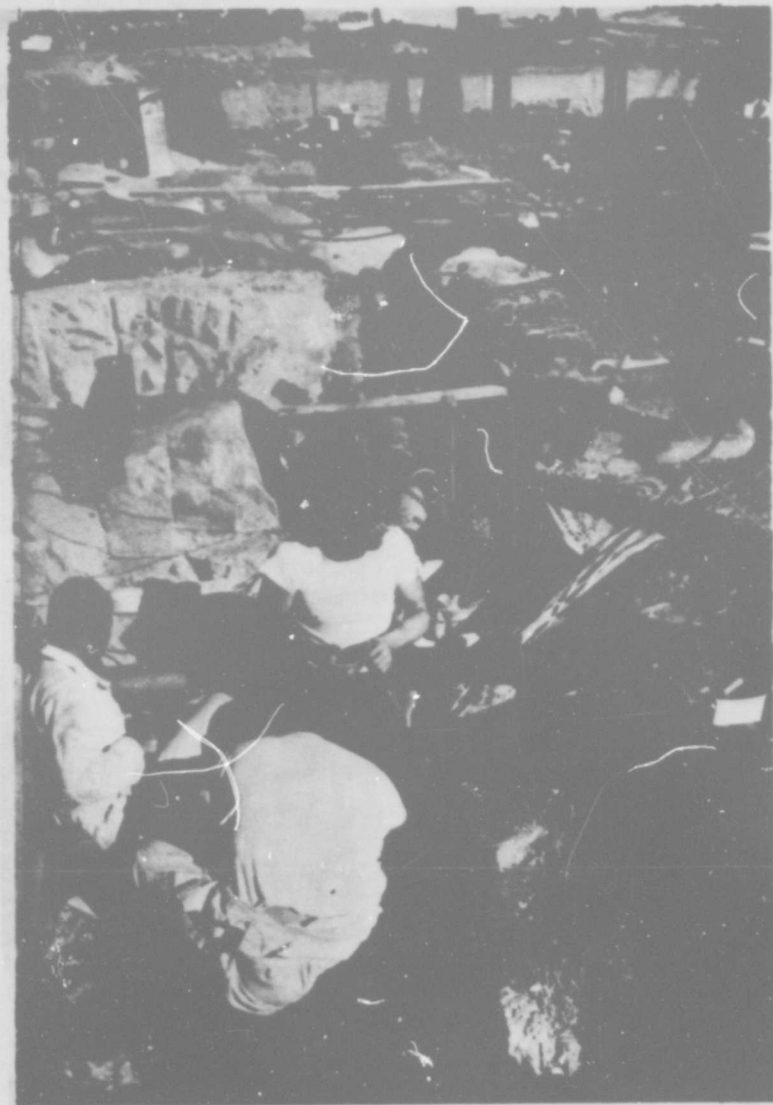
Figure II-26. AFWL Personnel Installing Instrumentation.
