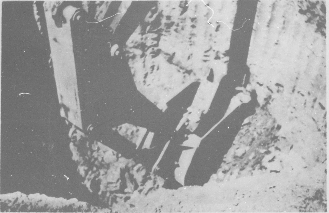
Figure II-42. Excavating Full Scale Model.
