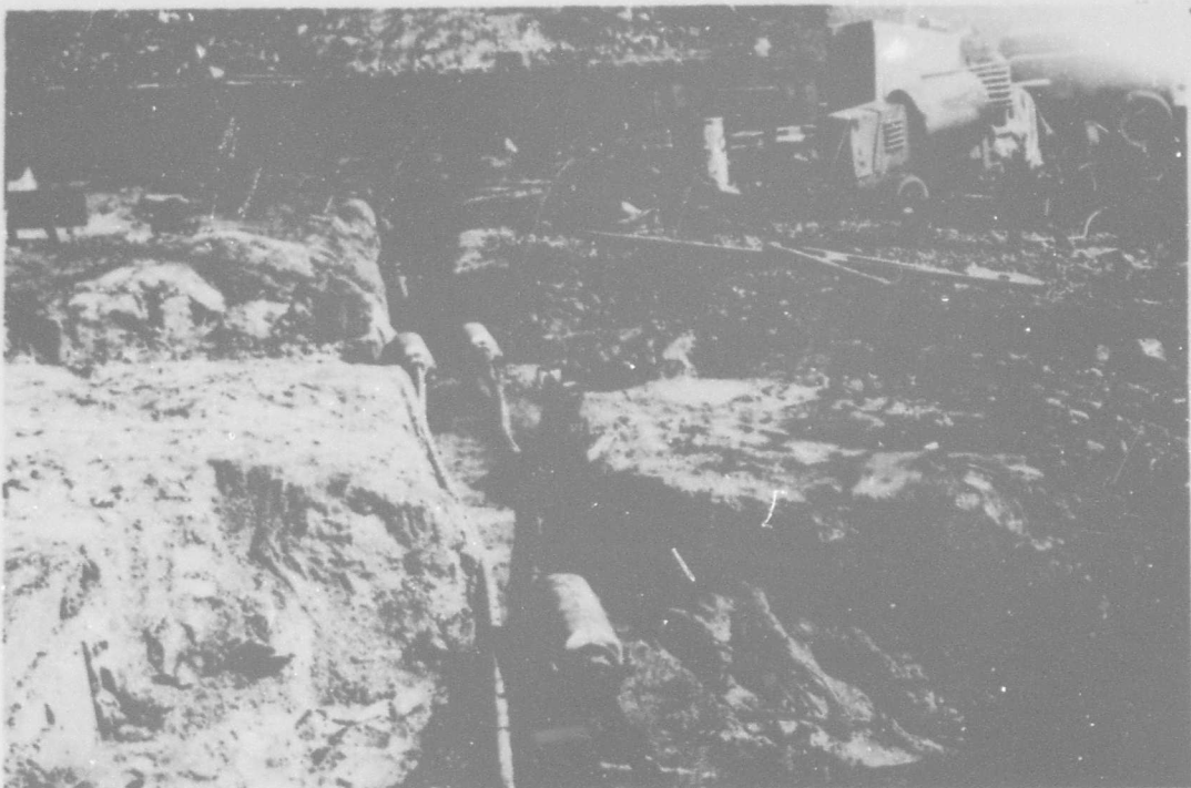
Figure II-24. Rock Excavation for Government Installed Splice Cases.
