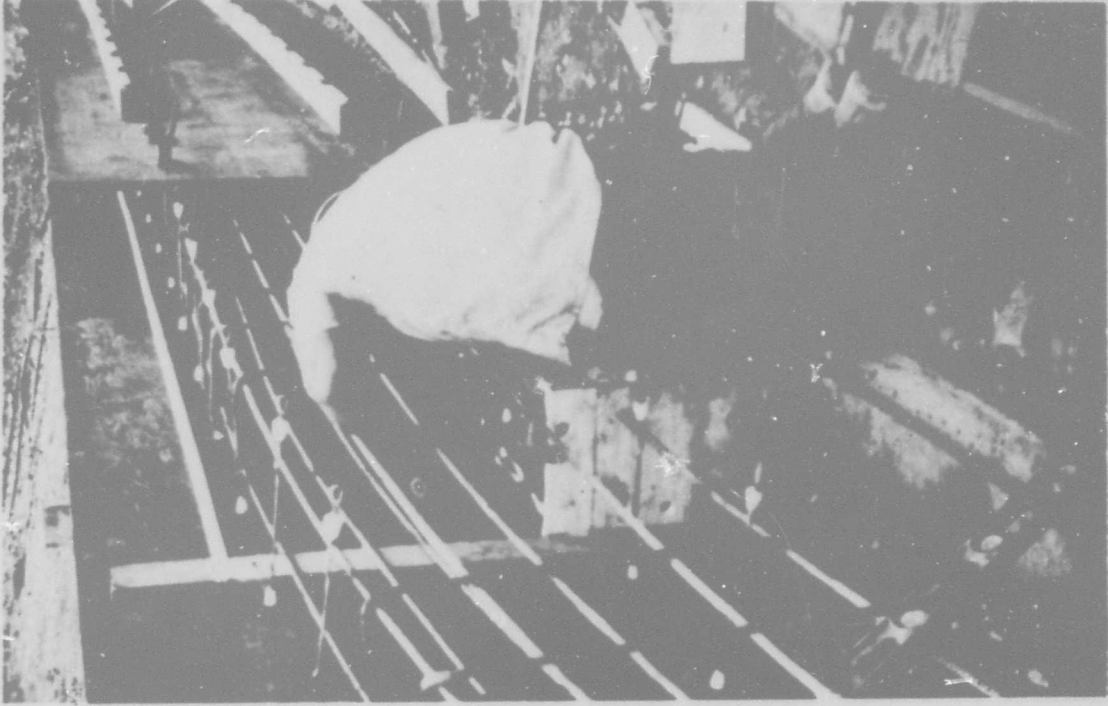
Figure II-9. Reinforcing Steel Placement for Concrete Perimeter Walls.
