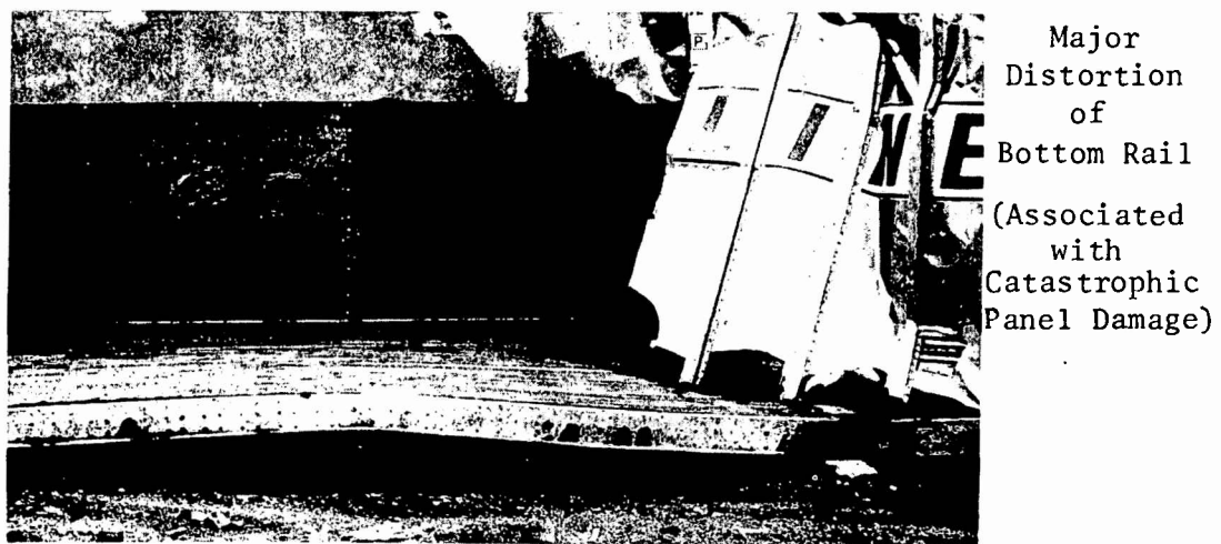
Figure 5-5. Typical Bottom Rail Damage
