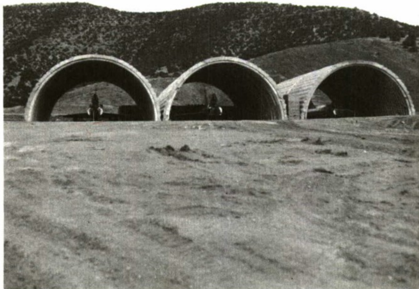
Figure 4. Completed Test Facility
