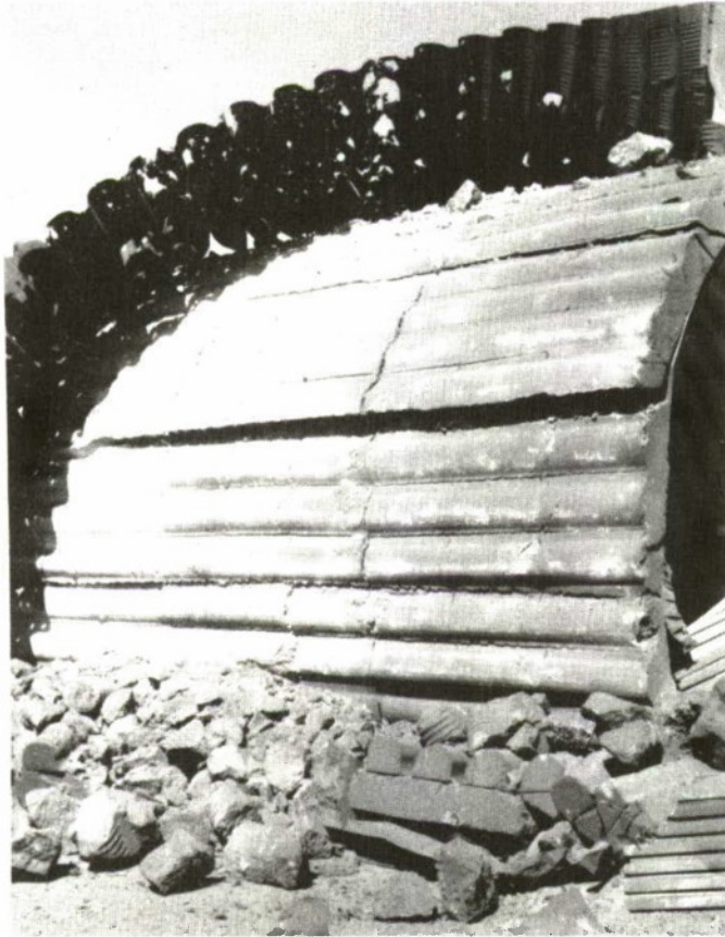
Figure 14. Exterior View of Shelter A
