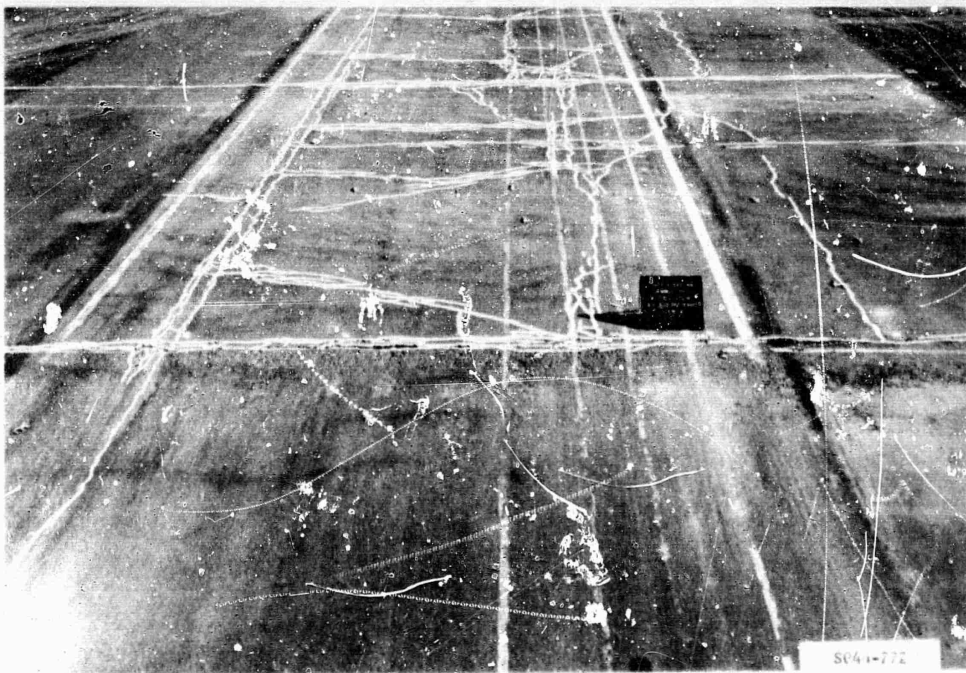
Figure 30. Crack Pattern in Nonrigid Overlay of Item 4, South Lane, at Conclusion of 12-Wheel-Assembly Traffic
