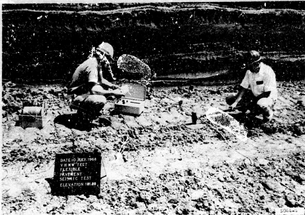
Figure 55. Refraction Seismic Test at the Bottom of the Excavation
