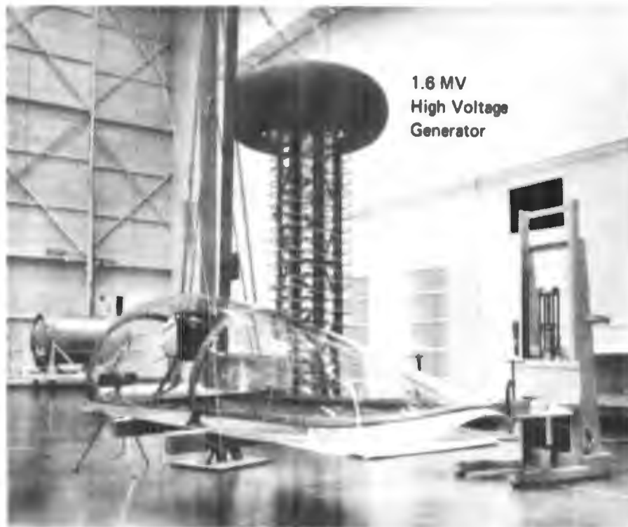
FIGURE 16 HIGH VOLTAGE GENERATOR AND CANOPY - SIDEVIEW
