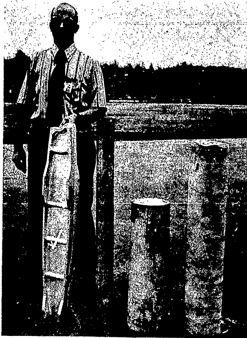
PRODUCTION SEQUENCE FOR P/M DIE FORGINGS RIGHT TO LEFT: GREEN COMPACT; HOT PRESSED COMPACT; EXTRUDED STOCK; FORGING.
