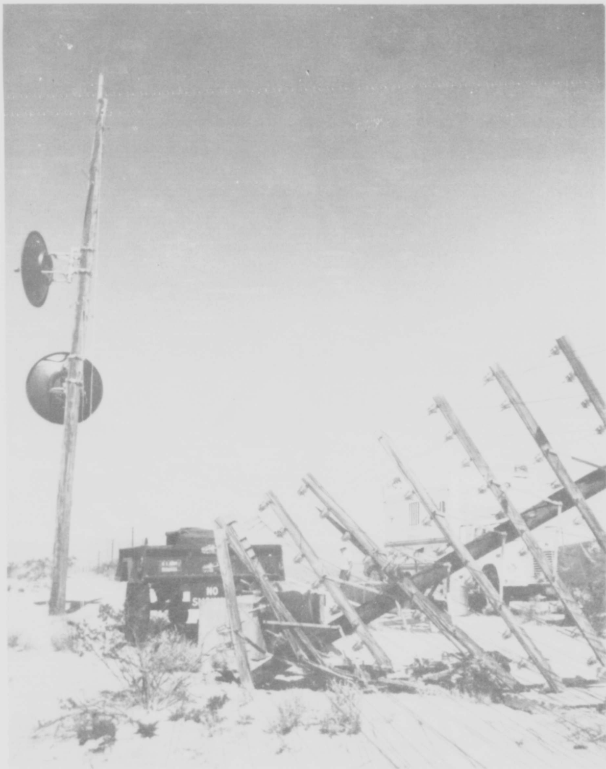
Figure 80 South Pole Movement as a Result of Wind Damage
