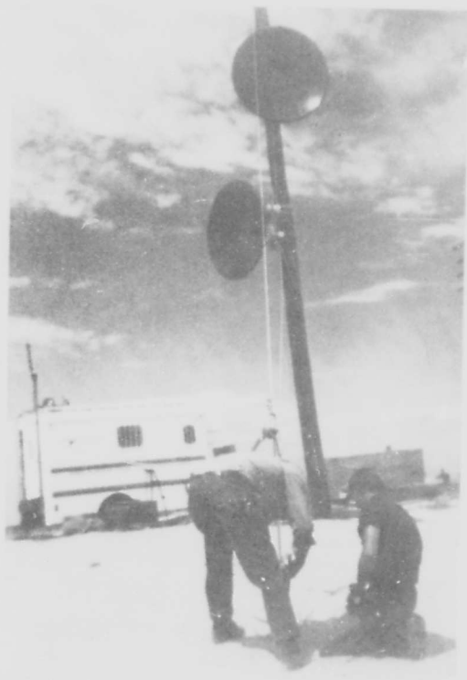
Figure 82 WSMR Engineers Straightening South Pole
