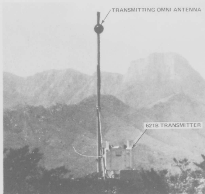
TRANSMITTER SITE TYPICAL (SHOWN AT POSITION ONE)
