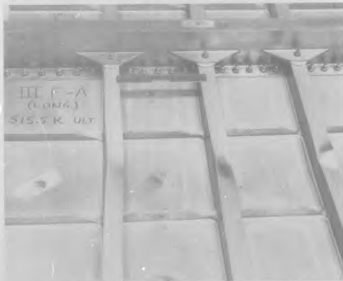
FIGURE 22.—POSTFAILURE PHOTOGRAPHS OF TYPE III F PANELS
