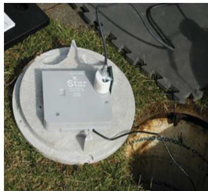
Meter Transmitter Unit
