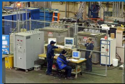
Power Conditioning Lab
