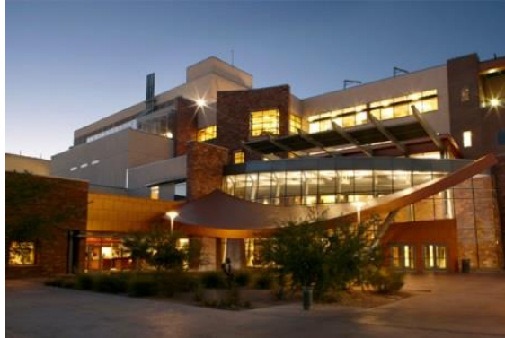
Figure Appendix-1. Exterior of Science and Engineering Building at UNLV
