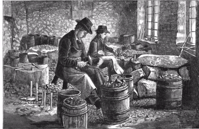
Fig. 13.—Flaker at Work. Boy knapping in background. (From a Photograph.)
