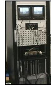
OAR SPIL Open Air Range Signal Processor in the Loop
