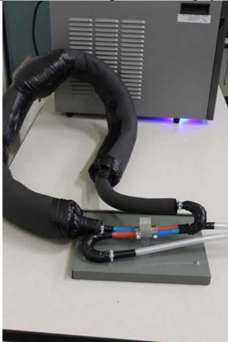
Figure B.A.4. Completed cooling system
