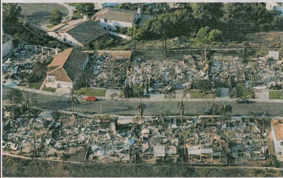
SAN DIEGO A neighborhood in the Rancho Bernardo section was left in ruins yesterday after a fire raced through.
