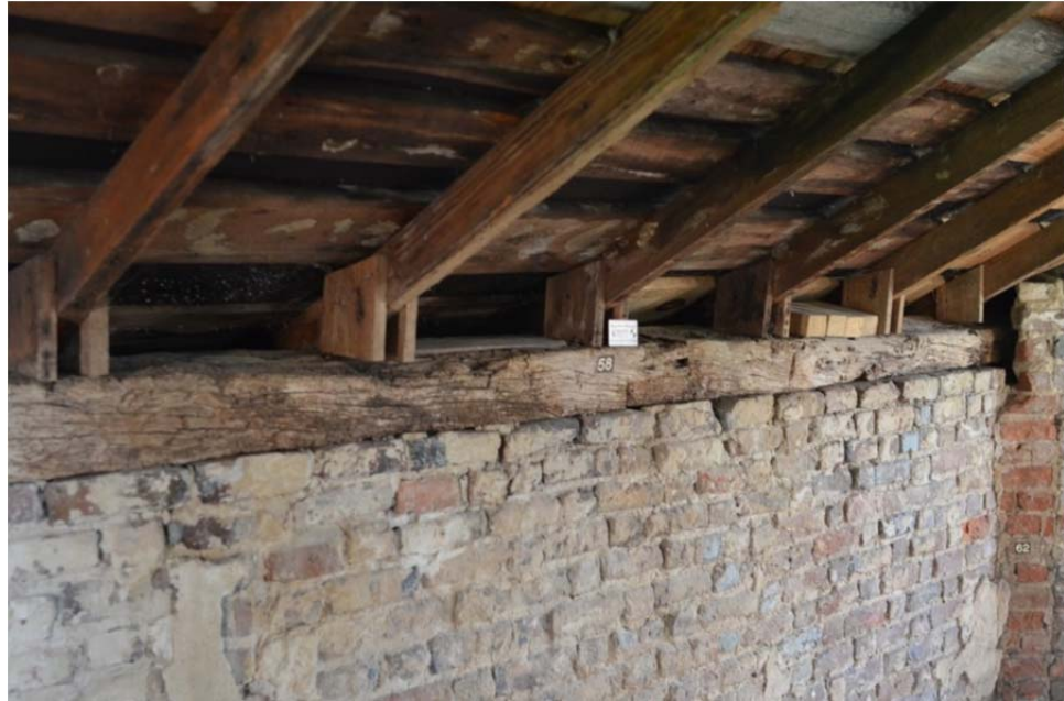
Figure 6. Exposed rafters and sheathing in rear chamber exhibiting signs of past and ongoing water damage. (NCPTT, 2015)
