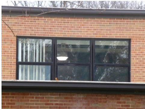
Original clerestory opening with replacement anodized-bronze aluminum windows (ERDC-CERL, 2013).
