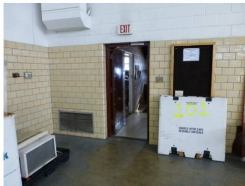
Original glazed sanitary tile walls in the drill hall (ERDC-CERL, 2014).
