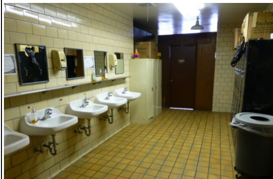
Original glazed sanitary tile walls in the latrines (ERDC-CERL, 2014).
