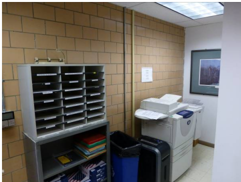
Original glazed sanitary tile wall in the locker room (modified into office space) (ERDC-CERL, 2013).
