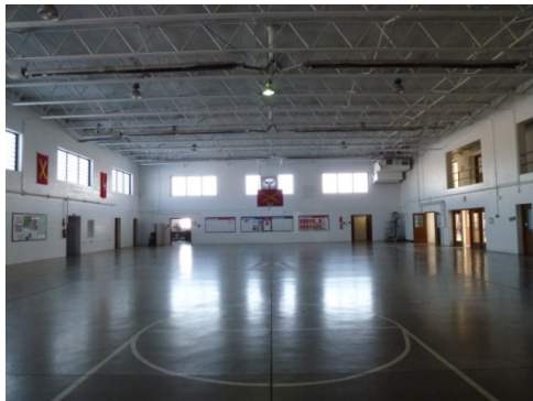
Interior view of the drill hall with concrete floor, combination of concrete-block and glazed sanitary tile walls, flat roof, exposed truss system (ERDC-CERL, 2014).
