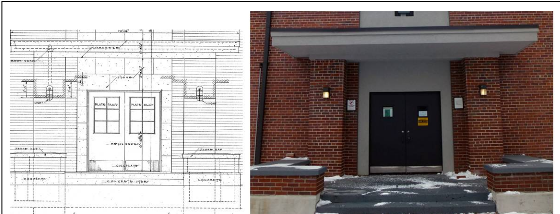
Close-up North main entry on the east (front) elevation: original design and materials: flat canopy, stone-capped bench/half walls, light fixtures, metal and glass windows, and stone tiles framing the entry bay on the left (1950 drawing), compared to the current replacement one-over-one anodized-bronze aluminum window, replacement entry doors, and replacement light fixtures on the right (ERDC-CERL, 2014).
