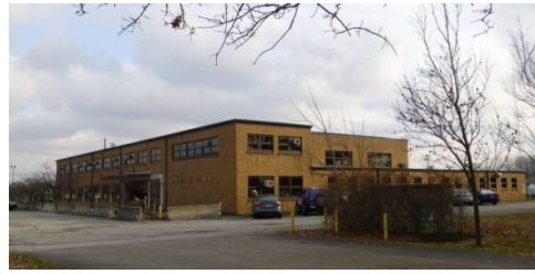
Cleveland-Brook Park OHARNG Armory (1957) – Type C.
