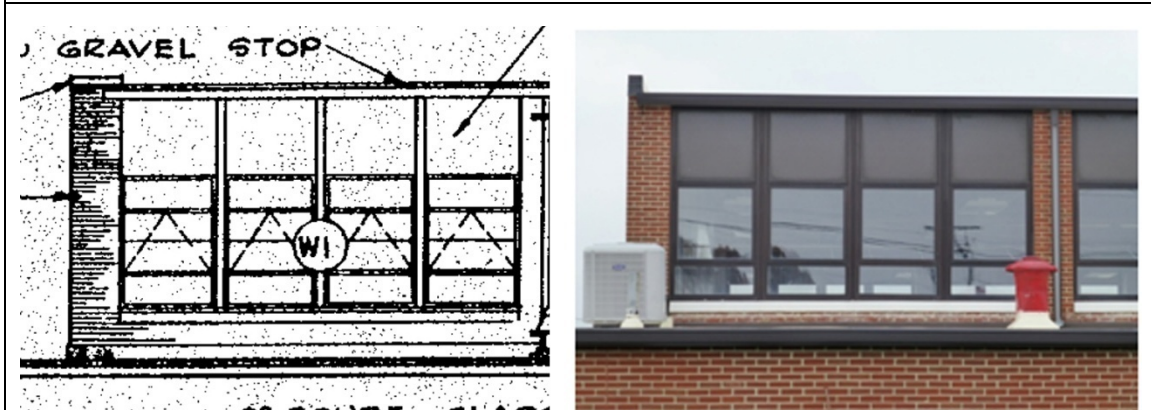
Clerestory windows on the east and west elevations: original design and materials with four-pane awning windows with laminated porcelain enamel panels above on the left (1952 drawing), compared to the current condition, replacement one-over-one anodized-bronze aluminum windows and fiberglass panel inserts above on the right (ERDC-CERL, 2014).
