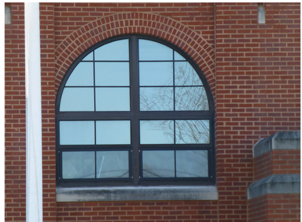
Arch windows on the north (front) elevation : original design and materials with multipane steel-sash industrial window on the left (original drawing), compared to the current condition of the elevation with replacement anodized-bronze aluminum window on the right (ERDC-CERL, 2013).
