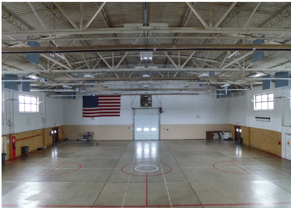
Figure 36. Interior view of the drill hall at Lebanon OHARNG Armory (ERDC-CERL, 2014).
