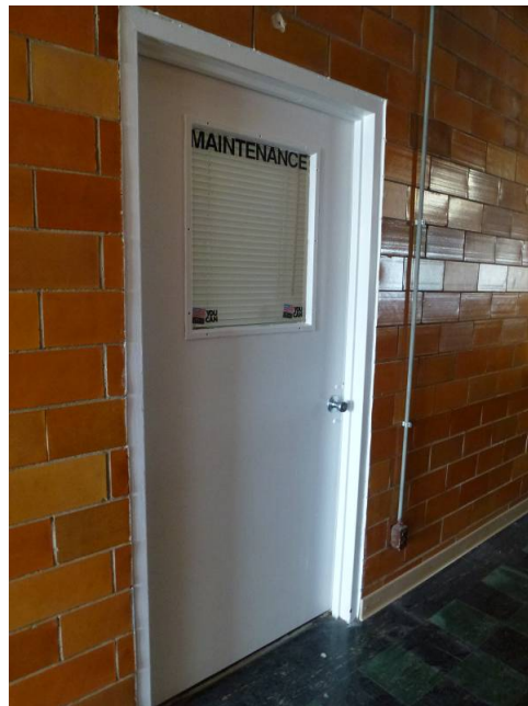
Typical metal and glass office door (ERDC-CERL, 2014).
