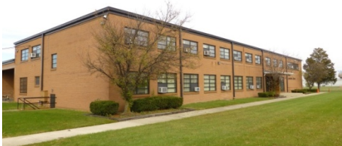
Columbus-Haubrich OHARNG Armory (1958) – Type C.
