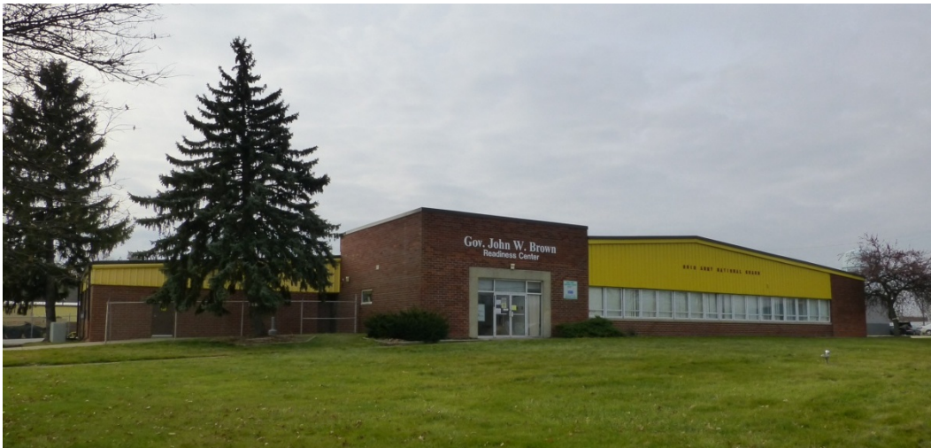
Figure 78. North (front) elevation of Medina OHARNG Armory (ERDC-CERL, 2013).
