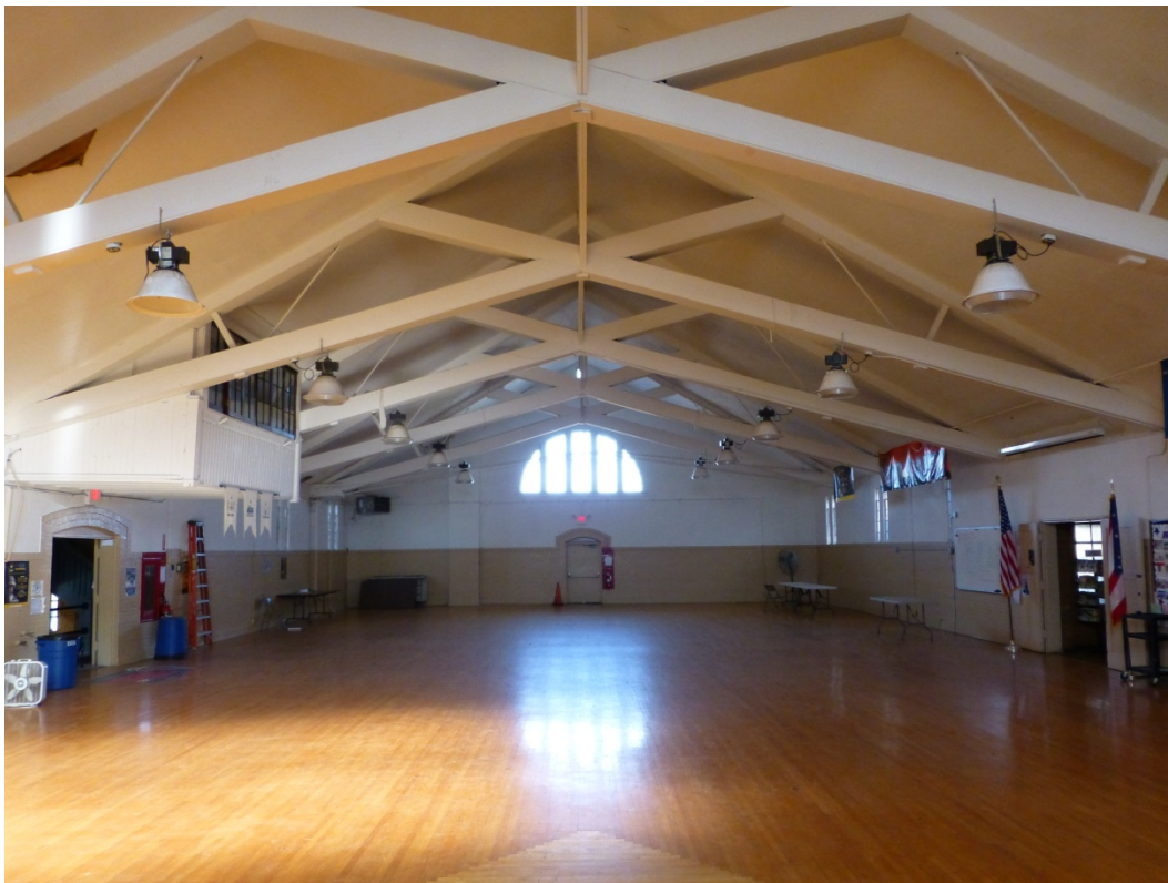
Figure 9. Interior view of the assembly hall at St. Marys OHARNG Armory (ERDC-CERL, 2013).
