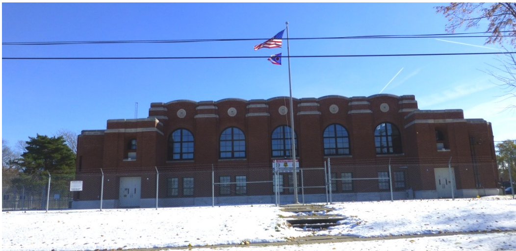
Figure 11. Northwest (front) elevation of Lima OHARNG Armory (ERDC-CERL, 2013).
