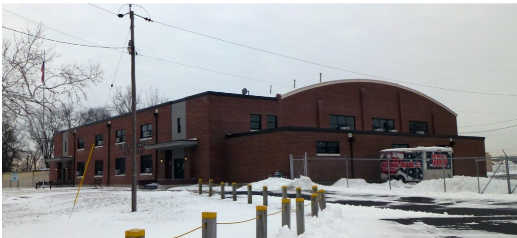
Figure 37. Northeast oblique of Middletown-Kessler OHARNG Armory (ERDC-CERL, 2014).
