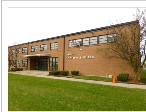
Original ribbon-style window opening with replacement anodized-bronze aluminum windows and original Stainless-steel lettering (ERDC-CERL, 2014).
