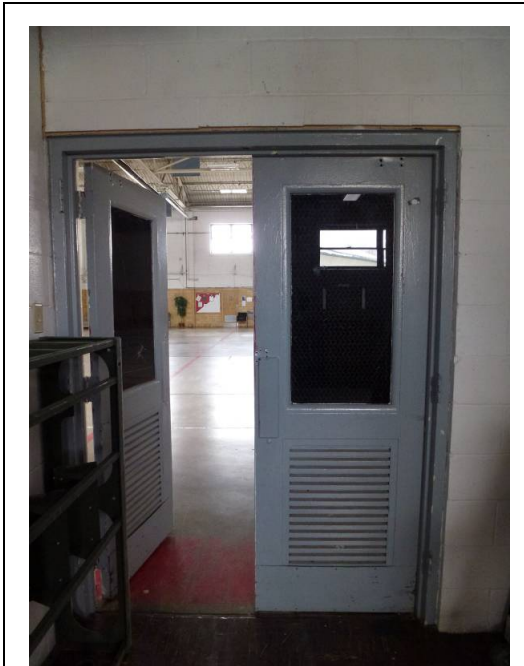
Metal, glass, and louvered vent interior doors (ERDC-CERL, 2014).
