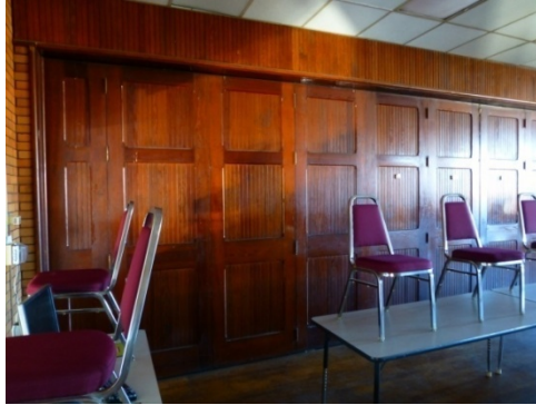
Wood panel pocket doors opening up from the lecture room into the assembly hall space (ERDC-CERL, 2013).
