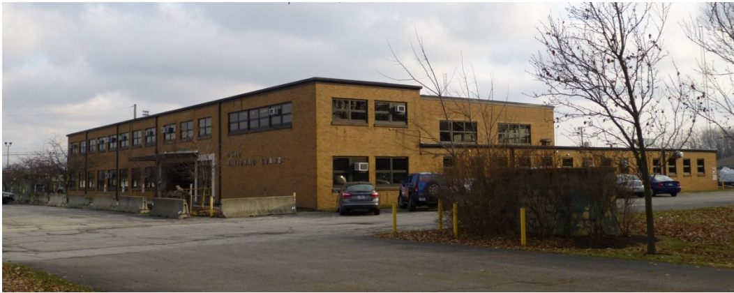
Figure 59. Northeast (front) elevation of Brook Park OHARNG Armory (ERDC-CERL, 2013).
