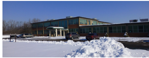
Rickenbacker Army Enclave, Building 930 (1957, acquired in 1996).
