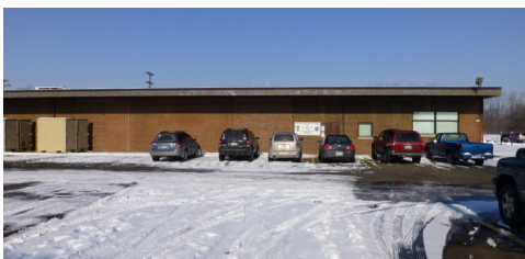
Rickenbacker Army Enclave, Building 933 (1956, acquired in 1996).
