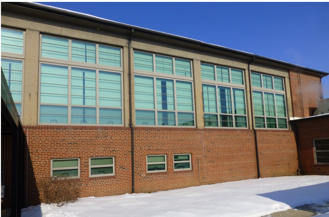
Figure 90. Curtain wall system with replacement windows of Building 930 (ERDC-CERL, 2014).
