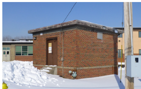
Rickenbacker Army Enclave, Building 934 (1956, acquired in 1996).
