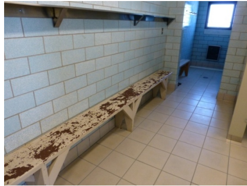
Glazed sanitary tile walls in the latrines (ERDC-CERL, 2014).
