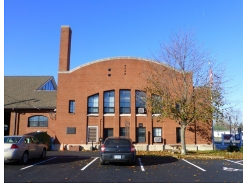
Repetitive window pattern, narrow fenestration, parapet wall, barrel roof (ERDC-CERL, 2013).
