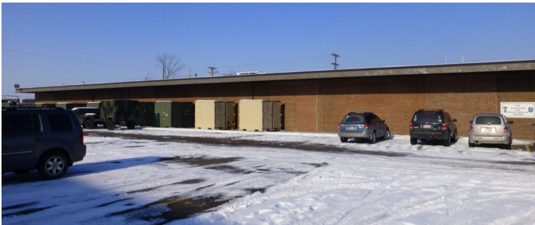
Figure 95. Southeast (front) elevation of Building 933 (ERDC-CERL, 2014).
