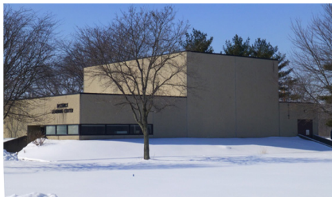
Rickenbacker Army Enclave, Building 944 (1977, acquired in 1996).
