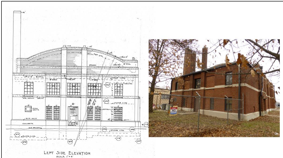
South elevation: original (1937 drawing) on the left and current photograph on the right (ERDC-CERL, 2013). Note that some of the original windows have been removed and filled with brick.
