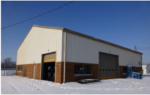
Rickenbacker Army Enclave, Building 929 (1965, acquired in 1996).
