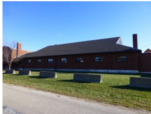
Gable-on-hip roof of the riding stadium (ERDC-CERL, 2013).
