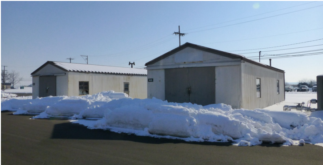
Figure 97. West oblique of Building 935 (right) and Building 936 (left) (ERDC-CERL, 2014).
