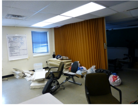
Classroom with original accordion-style divider wall (ERDC-CERL, 2014).
