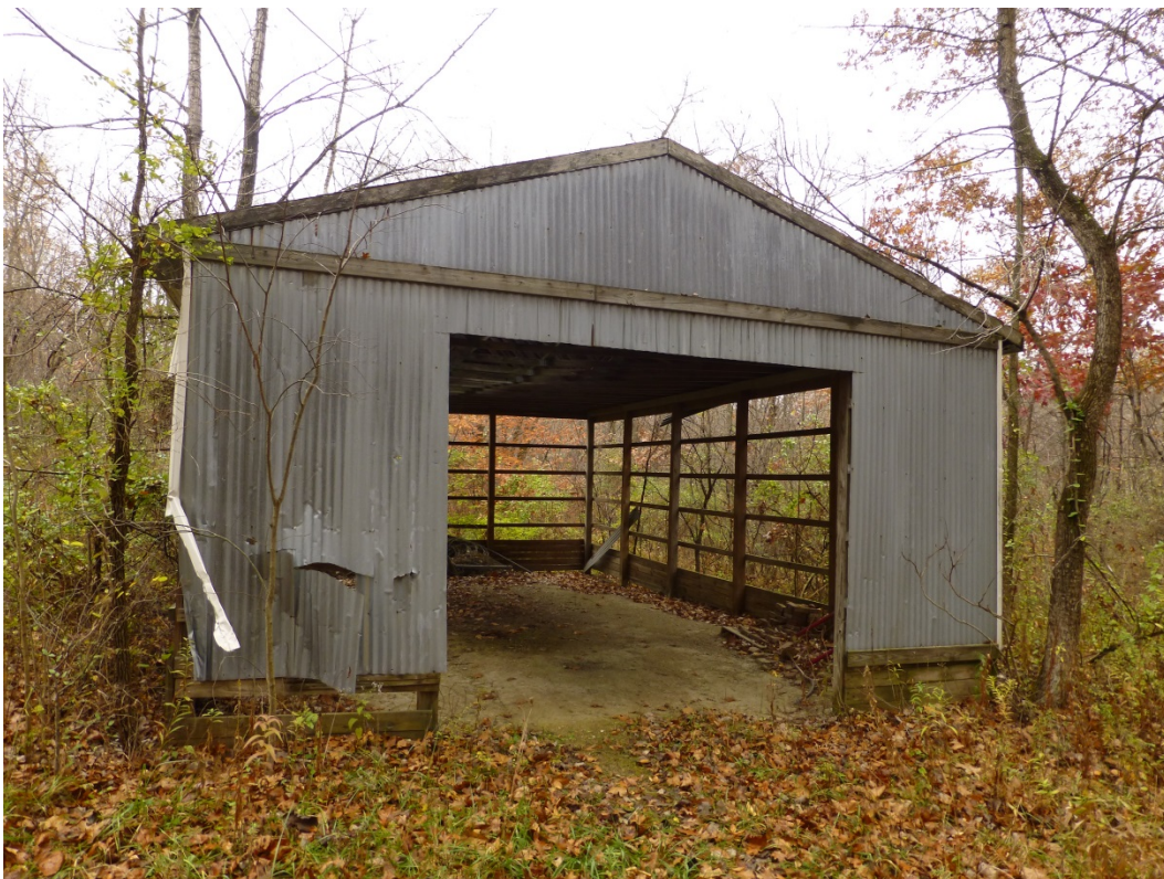
Figure 75. Vacant storage building (ERDC-CERL, 2014).
