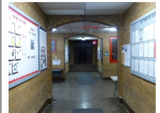
St. Marys OHARNG Armory, interior corridor with brick walls, concrete floor, and arched passageways [drop-ceiling is noncontributing] (ERDC-CERL, 2013).
