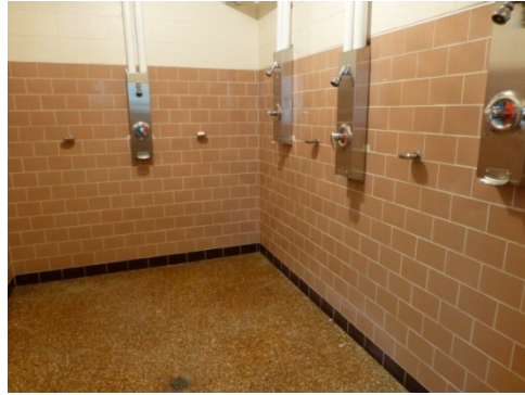
Glazed sanitary tile walls in the latrines (ERDC-CERL, 2013).
