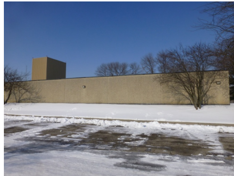
Rickenbacker Army Enclave, Building 943 (1978, acquired in 1996).
