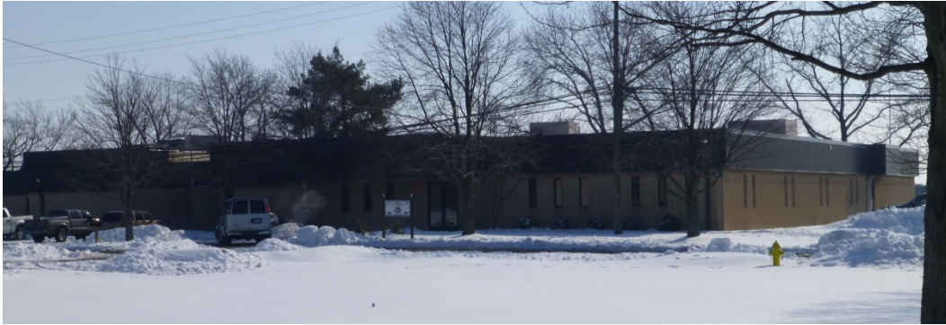
Figure 85. West oblique of Building 920 (ERDC-CERL, 2014).
