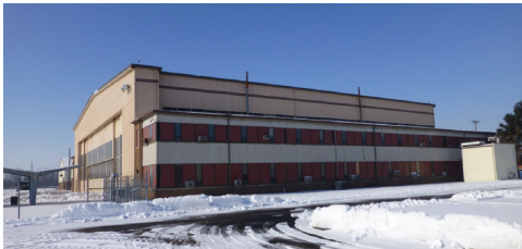
Rickenbacker Army Enclave, Building 931 (1957, acquired in 1996).
