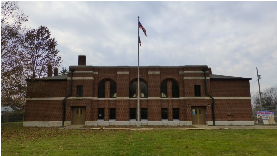
Figure 25. East (front) elevation of Akron-Hawkins OHARNG Armory (ERDC-CERL, 2013).
