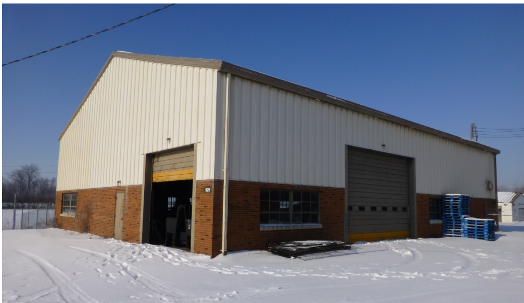
Figure 88. East oblique of Building 929 (ERDC-CERL, 2014).
