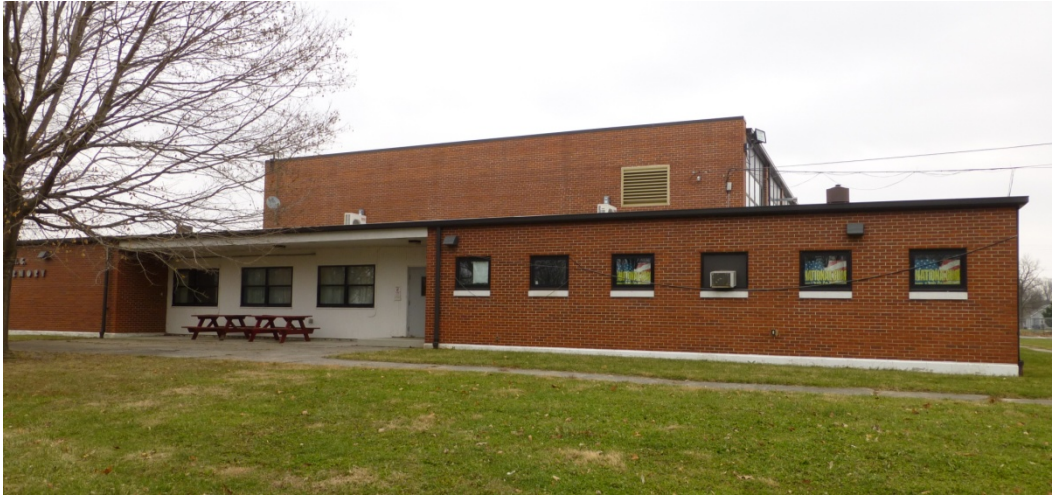
Figure 45. West elevation of Tiffin OHARNG Armory (ERDC-CERL, 2013).
