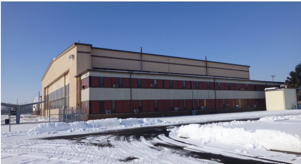
Figure 92. East oblique of Building 931 (ERDC-CERL, 2014).
