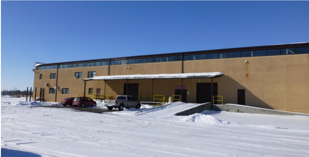
Figure 76. South (front) elevation of Marion OHARNG Armory (ERDC-CERL, 2014).
