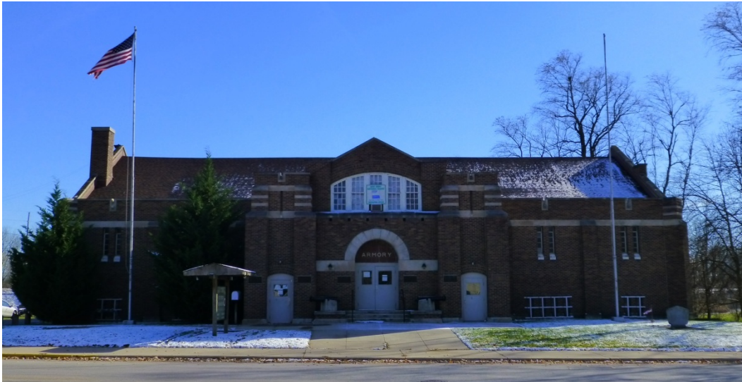
Figure 6. North (front) elevation of St. Marys OHARNG Armory (ERDC-CERL, 2013).
