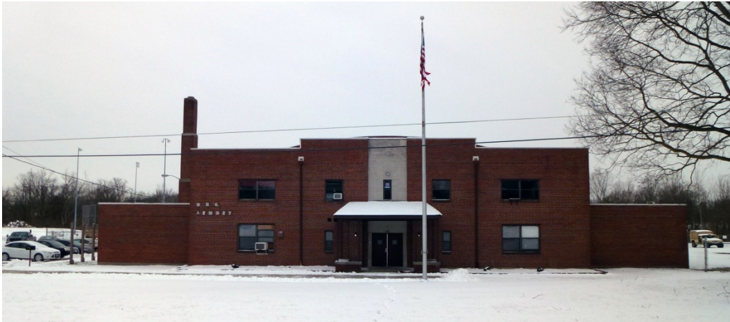
Figure 35. North (front) elevation of Lebanon OHARNG Armory (ERDC-CERL, 2014).
