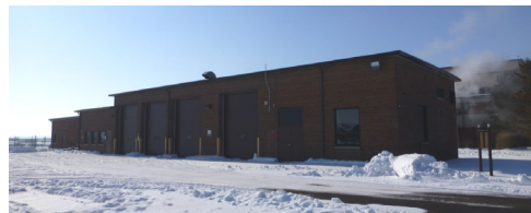
Rickenbacker Army Enclave, Building 932 (1962, acquired in 1996).
