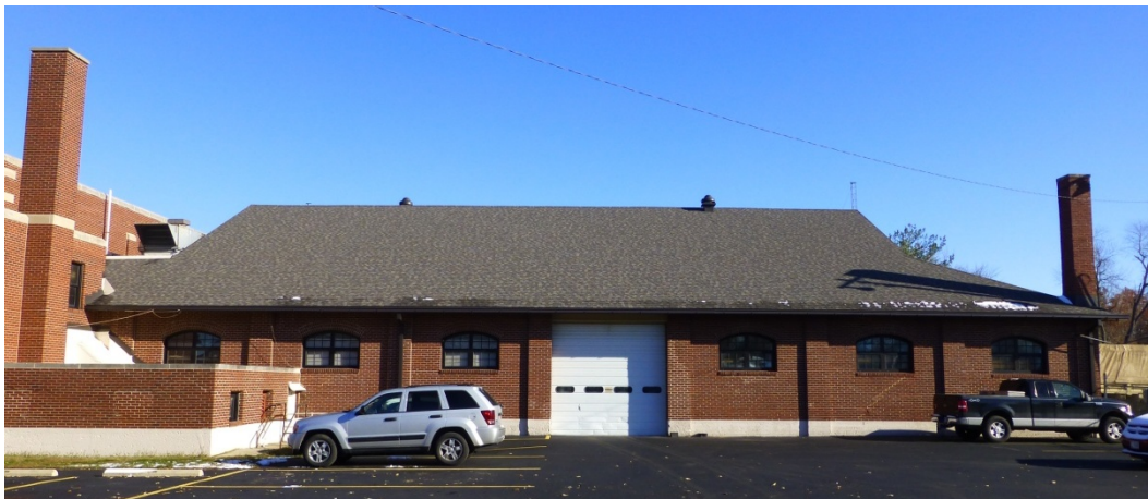
Figure 12. Southwest elevation of the riding stadium at Lima OHARNG Armory (ERDC-CERL, 2013).
