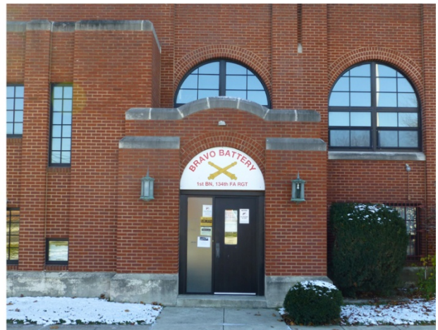
Entry bay on the north (front) elevation: original design and materials with multipane steel-sash industrial windows and metal and glass entry doors on the left (original drawing), compared to the current condition of the elevation with replacement anodized-bronze aluminum windows and metal door with sidelight on the right (ERDC-CERL, 2013).
