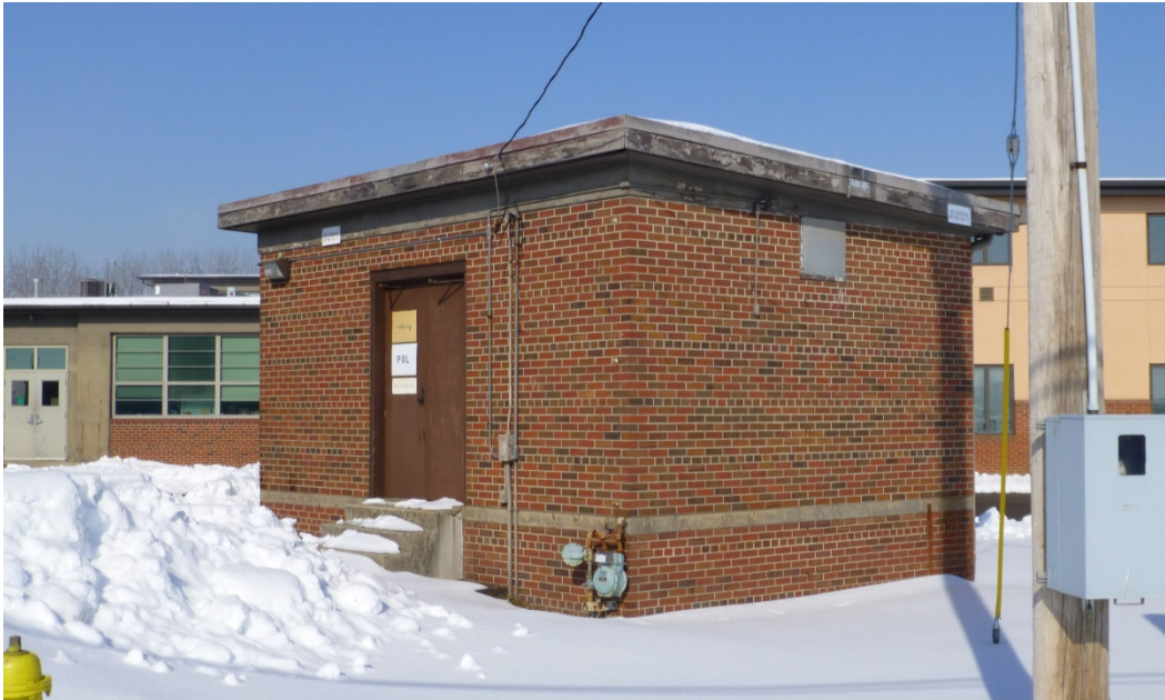
Figure 96. South oblique of Building 934 (ERDC-CERL, 2014).
