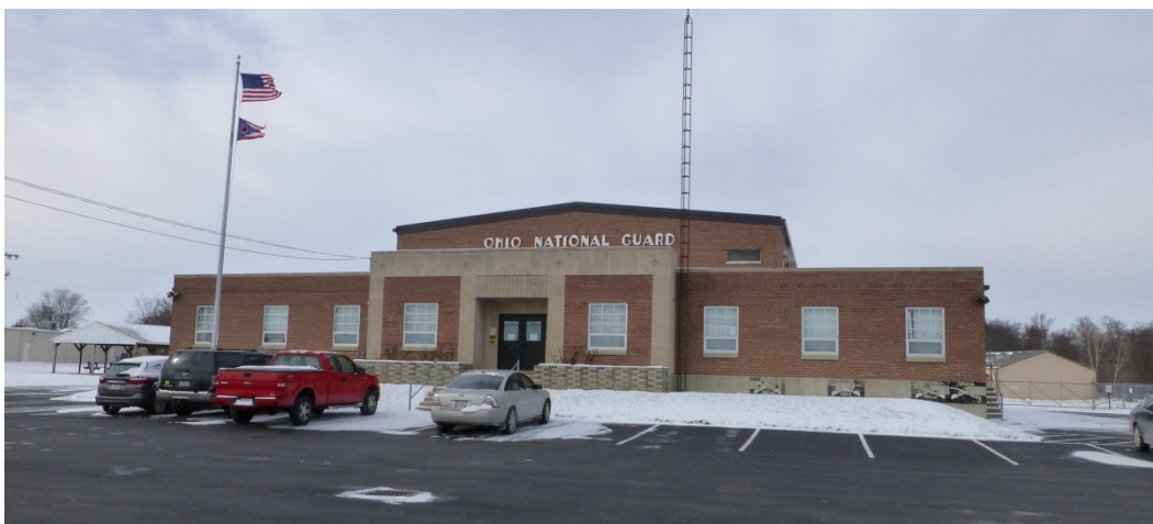
Figure 69. East (front) elevation of Greenville OHARNG Armory (ERDC-CERL, 2014).
