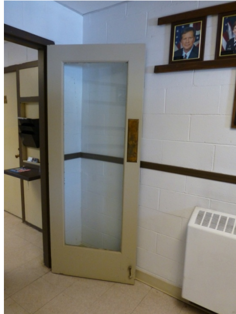
Original metal and plate-glass vestibule doors (ERDC-CERL, 2014).
