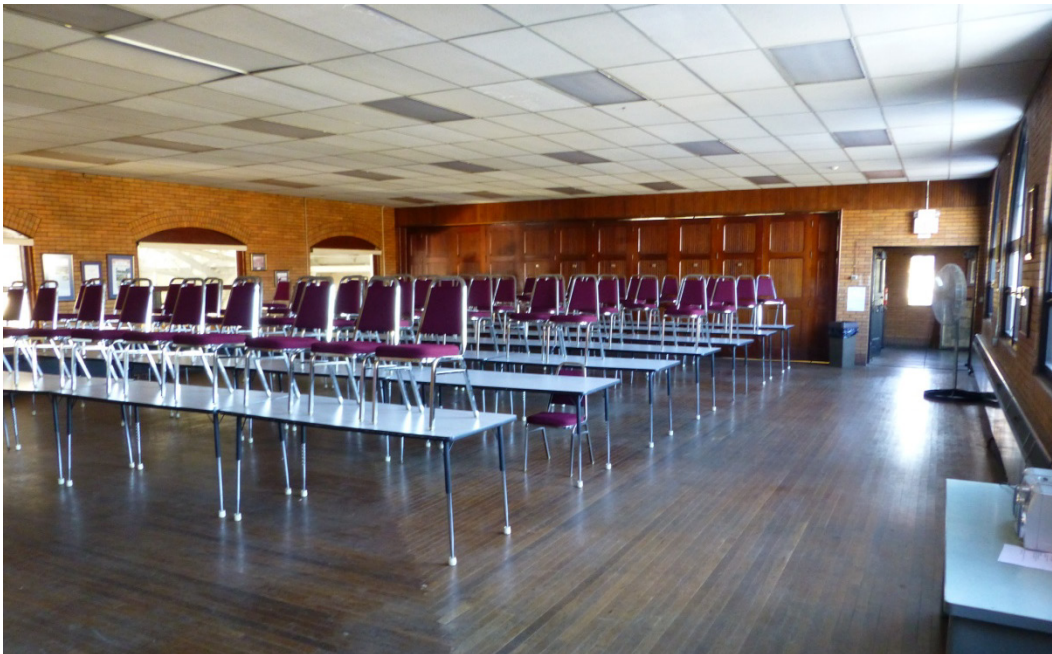
Figure 19. Interior view of the assembly hall at Piqua OHARNG Armory with original window openings on south wall to view into riding stadium and modified drop-ceiling covering the original barrel ceiling (ERDC-CERL, 2013).
