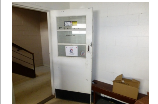
Typical metal and glass interior door (ERDC-CERL, 2014).
