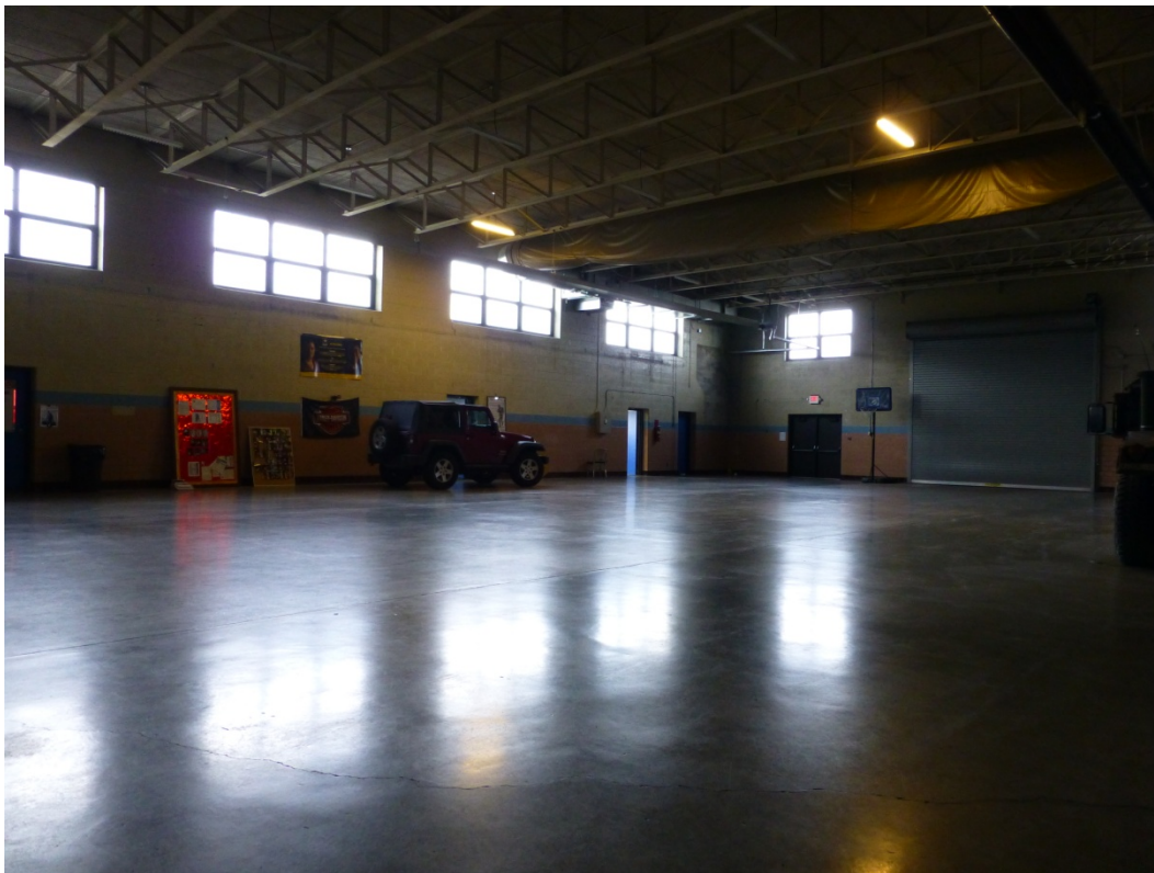
Figure 54. Interior view of the drill hall of Sandusky OHARNG Armory (ERDC-CERL, 2013).
