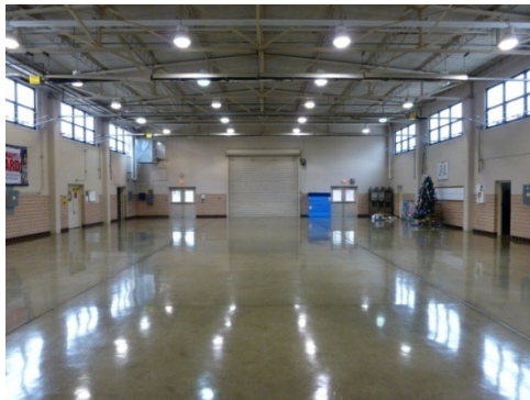
Interior view of the open double-height drill hall with concrete floor, combination of concrete-block and glazed sanitary tile walls, clerestory windows, and exposed truss roof system (ERDC-CERL, 2013).
