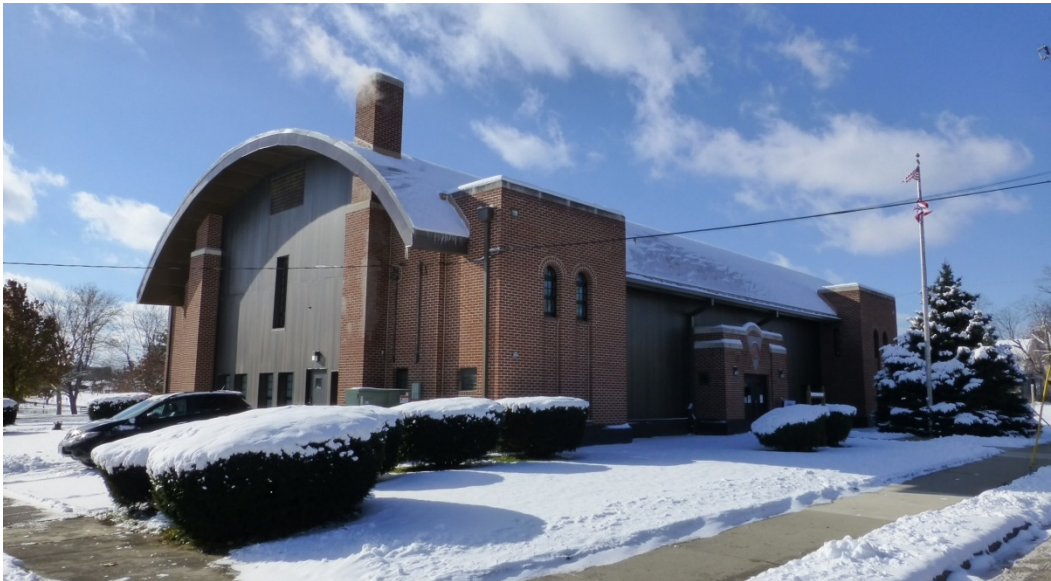
Figure 23. Northeast oblique of Xenia OHARNG Armory (ERDC-CERL, 2014).
