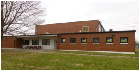
Tiffin OHARNG Armory (1954).
