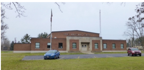
Norwalk OHARNG Armory (1961) – Type D.
