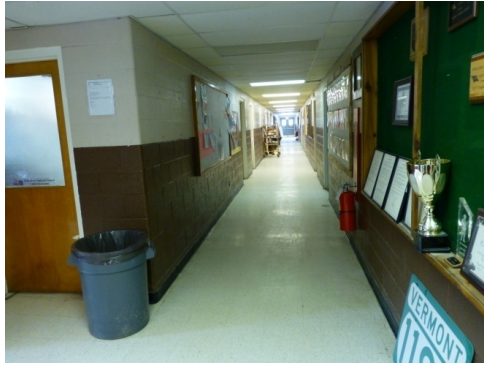
Central corridor with concrete-block walls (ERDC-CERL, 2014).
