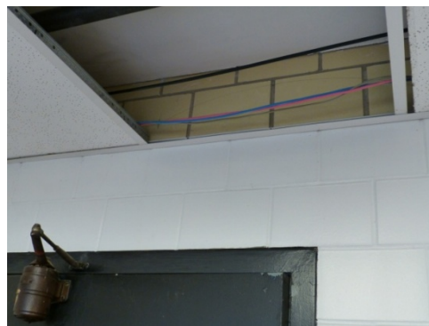
Looking up at the original unpainted glazed sanitary tile walls of the latrine (ERDC-CERL, 2014).
