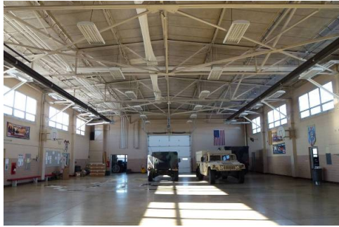
Interior view of the open double-height drill hall with concrete floor, combination of concrete-block and glazed sanitary tile walls, clerestory windows, and exposed truss roof system (ERDC-CERL, 2014).
