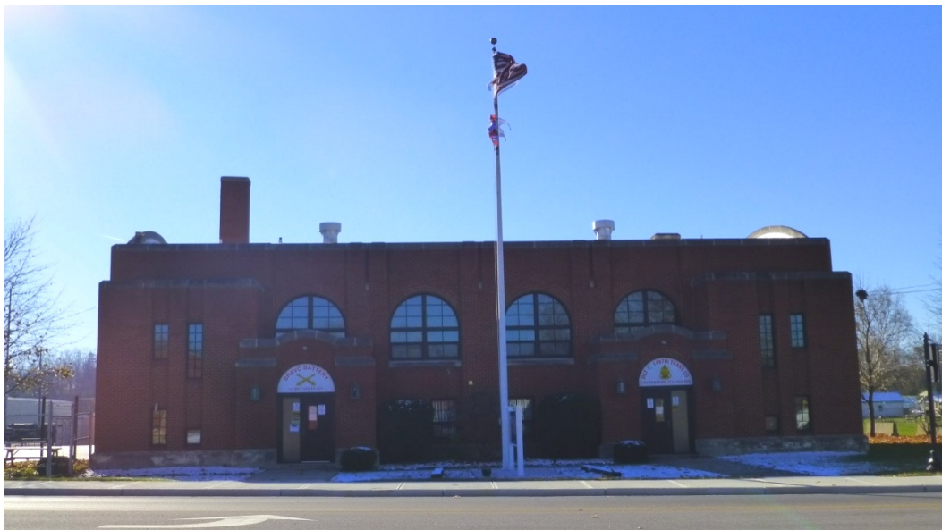
Figure 17. North (front) elevation of Piqua OHARNG Armory (ERDC-CERL, 2013).
