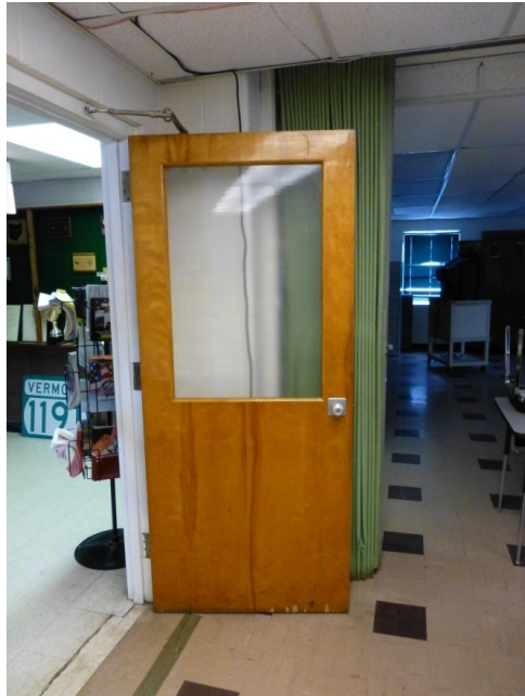
Original blonde wood and glass interior doors (ERDC-CERL, 2014).
