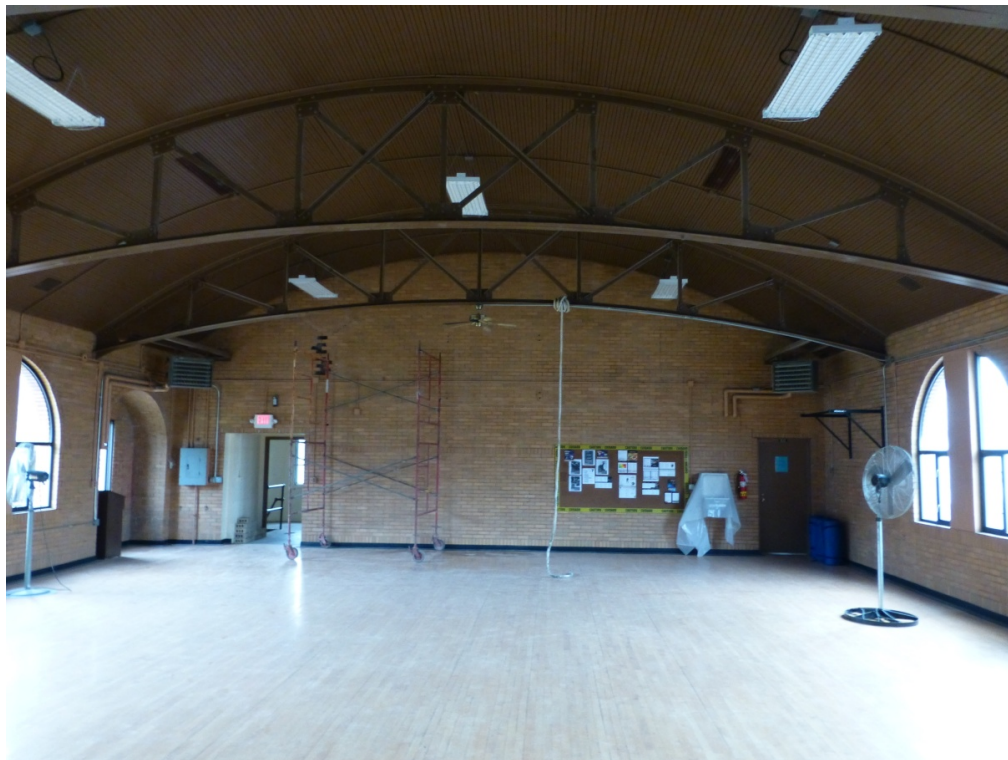
Figure 26. Interior view of the assembly hall at Akron-Hawkins OHARNG Armory (ERDC-CERL, 2013).
