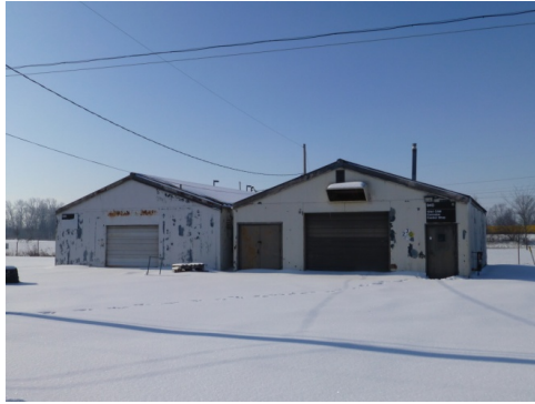
Rickenbacker Army Enclave, Building 939 on the left and Building 940 on the right (built in 1966 (Building 939) and 1965 (Building 940), acquired in 1996).
