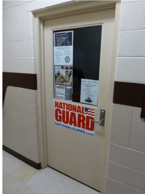
Typical metal and glass interior door (ERDC-CERL, 2013).
