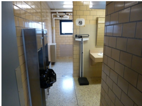
Original glazed sanitary tile walls in the women's latrine (ERDC-CERL, 2013).
