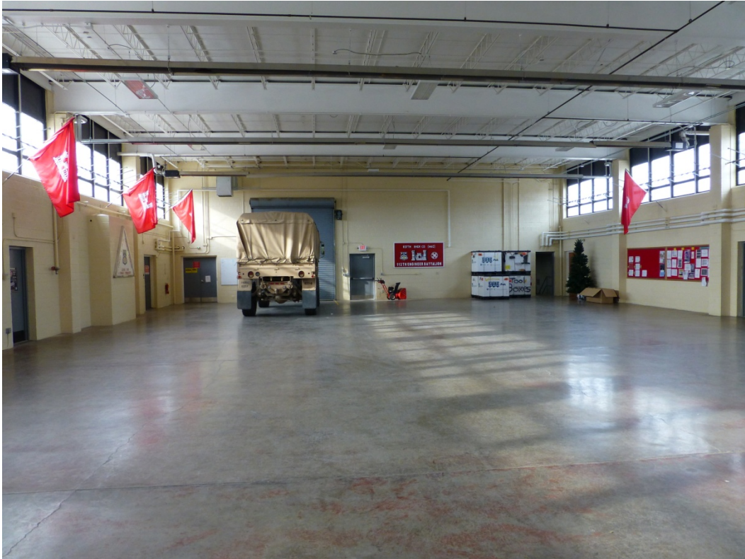
Figure 44. Interior view of the drill hall of Lorain OHARNG Armory (ERDC-CERL, 2013).
