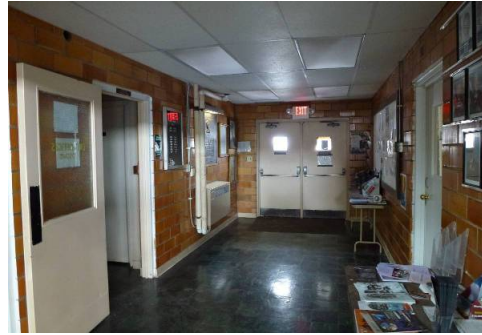
Glazed sanitary tile walls in the lobby (ERDC-CERL, 2014).
