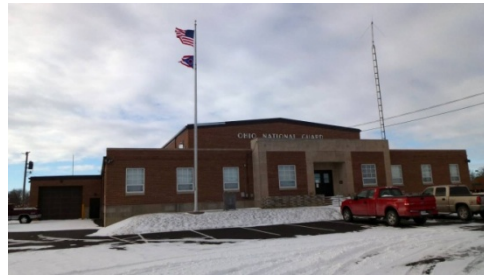
Greenville OHARNG Armory (1962).
