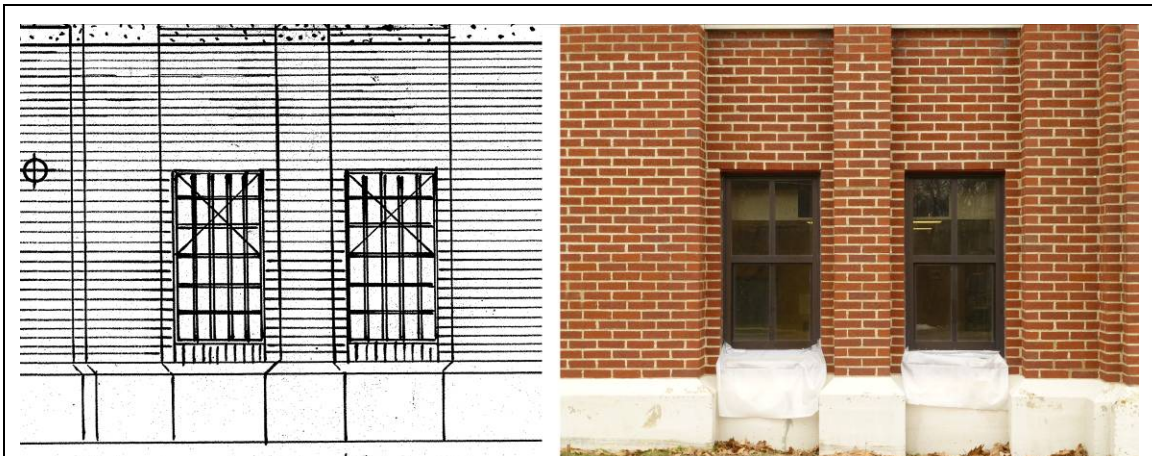
Rectangular window comparison: original on the left (1937 drawing), and the current photograph on the right (ERDC-CERL, 2013). Original multipane metal-sash awning window was replaced with anodized-bronze aluminum windows.
