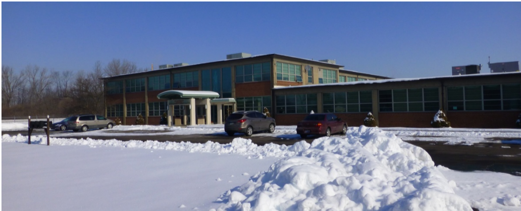
Figure 89. Southwest (front) elevation of Building 930 (ERDC-CERL, 2014).
