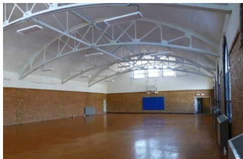
Interior view of the open assembly hall space on the second floor with wood floor, brick walls, barrel roof, and arched steel truss system (ERDC-CERL, 2013).
