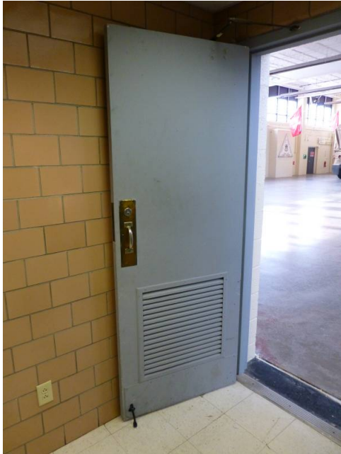
Original door into the men's latrine (ERDC-CERL, 2013).
