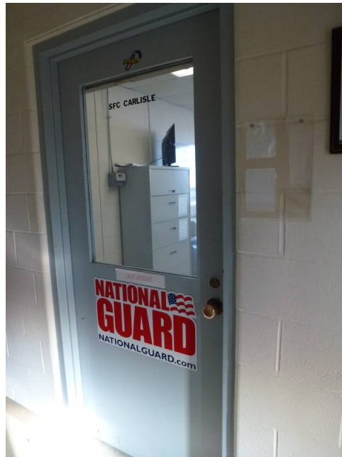
Typical metal and glass interior door (ERDC-CERL, 2014).
