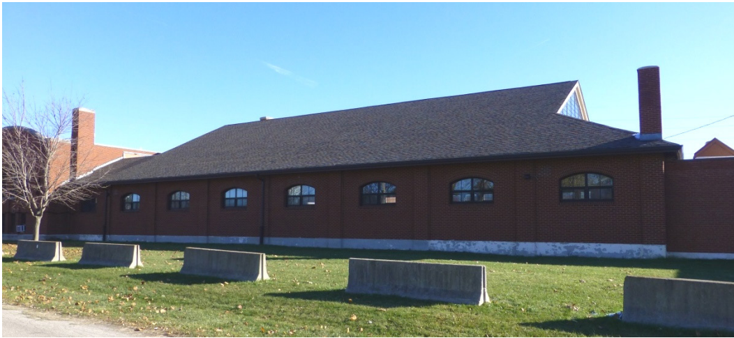
Figure 18. East elevation of the riding stadium at Piqua OHARNG Armory (ERDC-CERL, 2013).
