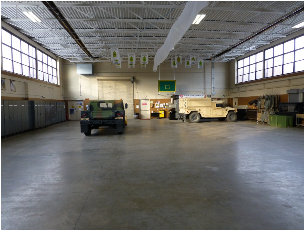
Figure 48. Interior view of the drill hall of Chagrin Falls OHARNG Armory (ERDC-CERL, 2013).
