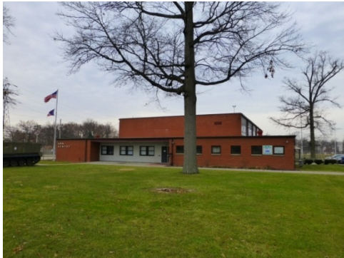
Brick exterior walls, one-story administration wings with central high-bay drill hall space, flat roofs (ERDC-CERL, 2013).
