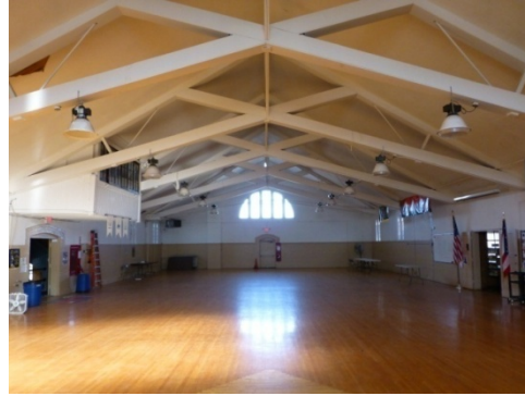
St. Marys OHARNG Armory, open interior of assembly hall space with exposed wood scissor trusses and wood plank floor (ERDC-CERL, 2013).
