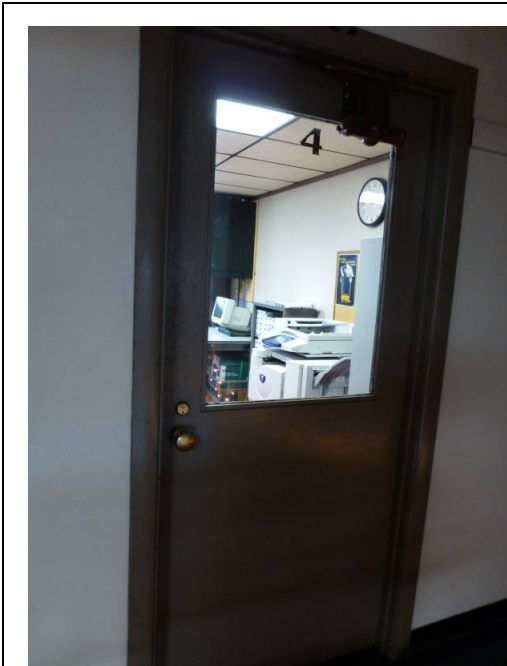
Typical metal and glass interior door (ERDC-CERL, 2013).
