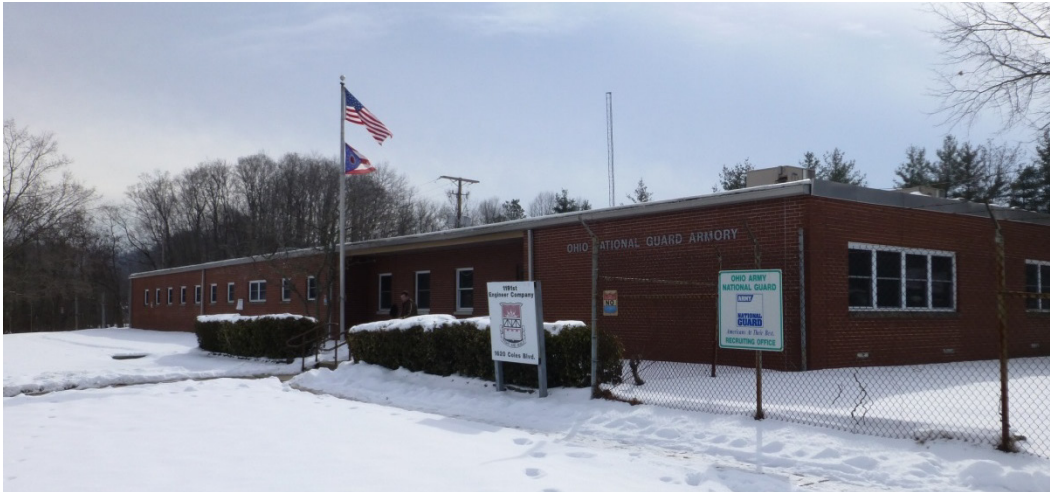
Figure 80. North (front) elevation of the Portsmouth OHARNG Armory (ERDC-CERL, 2014).
