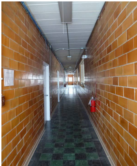
Second floor corridor with glazed sanitary tile walls (ERDC-CERL, 2014).
