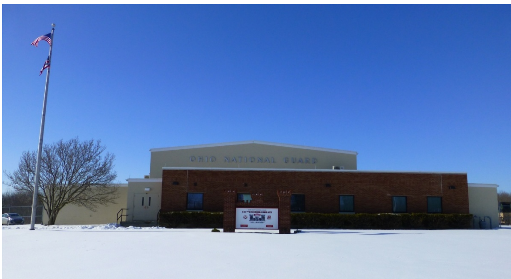
Figure 71. East (front) elevation of Tarlton OHARNG Armory (ERDC-CERL, 2014).
