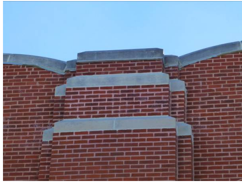
Stone coping and horizontality of details on front elevation (ERDC-CERL, 2013).
