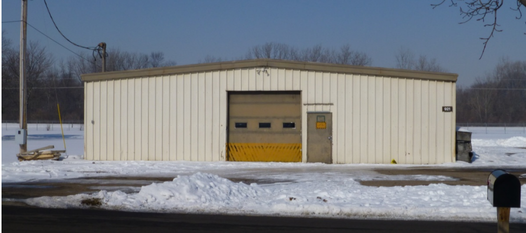
Figure 87. Southeast (front) elevation of Building 921 (ERDC-CERL, 2014).
