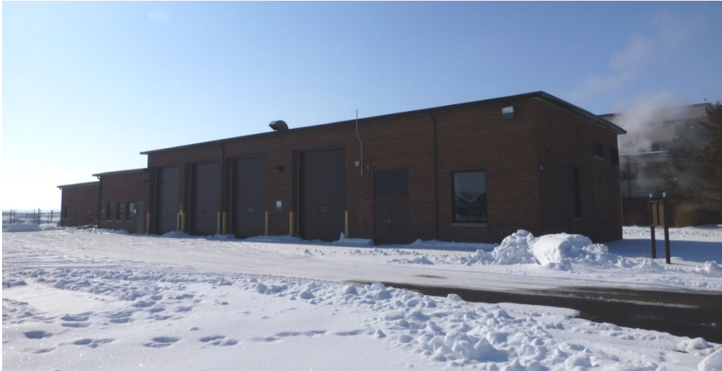
Figure 94. Northeast (front) elevation of Building 932 (ERDC-CERL, 2014).
