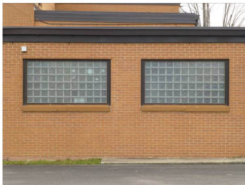
Original paired window openings with replacement windows (ERDC-CERL, 2014).
