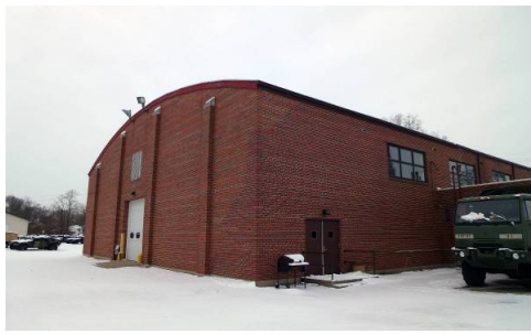
Barrel roof over the drill hall (ERDC-CERL, 2014).
