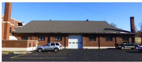
Gable-on-hip roof of riding stadium (ERDC-CERL, 2013).
