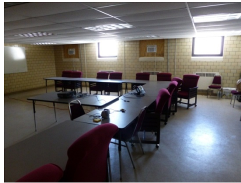
Interior view of the modified space of the original locker room, glazed sanitary tile walls intact (ERDC-CERL, 2014).
