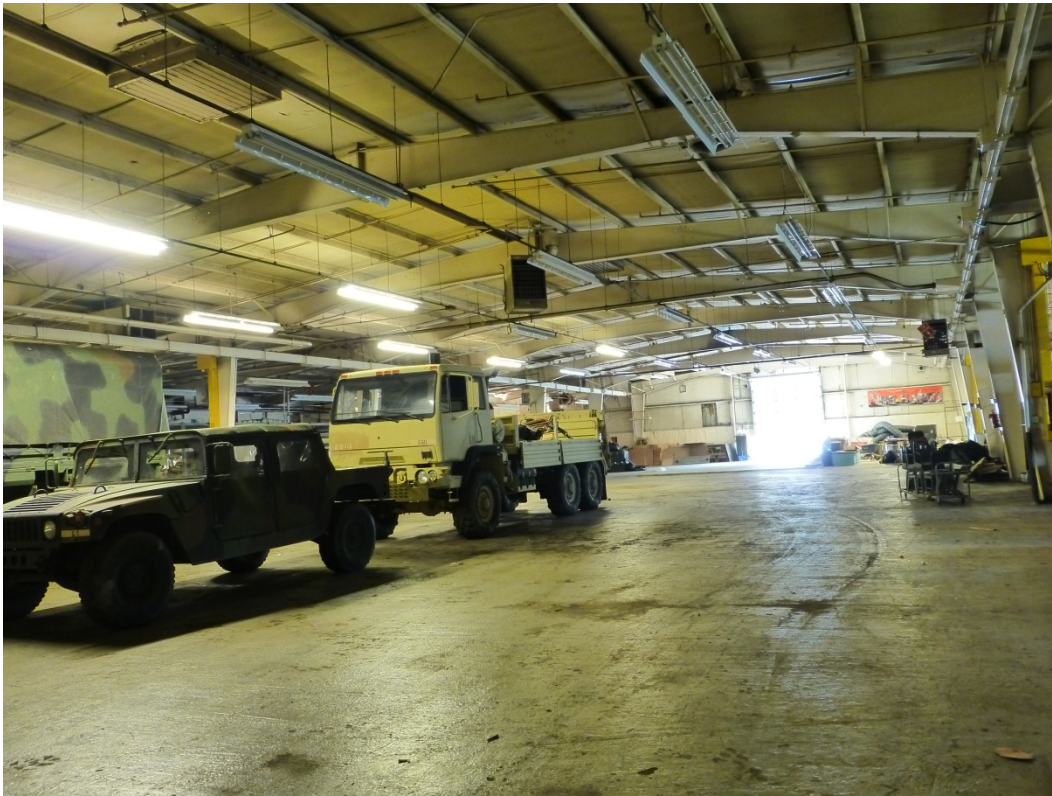
Figure 79. Interior view of the open high-bay area of the Medina OHARNG Armory (ERDC-CERL, 2013).
