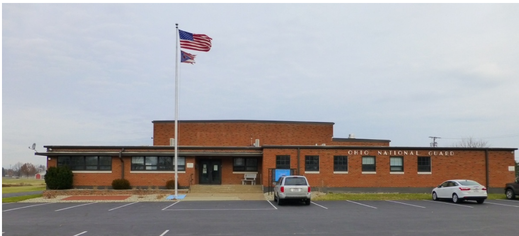
Figure 53. South (front) elevation of the Sandusky OHARNG Armory (ERDC-CERL, 2013).
