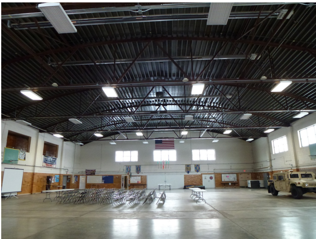
Figure 38. Interior view of the drill hall at Middletown-Kessler OHARNG Armory (ERDC-CERL, 2014).
