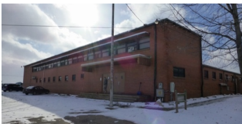
Springfield OHARNG Armory (1956).
