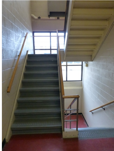
Metal switchback staircase with original wood and metal handrails (ERDC-CERL, 2013).
