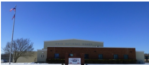
Tarlton OHARNG Armory (1968) – Type D.
