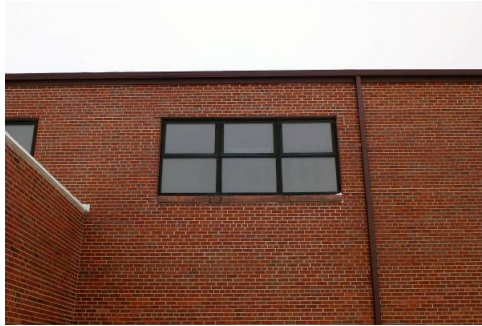
Large clerestory windows (replacement) (ERDC-CERL, 2014).
