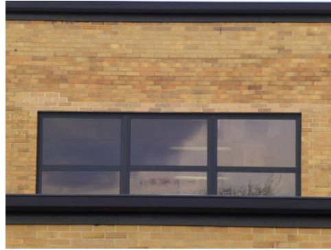
Original clerestory window opening with replacement one-over-one anodized-bronze aluminum windows (ERDC-CERL, 2013).
