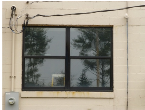
Original paired window openings with replacement one-over-one anodized-bronze aluminum windows (ERDC-CERL, 2013).
