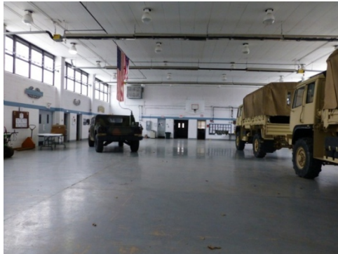
Interior view of the open drill hall, concrete floor, clerestory windows, concrete-block walls, and steel I-beam roofing system (ERDC-CERL, 2013).
