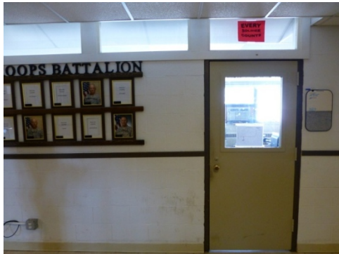
Typical metal and glass interior door (ERDC-CERL, 2014).
