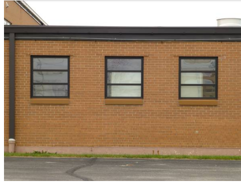
Original single window openings with replacement three-pane anodized-bronze aluminum windows (ERDC-CERL, 2014).
