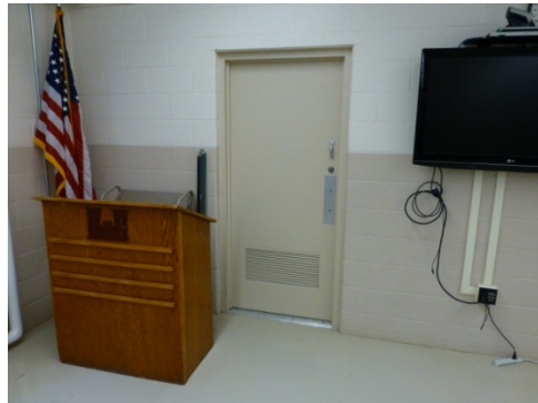
Typical metal door with louvered vent (ERDC-CERL, 2013).
