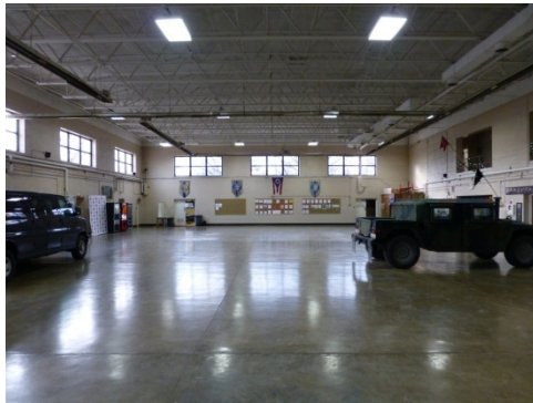
Interior view of the open drill hall space with concrete floor, clerestory windows, exposed truss system, and glazed sanitary tile walls (ERDC-CERL, 2013).
