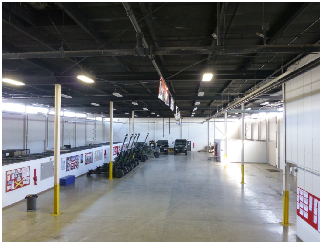
Figure 77. Interior view of the open high-bay of the Marion OHARNG Armory (ERDC-CERL, 2014).
