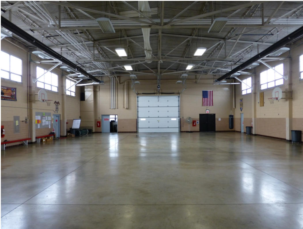
Figure 70. Interior view of the drill hall of Greenville OHARNG Armory (ERDC-CERL, 2014).
