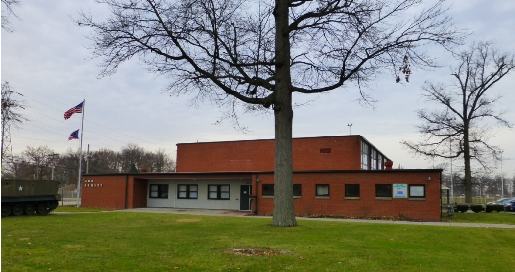
Figure 43. East elevation of Lorain OHARNG Armory (ERDC-CERL, 2013).
