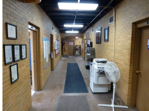
Central corridor with brick walls and concrete floor (ERDC-CERL, 2013).
