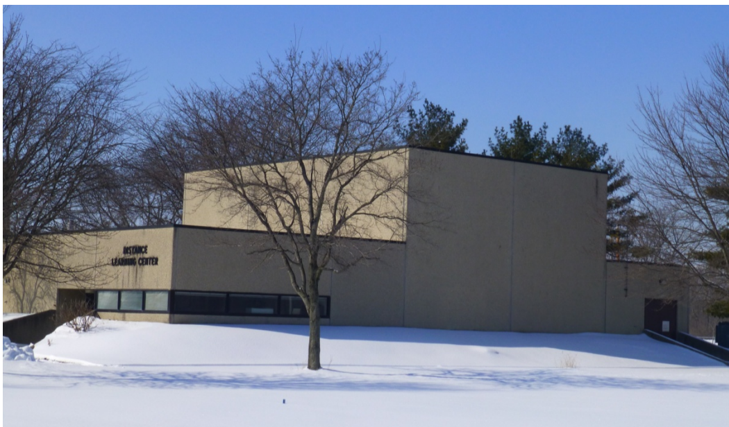
Figure 100. East oblique of Building 944 (ERDC-CERL, 2014).
