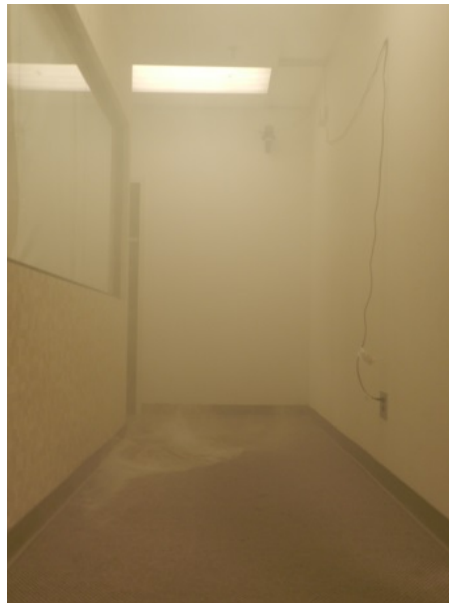
Figure 31: Example of smoke-filled hallway after smoke detector is triggered.
