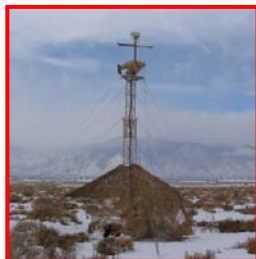
Remote Sensor Station
