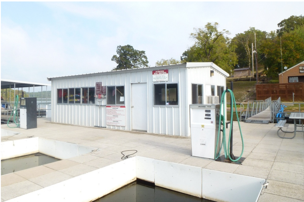
Figure 49. Southwest oblique of Building 537 (ERDC-CERL, 2015).
