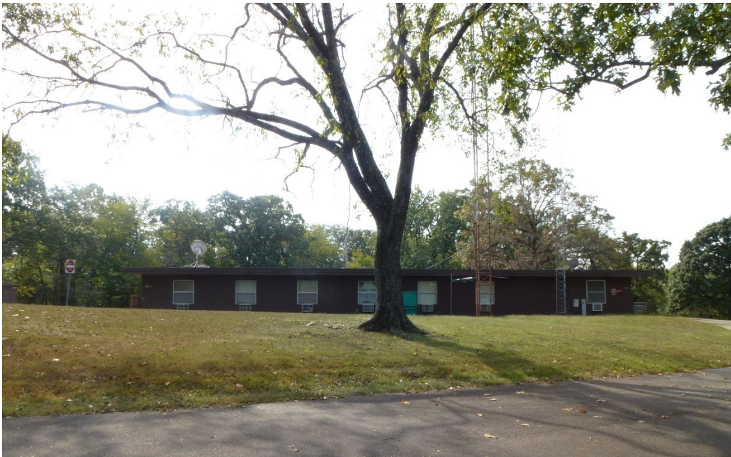
Figure 68. North elevation of Building 560 (ERDC-CERL, 2015).
