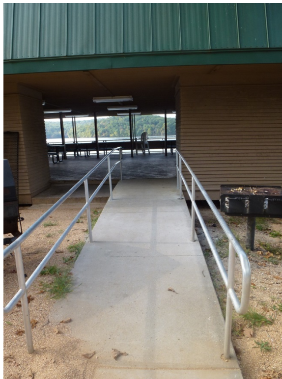
Figure 54. Newer concrete ramp on the northeast side of Building 549 (ERDC-CERL, 2015).
