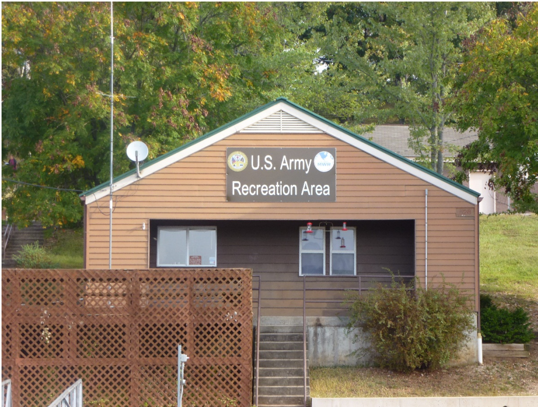
Figure 44. South elevation of Building 528 (ERDC-CERL, 2015).
