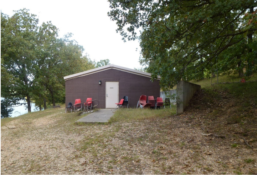
Figure 14. South elevation of Building 144 (ERDC-CERL, 2015).
