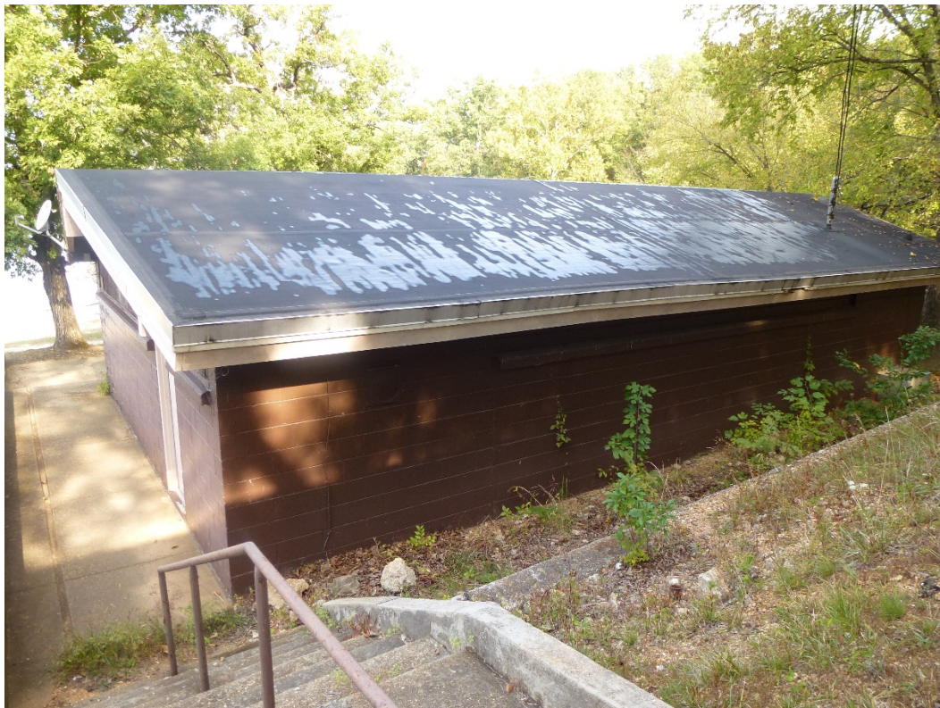
Figure 62. North elevation of Building 550 (ERDC-CERL, 2015).
