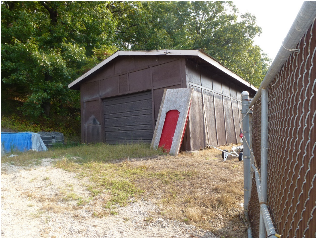
Figure 36. West elevation of Building 506 (ERDC-CERL, 2015).
