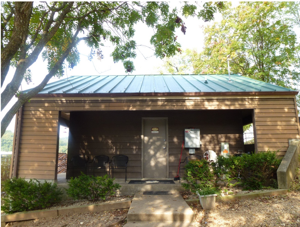
Figure 45. East elevation of Building 528 (ERDC-CERL, 2015).
