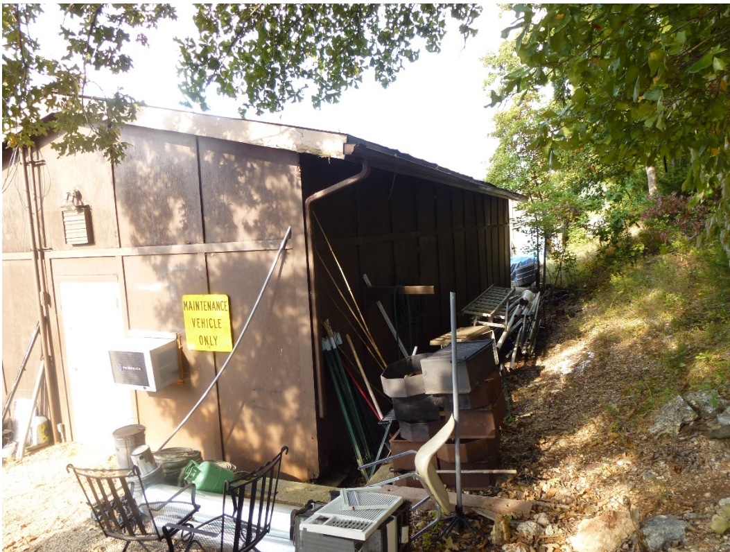
Figure 39. North elevation of Building 506 (ERDC-CERL, 2015).
