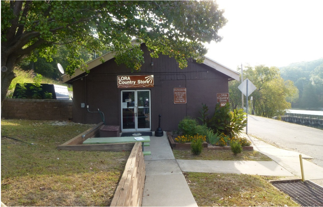
Figure 27. West (front) elevation of Building 500 (ERDC-CERL, 2015).
