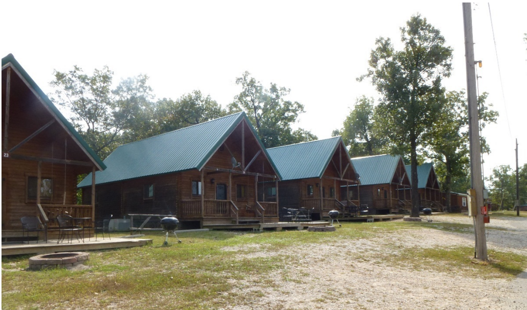
Figure 83. Examples of 3-bedroom log cabins with loft off Fleet Lane (ERDC-CERL, 2015).
