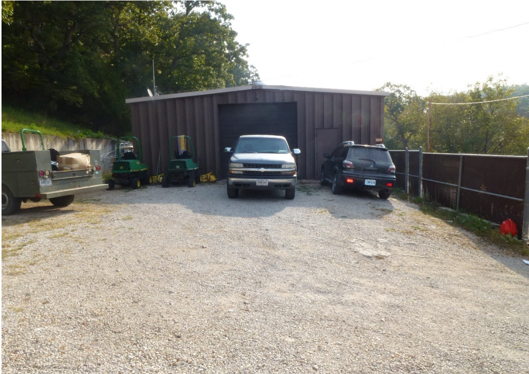
Figure 31. West elevation of Building 505 (ERDC-CERL, 2015).
