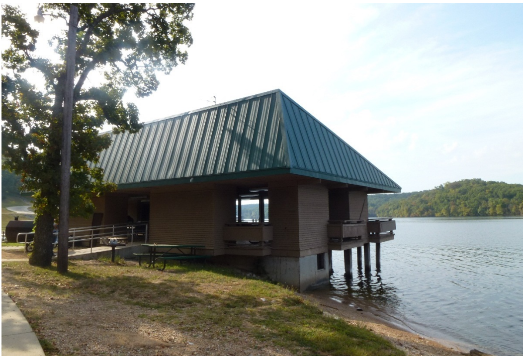
Figure 52. North oblique of Building 549 (ERDC-CERL, 2015).
