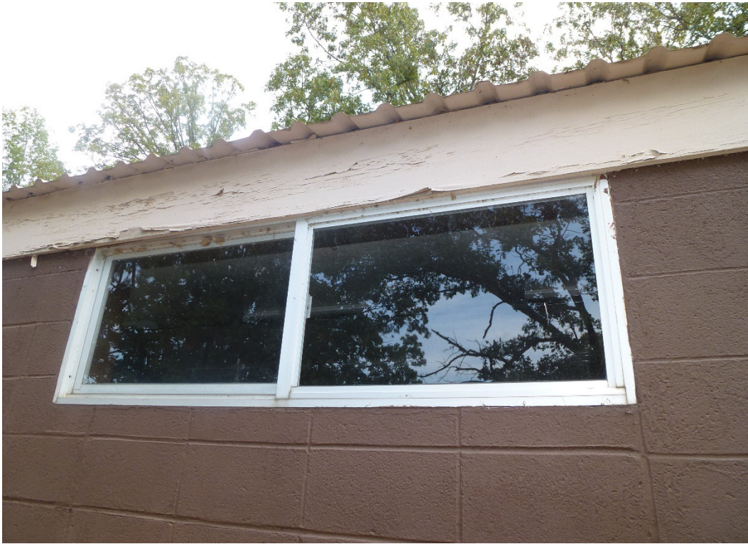
Figure 20. Close-up of metal-sash slider window, wood fascia, and metal roof decking on Building 146 (ERDC-CERL, 2015).
