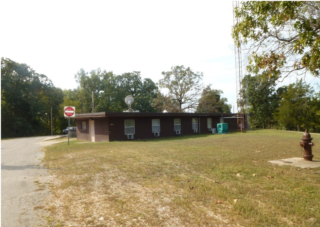
Figure 69. Northeast oblique of Building 560 (ERDC-CERL, 2015).
