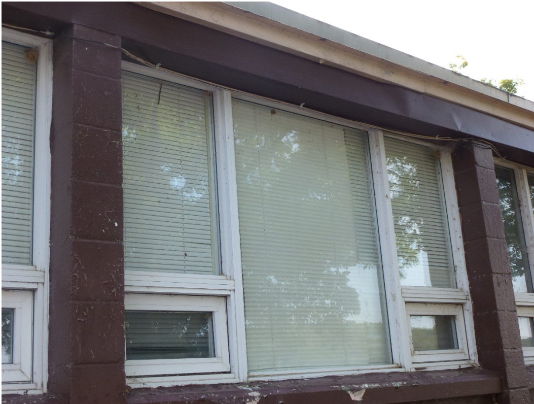
Figure 60. Close-up of a replacement vinyl window on the south elevation of Building 550 (ERDC-CERL, 2015).
