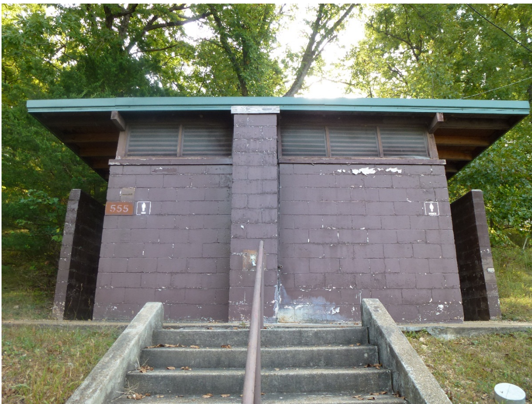
Figure 64. South elevation of Building 555 (ERDC-CERL, 2015).
