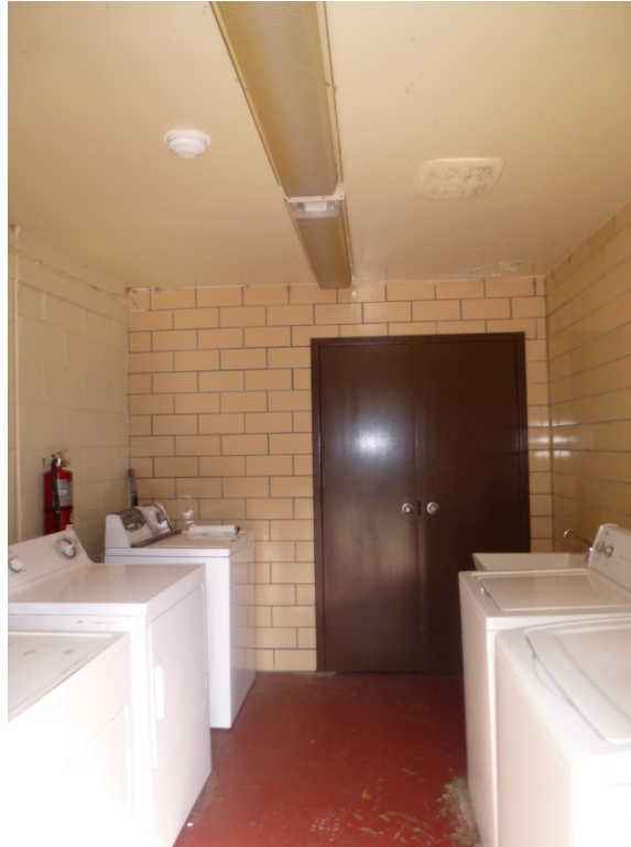
Figure 77. Interior view of the laundry facility of Building 560 (ERDC-CERL, 2015).
