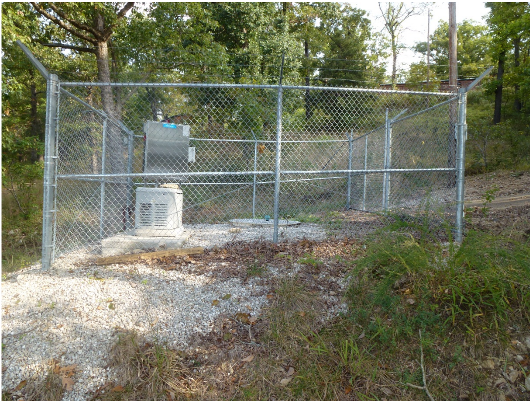
Figure 98. View of Building 610 (ERDC-CERL, 2015).
