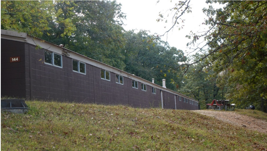
Figure 12. West elevation of Building 144 (ERDC-CERL, 2015).
