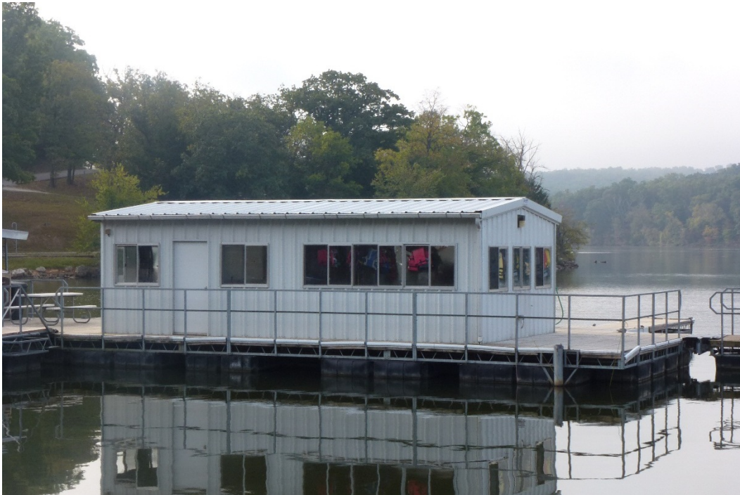
Figure 48. Northeast oblique of Building 537 (ERDC-CERL, 2015).
