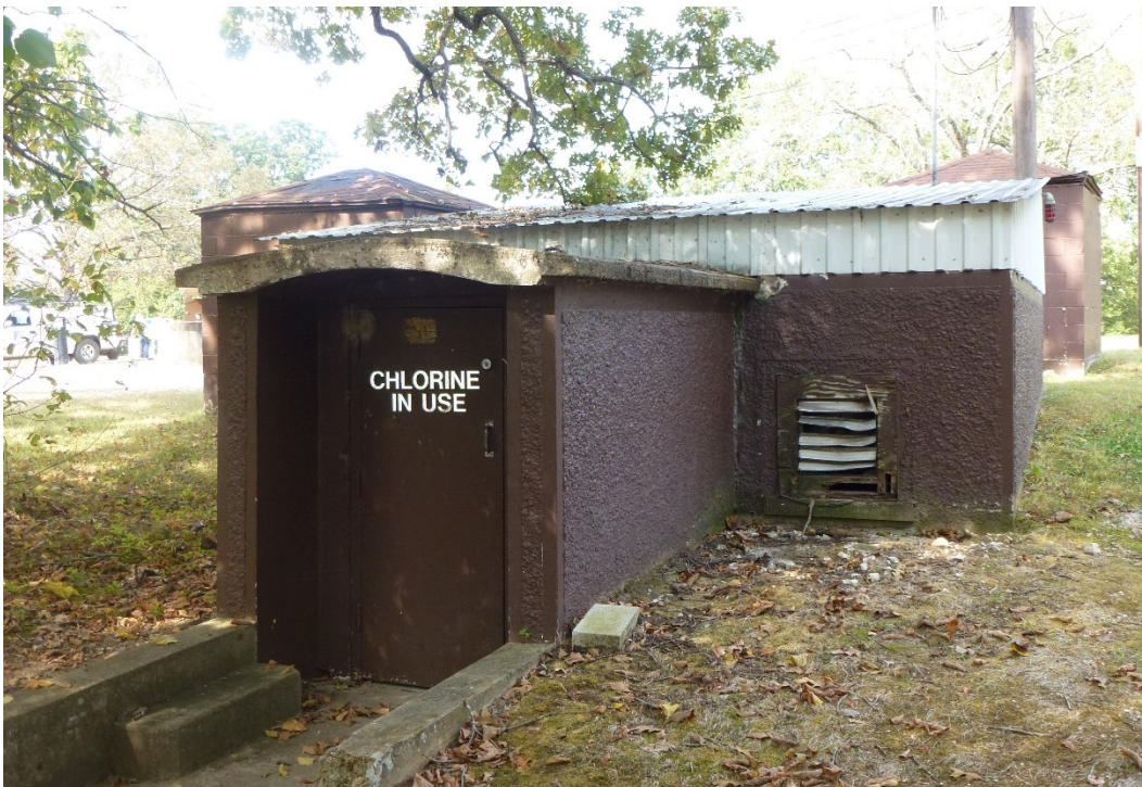
Figure 94. Southeast elevation, showing the concrete appendage of Building 561 (ERDC-CERL, 2015).
