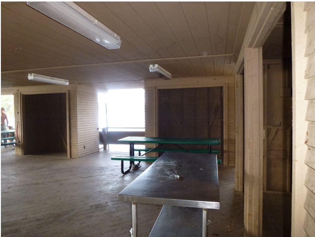
Figure 56. View of partial wall enclosures for the storage areas of Building 549 (ERDC-CERL, 2015).
