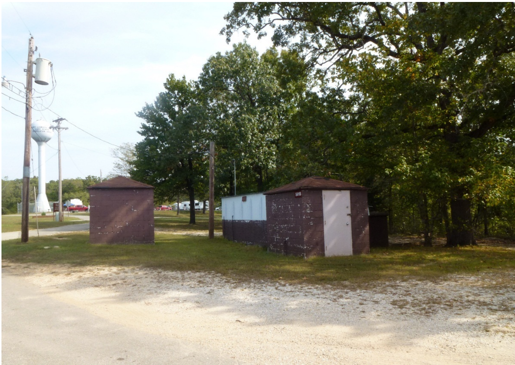
Figure 97. Southwest oblique of Building 561B [right] and south elevation of Building 561A [left] (ERDC-CERL, 2015).
