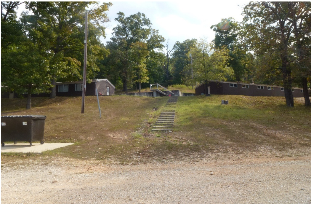
Figure 11. Looking east from the lower gravel road upward to Building 146 [left] and Building 144 [right] (ERDC-CERL, 2015).
