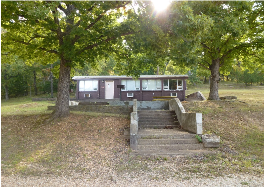
Figure 58. The concrete steps, retaining walls, and porch leading up to the south elevation of Building 550 (ERDC-CERL, 2015).
