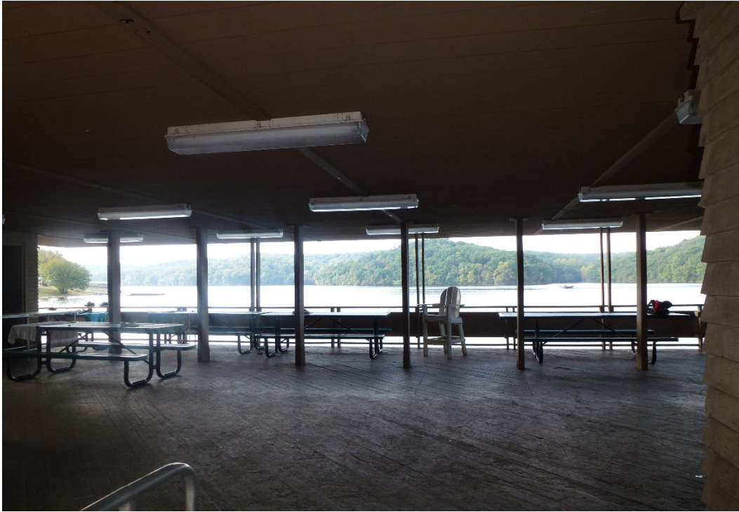
Figure 55. Interior view of Building 549 (ERDC-CERL, 2015).
