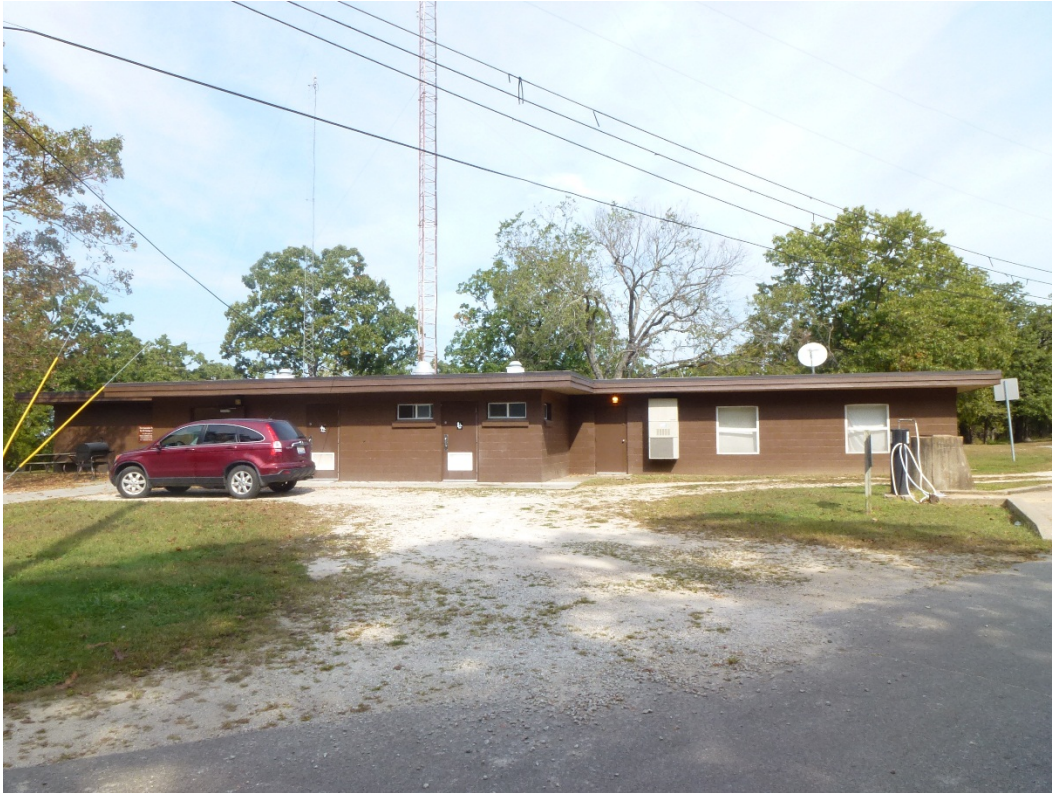
Figure 71. South elevation of Building 560 (ERDC-CERL, 2015).
