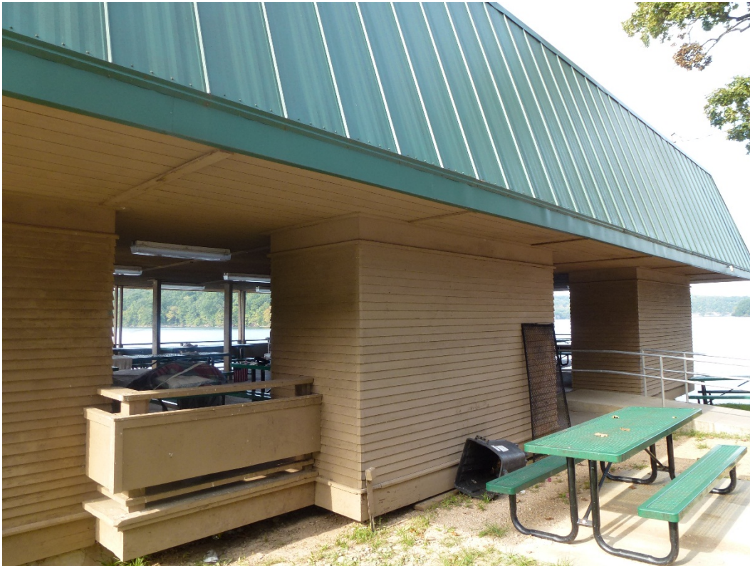
Figure 53. Northeast side of Building 549 (ERDC-CERL, 2015).
