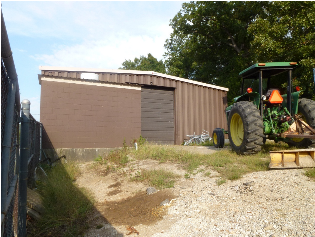
Figure 34. East elevation of Building 505 (ERDC-CERL, 2015).
