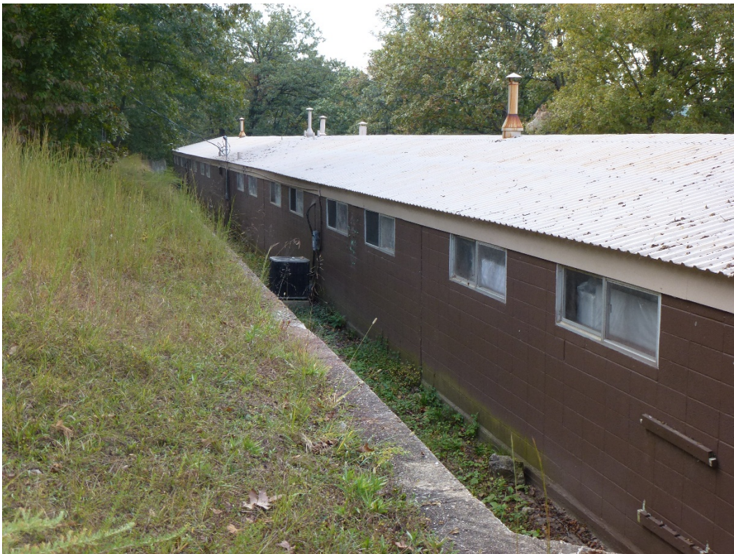
Figure 13. East elevation of Building 144 (ERDC-CERL, 2015).
