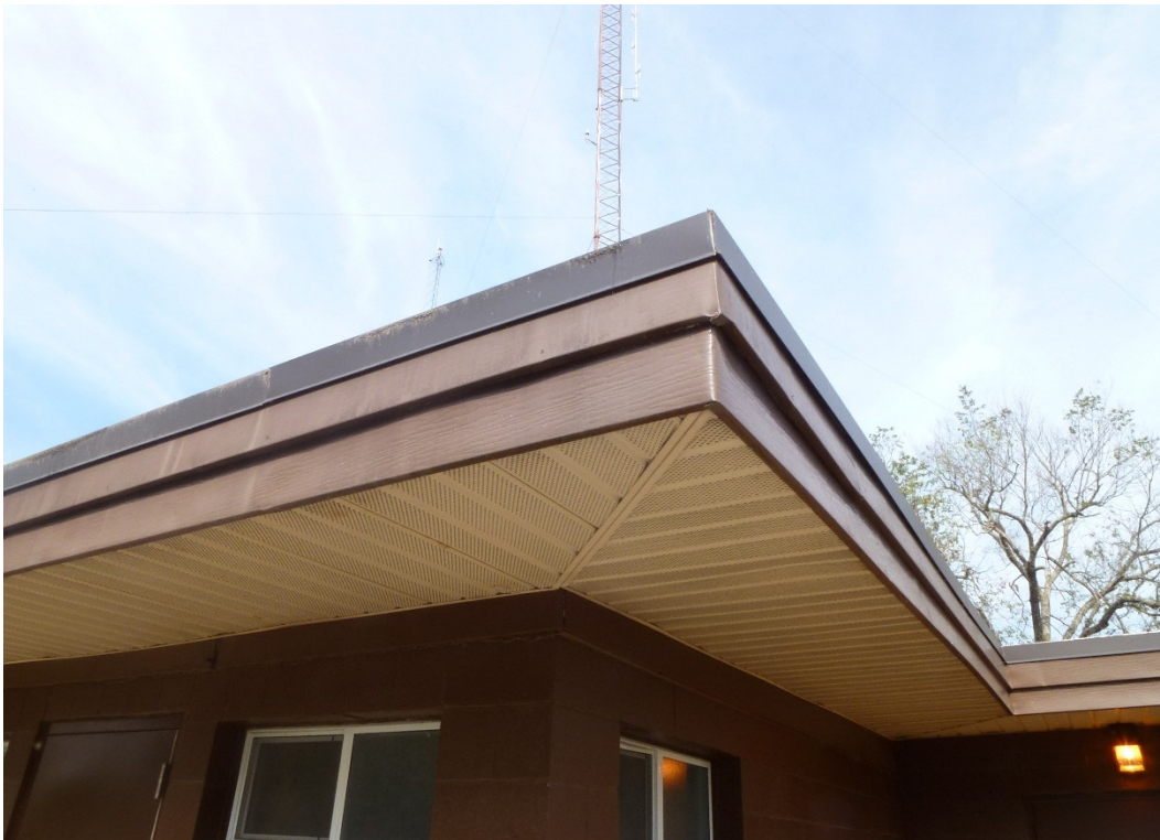
Figure 72. Close-up of the modified overhanging eave of Building 560 (ERDC-CERL, 2015).
