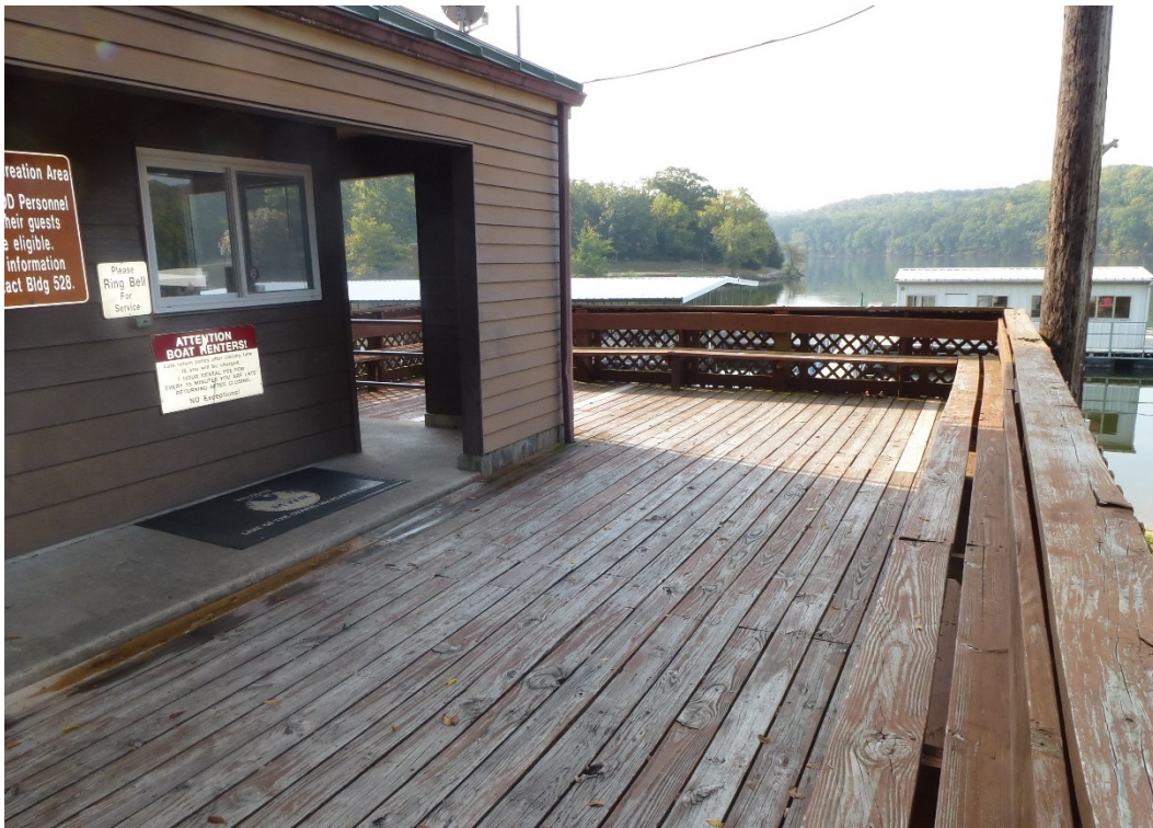
Figure 42. Wood deck addition surrounding the Building 528 on the east, south, and west sides (ERDC-CERL, 2015).
