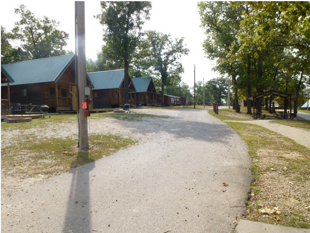
Figure 109. Looking south on Fleet Lane, with a row of three-bedroom log cabins on the left (ERDC-CERL, 2015).
