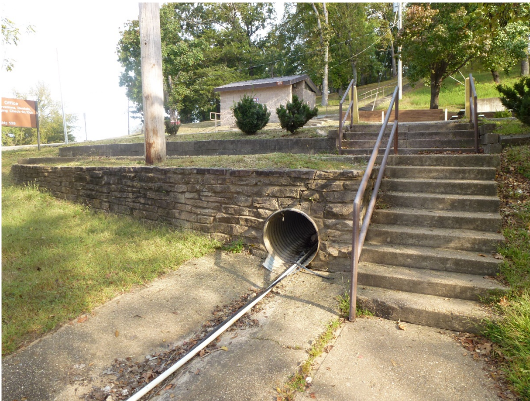
Figure 120. Stonework retaining wall constructed near Building 528 (ERDC-CERL, 2015).
