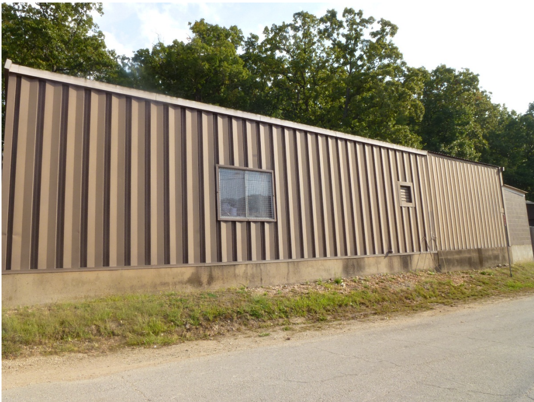
Figure 32. South elevation of Building 505 (ERDC-CERL, 2015).
