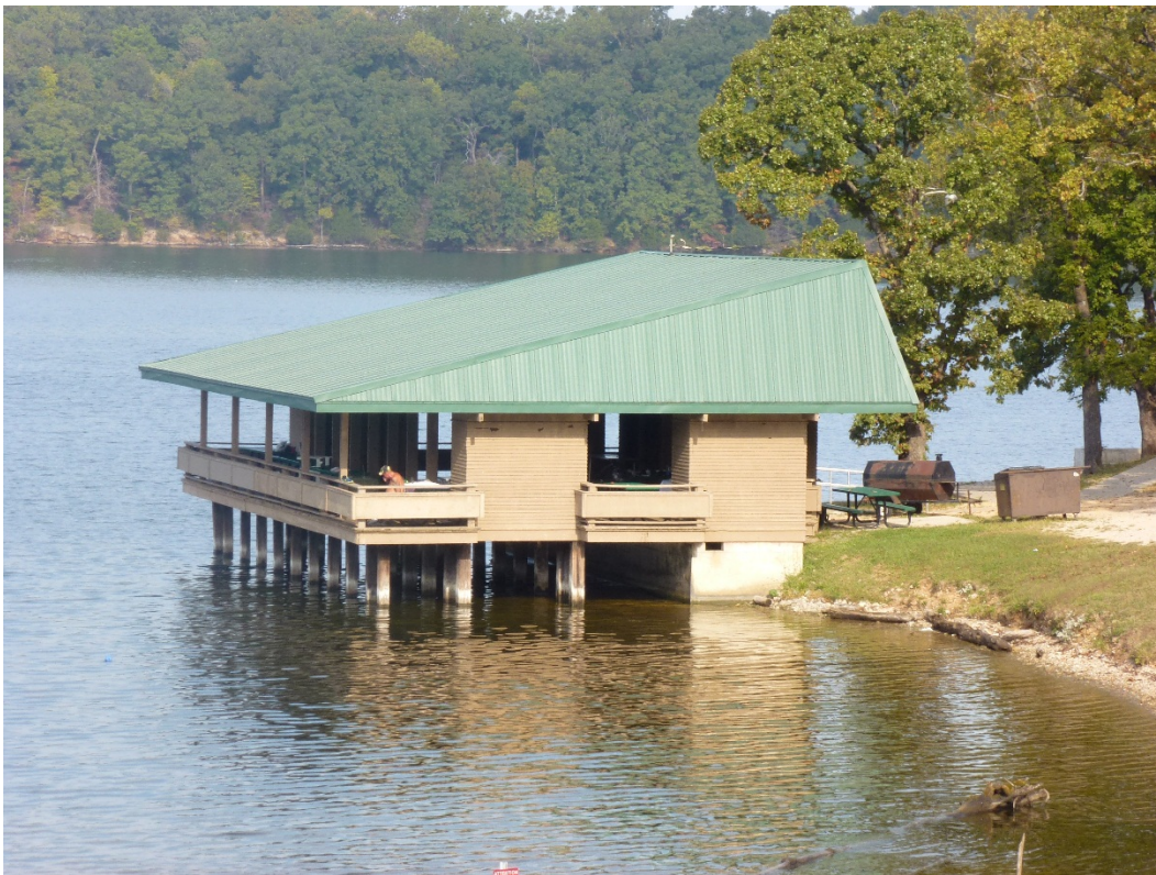
Figure 51. Looking at the southeast and southwest sides of Building 549, with the poured concrete foundation visible at the shoreline (ERDC-CERL, 2015).
