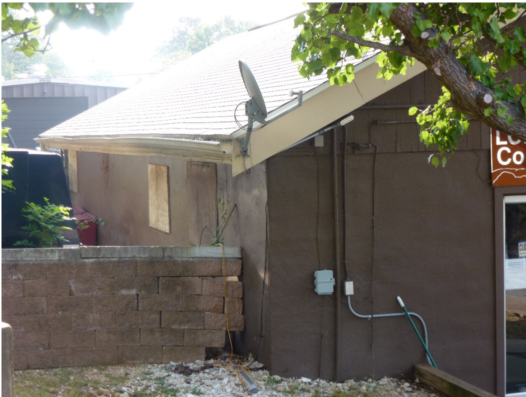
Figure 30. Northwest oblique of Building 500 (ERDC-CERL, 2015).
