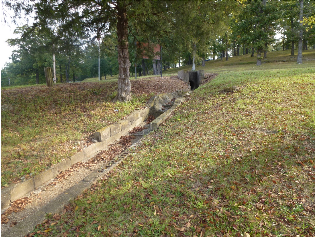
Figure 122. Concrete ditch located near Building 528 (ERDC-CERL, 2015).
