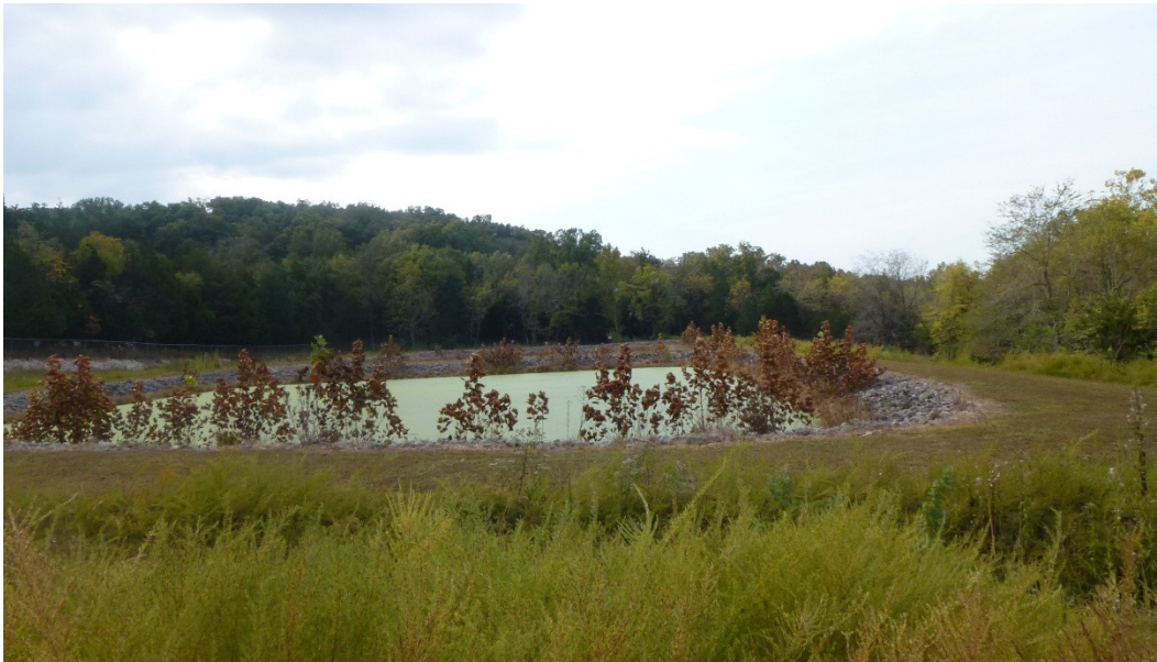
Figure 101. Looking at one of the two waste lagoons located at the south end of LORA (ERDC-CERL, 2015).
