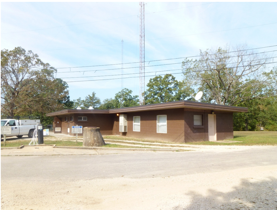
Figure 70. Southeast oblique of Building 560 (ERDC-CERL, 2015).
