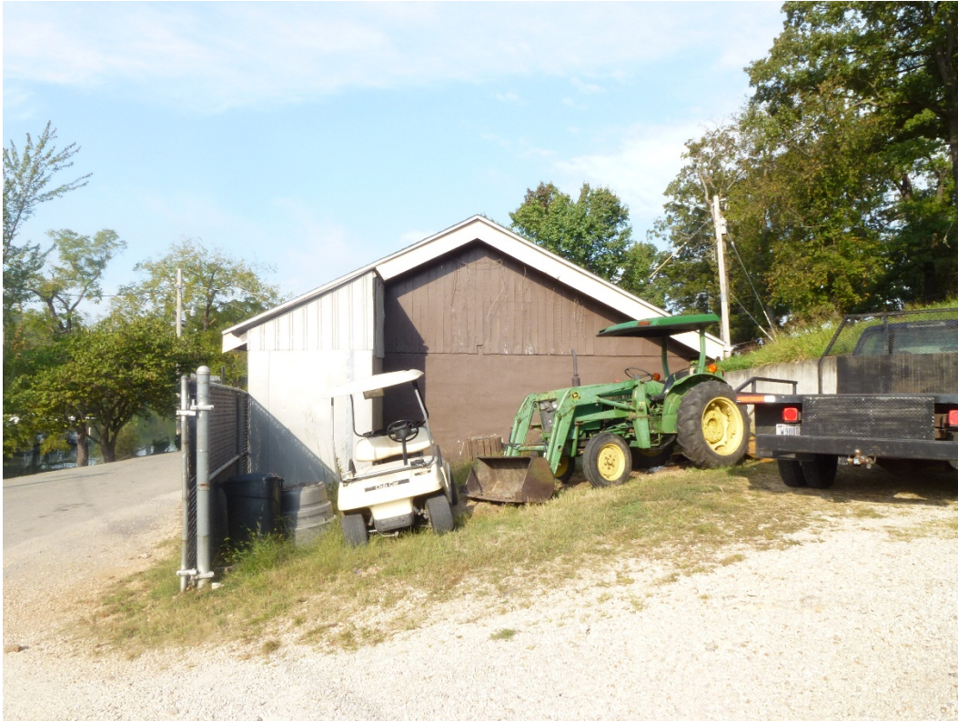
Figure 29. East elevation of Building 500 (ERDC-CERL, 2015).
