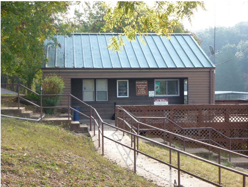
Figure 47. West elevation of Building 528 (ERDC-CERL, 2015).
