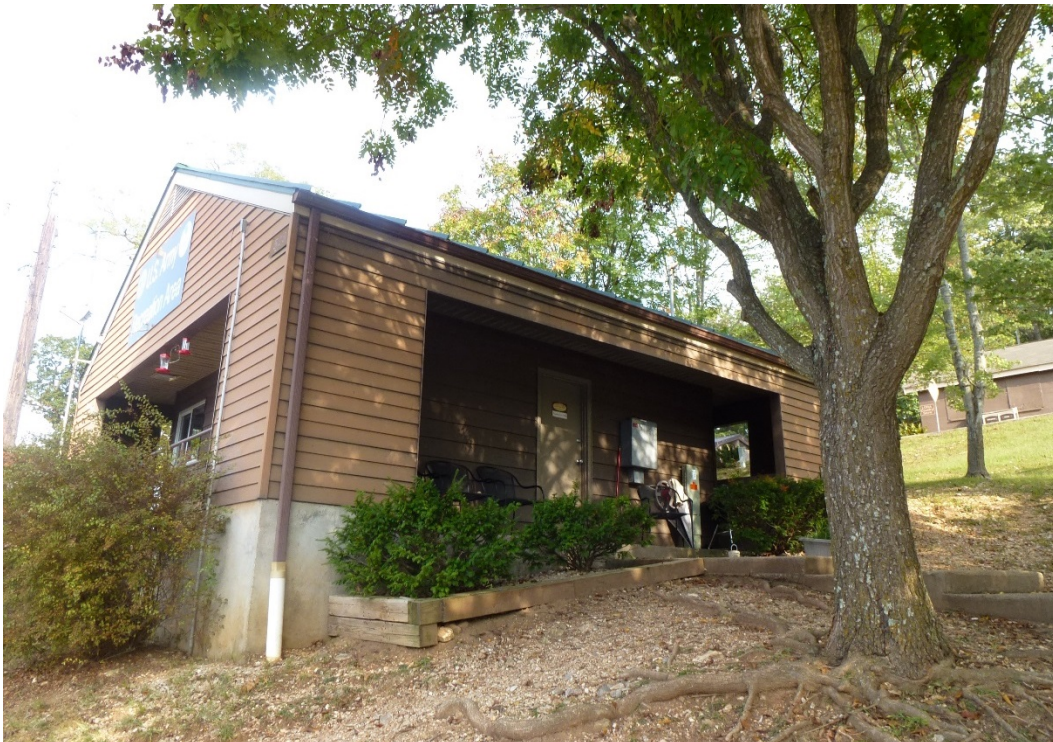
Figure 43. Gable roof that extends out to protect the incised concrete walkway of Building 528 (ERDC-CERL, 2015).
