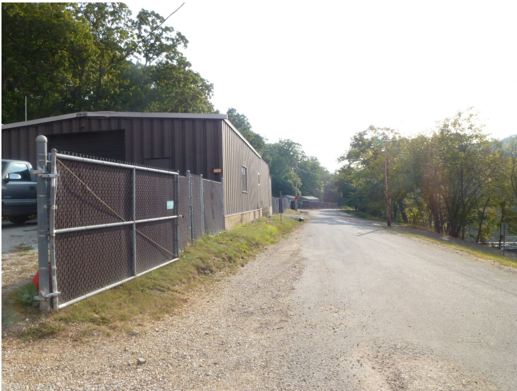
Figure 107. Looking southeast down Olney Circle with Building 505 on the left (ERDC-CERL, 2015).
