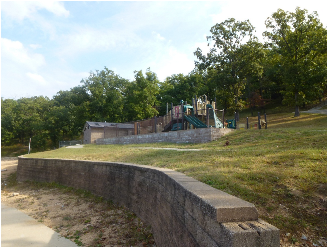
Figure 121. Newer concrete-block retaining wall near the swimming area (ERDC-CERL, 2015).
