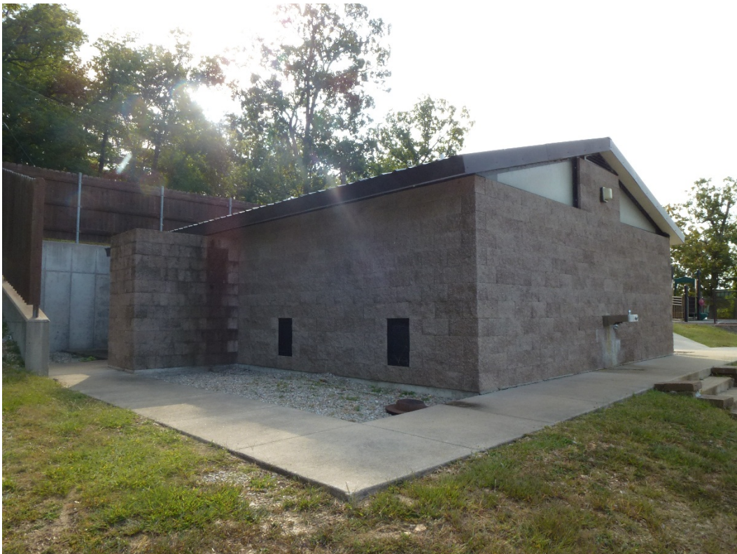
Figure 133. Newer bath house facility located near the boat launch (ERDC-CERL, 2015).
