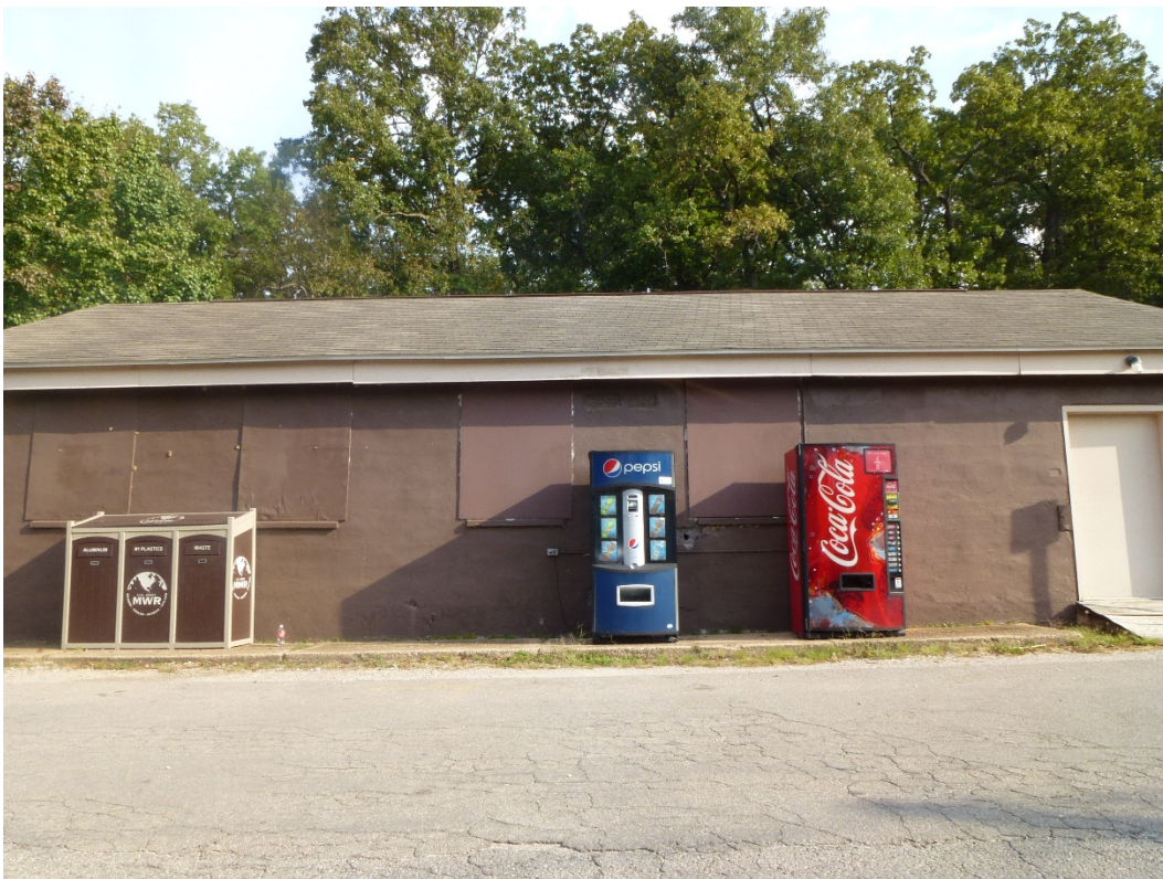
Figure 28. South elevation of Building 500 (ERDC-CERL, 2015).
