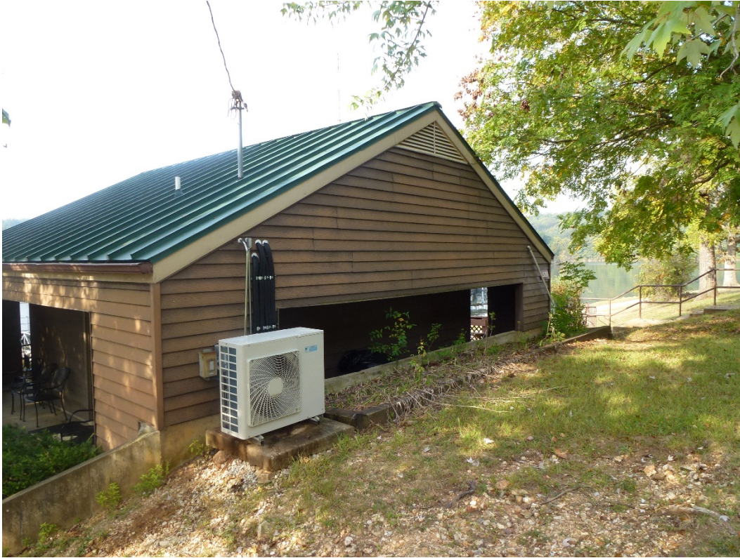
Figure 46. North elevation of Building 528 (ERDC-CERL, 2015).
