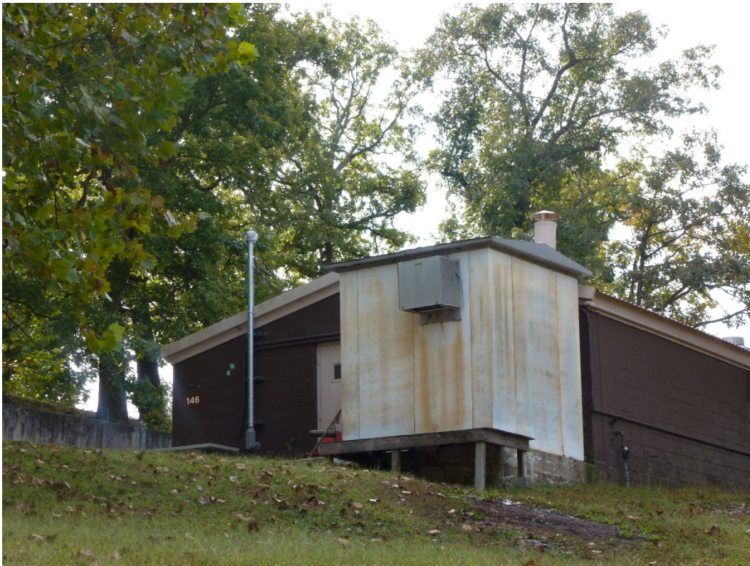
Figure 21. North elevation of Building 146 (ERDC-CERL, 2015).
