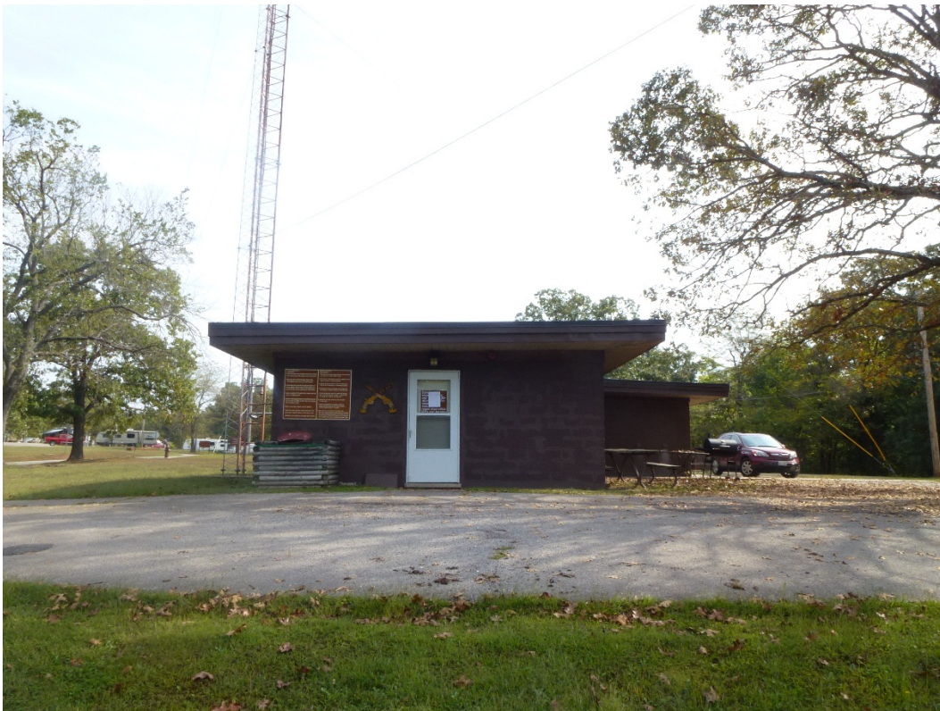
Figure 76. West elevation of Building 560 (ERDC-CERL, 2015).
