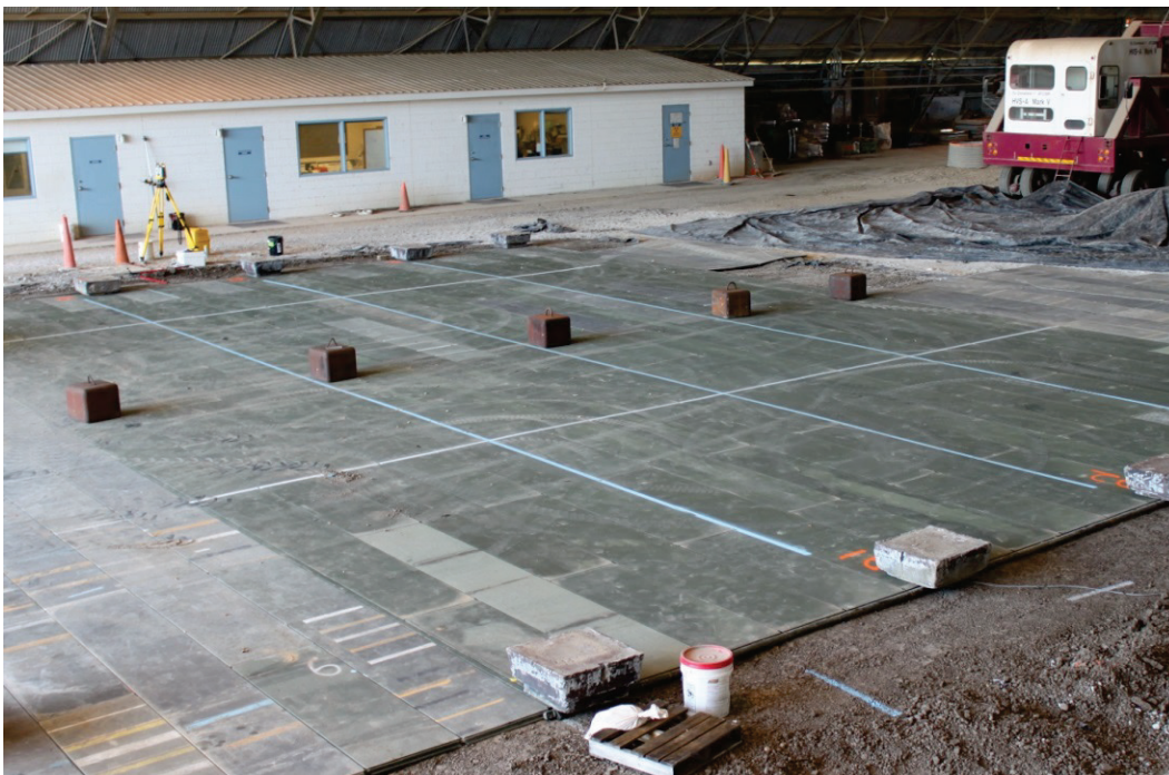
Figure 27. Test section surfaced with AM2.
