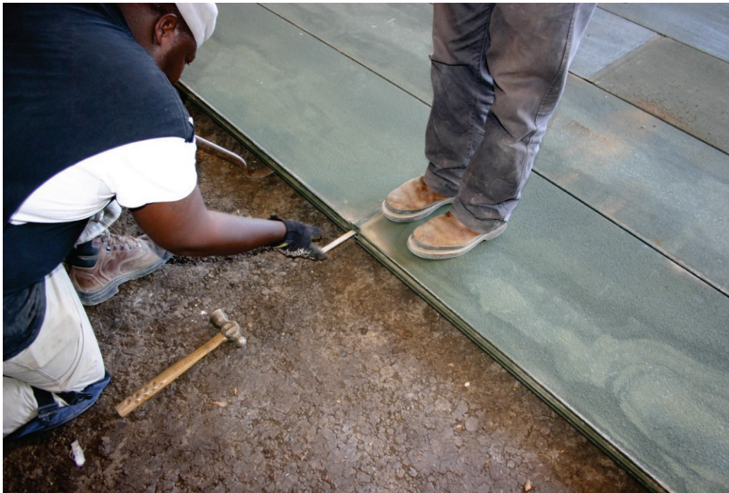
Figure 29. Insertion of AM2 locking bar.
