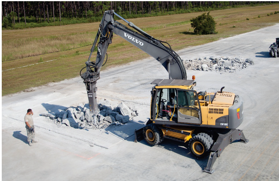
Figure 23. Large crater repair area.
