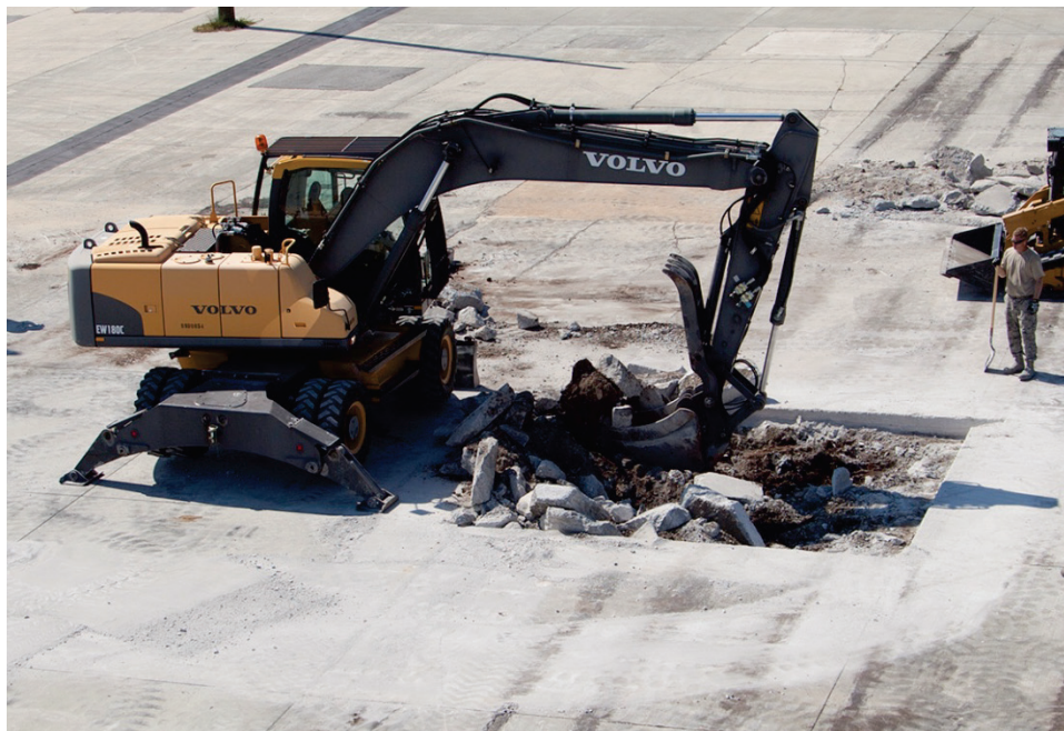
Figure 14. Removing debris using bucket attachment.
