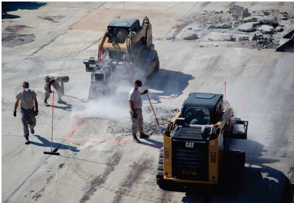
Figure 12. Sawing crater repair area.
