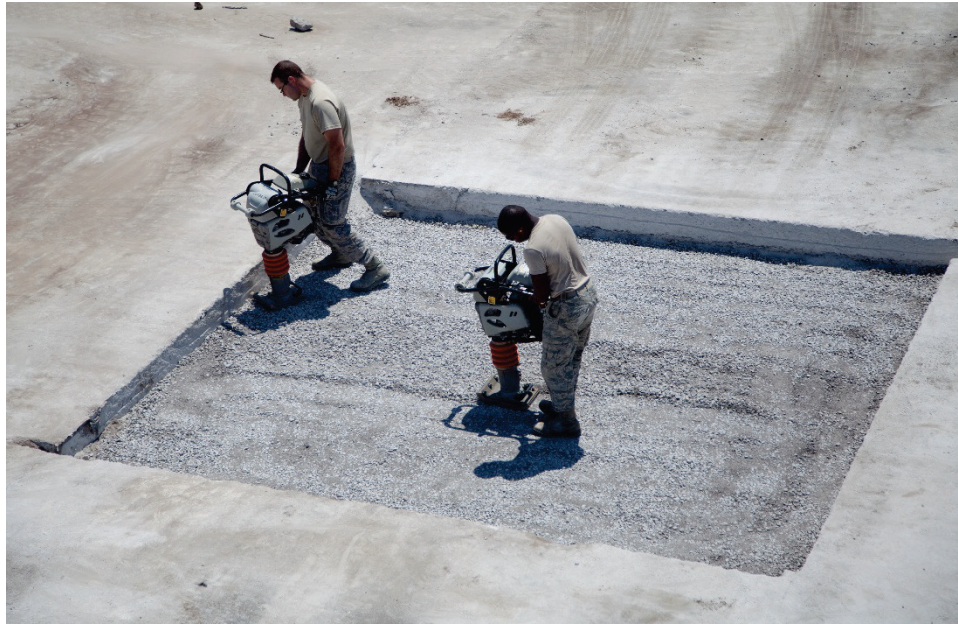
Figure 15. Compacting limestone with MultiQuip MTX-60.
