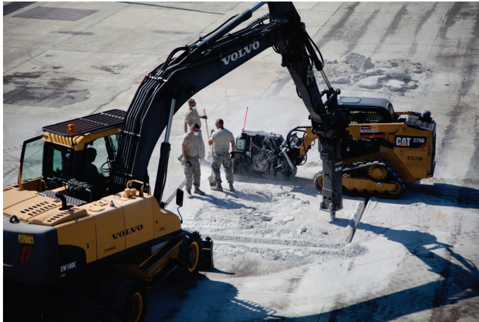
Figure 13. Breaking crater repair area.
