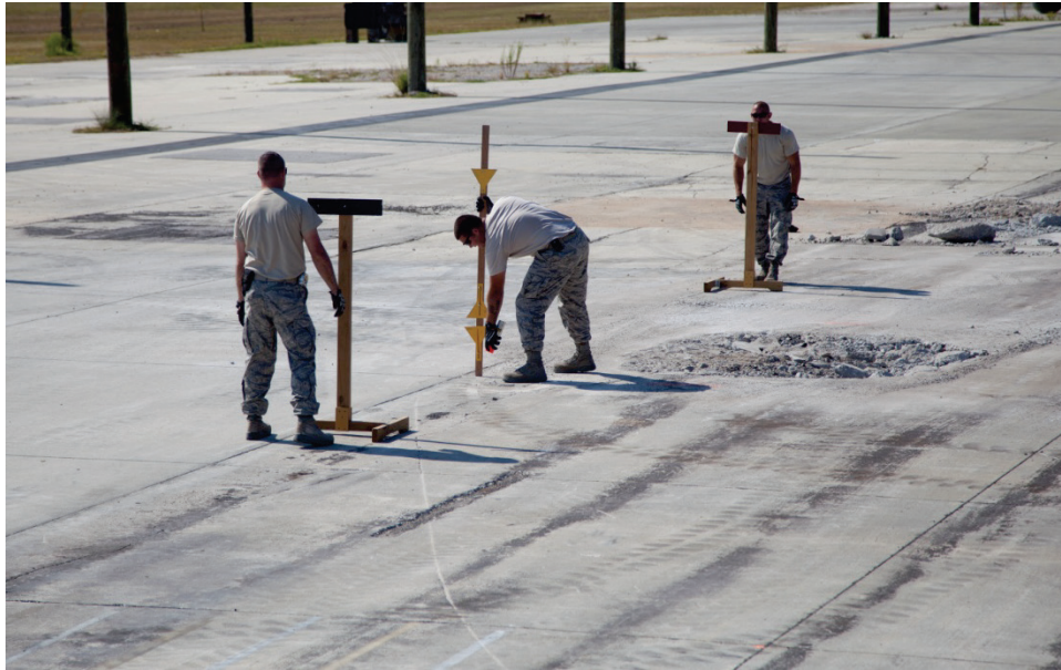
Figure 11. Marking crater repair area.
