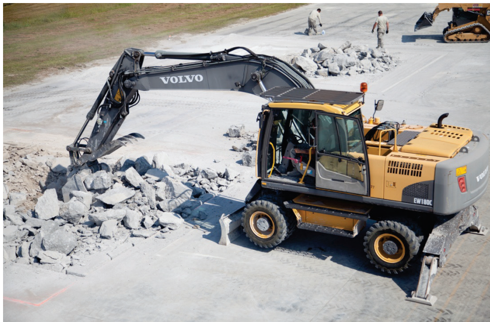
Figure 6. Wheeled excavator with bucket attachment.
