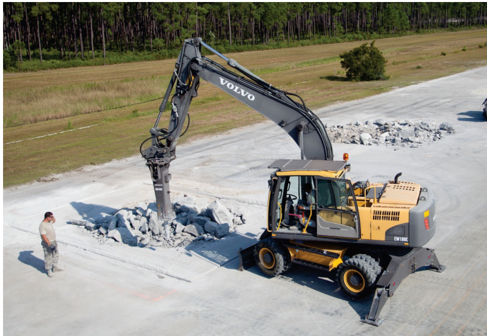
Figure 5. Wheeled excavator with breaker attachment.
