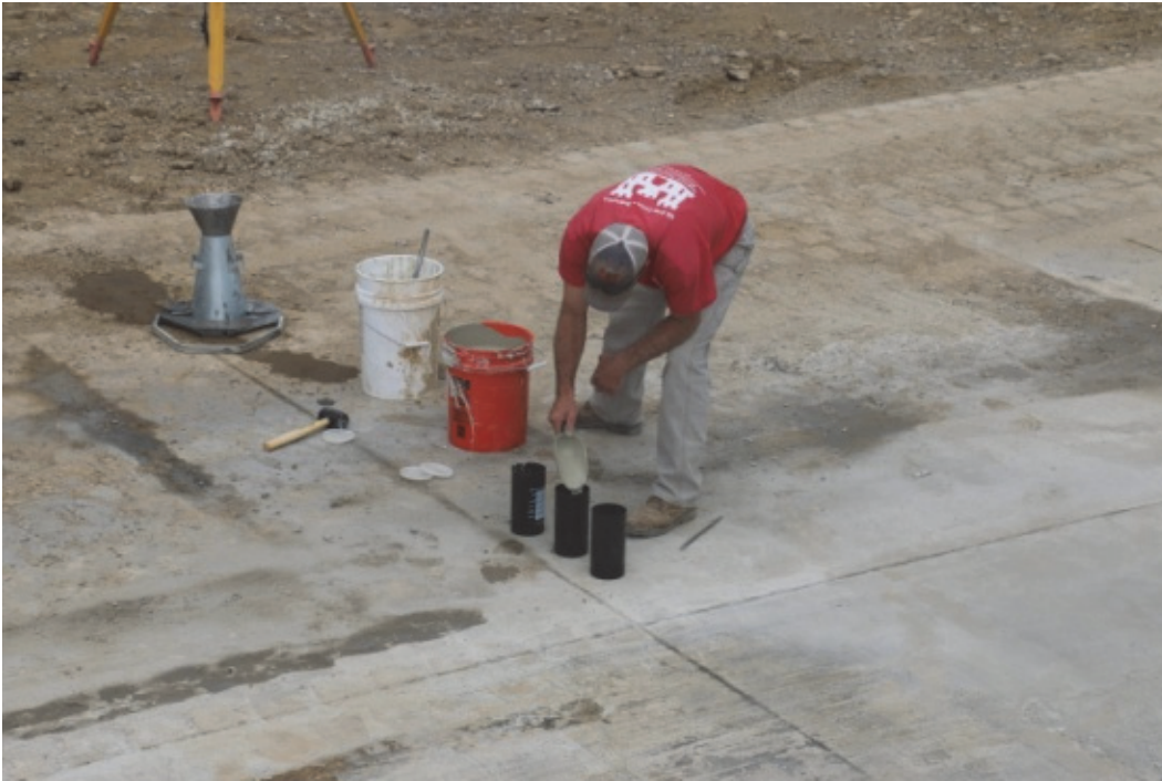
Figure 18. Preparation of compressive cylinders.
