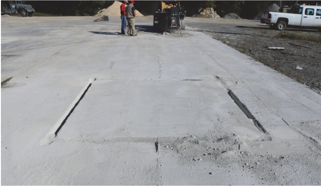
Figure 9. Typical saw-cut repair area.
