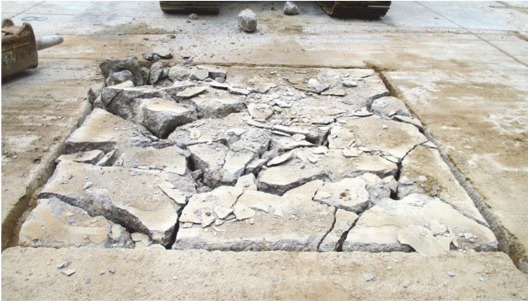
Figure 11. Broken PCC.
