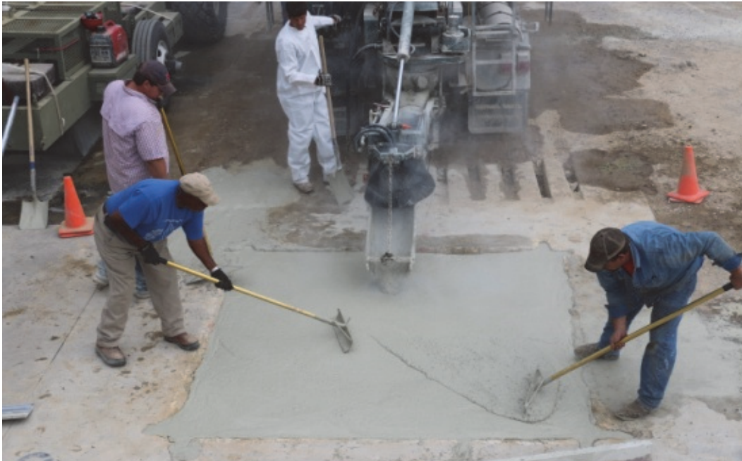
Figure 15. Placing rapid-setting concrete cap.
