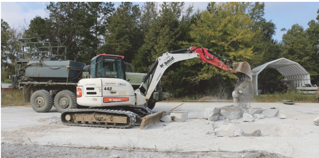
Figure 12. Excavating repair with compact excavator.
