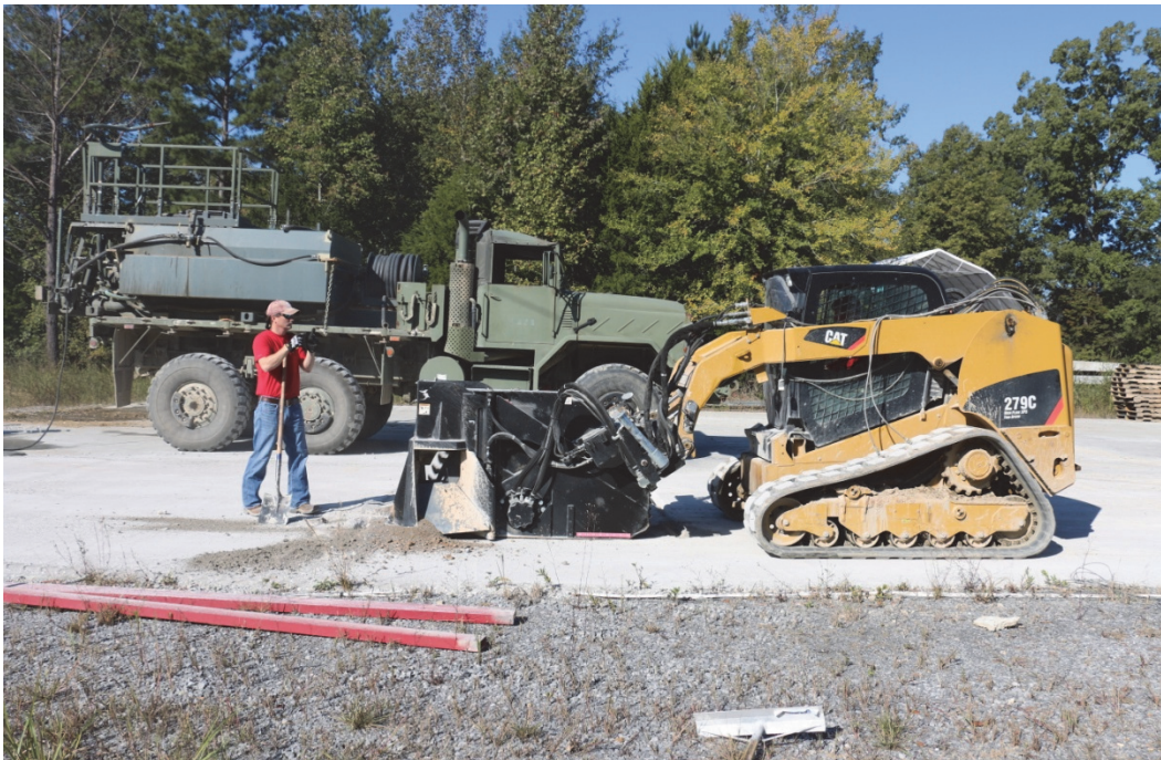
Figure 8. Saw-cutting repair area using CTL and wheel saw.
