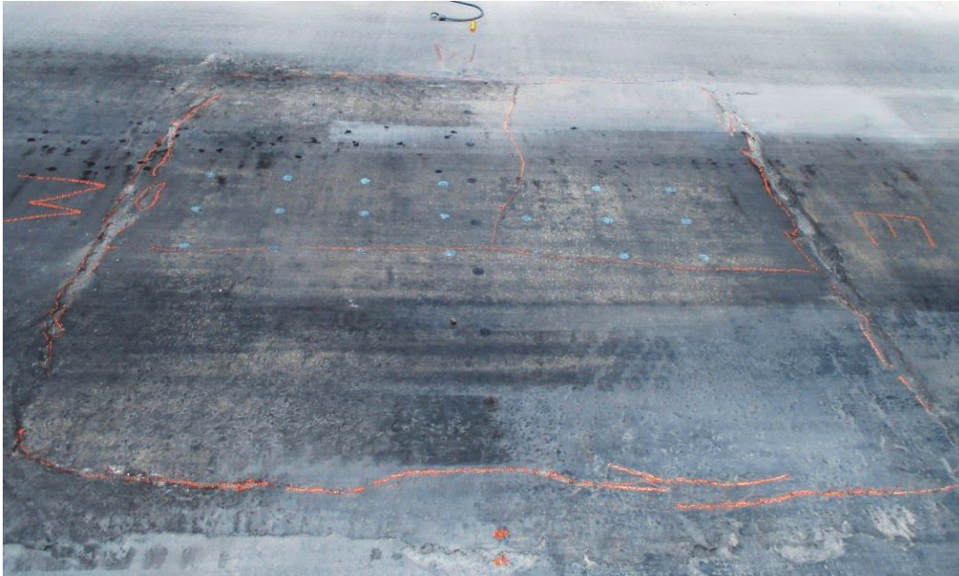
Figure 26. Series 2, Repair 8 - overall at 10,000 passes.
