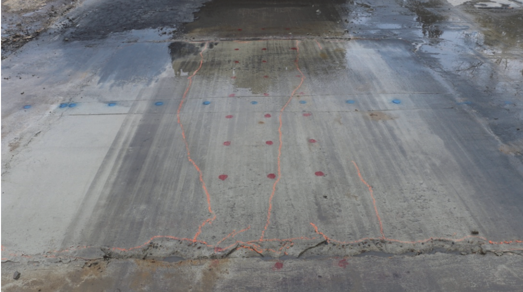
Figure 21. Series 1, Repair 2 - overall at failure (1,750 passes).
