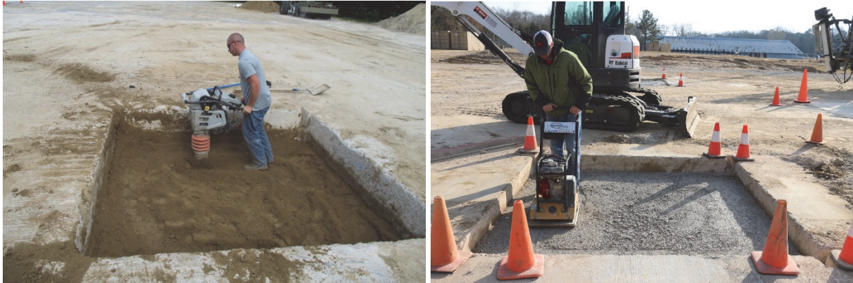
Figure 13. Compaction of subgrade (left) and limestone base (right).
