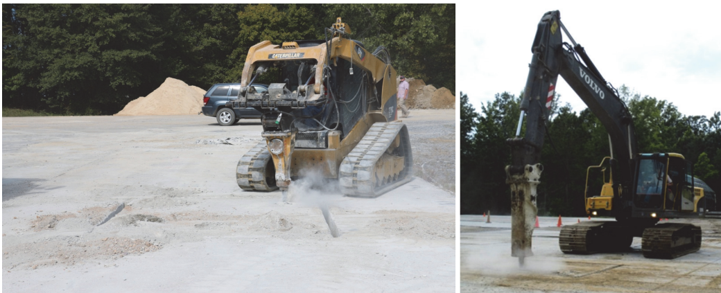
Figure 10. Breaking PCC using CTL (left) and excavator (right) with breaker attachments.
