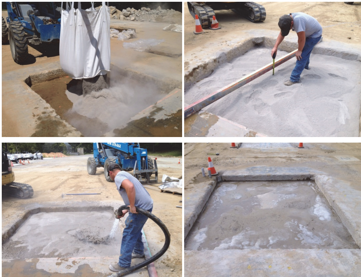
Figure 14. Flowable fill placement, clockwise from top left: dispensing dry material, checking depth, adding water, and completed base.
