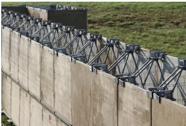
Figure 6.1. Modular Protective System (MPS) utilizing armor panels for rapidly deployable blast and ballistic protection.
