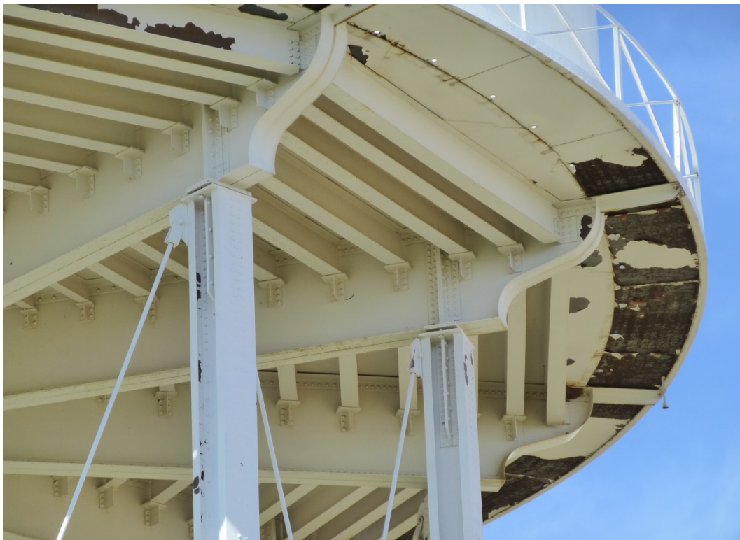
Photo 10. Detail of underside of Fort Huachuca elevated water tank (Facility 49001) (ERDC-CERL, 2015).
