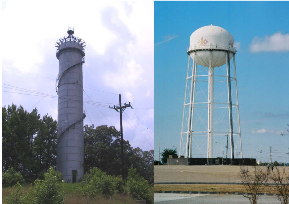
Figure 6. Standpipe at Naval Support Facility Indian Head, Maryland, on left versus an elevated water tank on right at Fort Gordon, Georgia (ERDC-CERL 2008 [left] and 2004 [right]).
