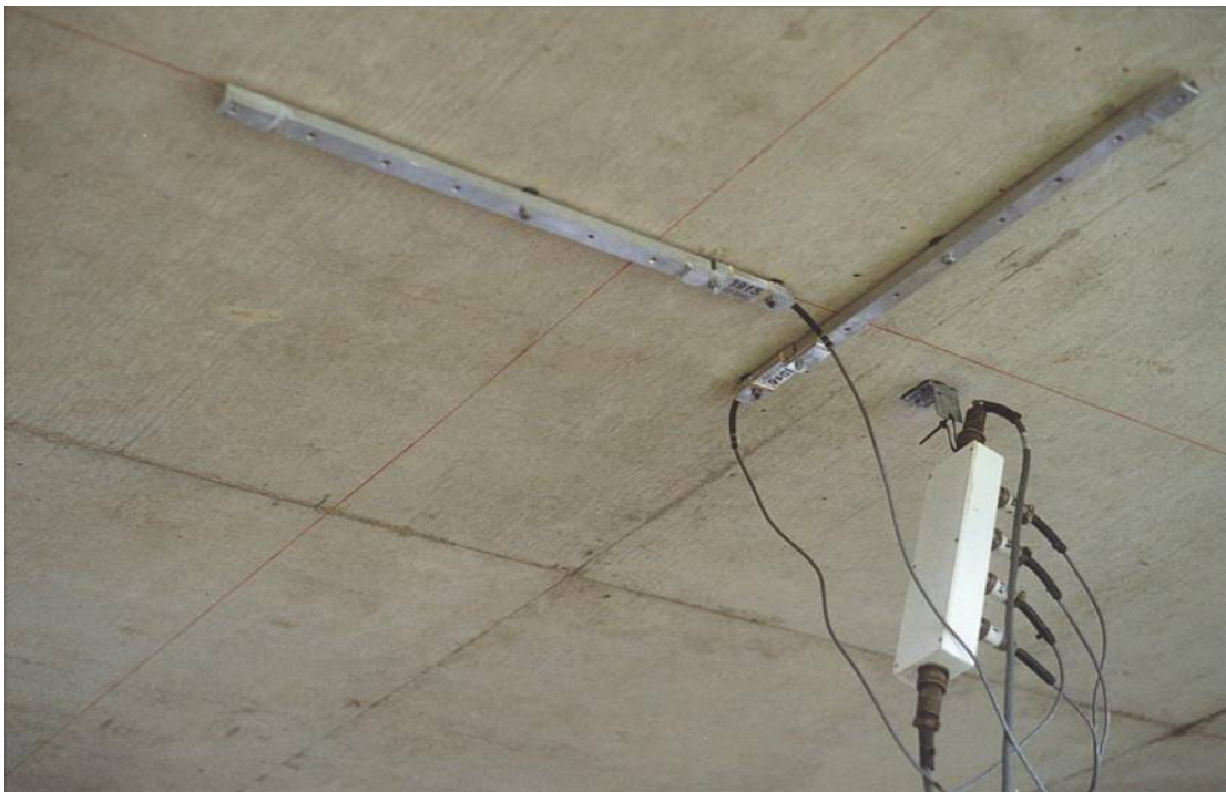
Figure C.2 Transducers w/Gage Extensions Mounted On R/C Slab
