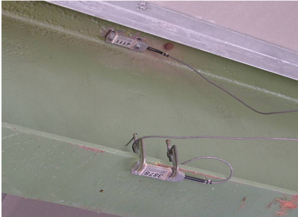
Figure C.1 Strain Transducers Mounted on Steel Girder
