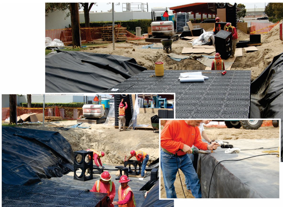
Figure 10. Construction and Installation of 17,000 gal UST for Storage of Harvested Water
