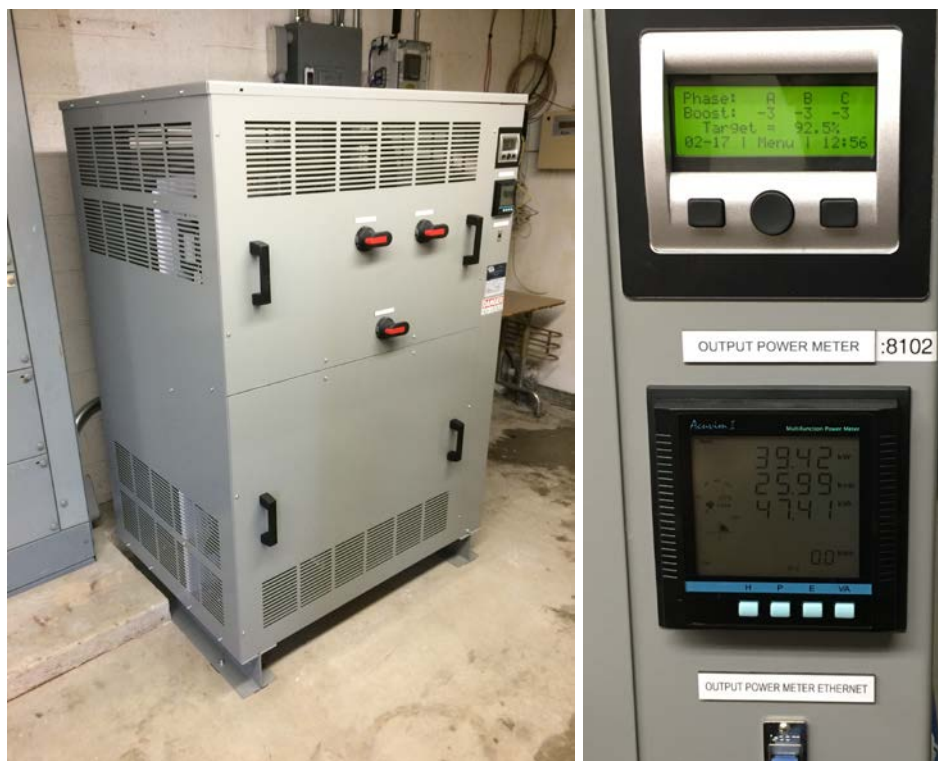
Figure 21 The EVR device installed in the building, and the meter panel display.
