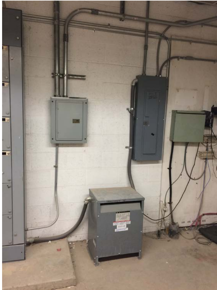
Figure 13 Photo inside of the electrical room at building B1588, showing a 480-208V transformer mounted to the floor, and electric load panels mounted to the wall.
