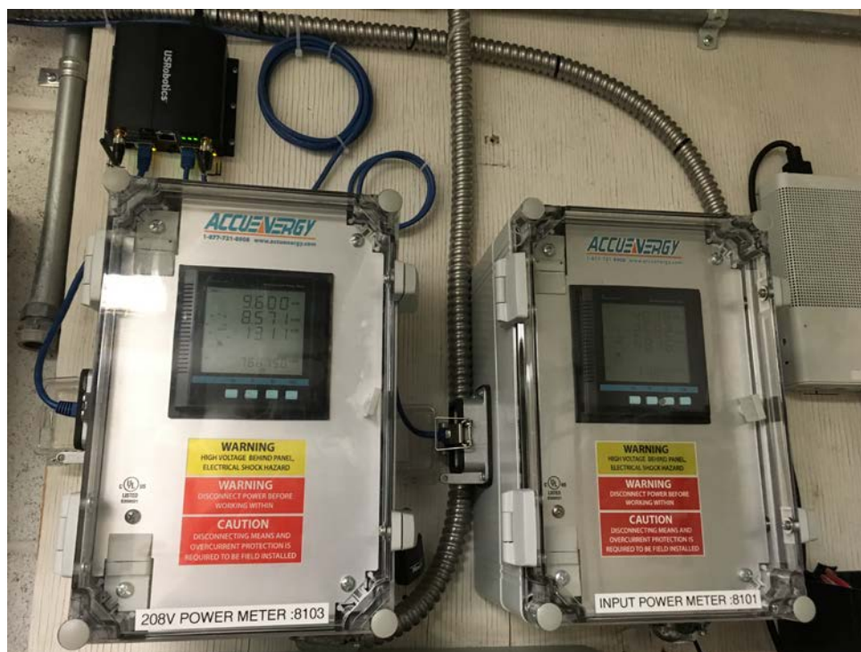
Figure 22 Installed Meters and Cellular Router for data retrieval.
