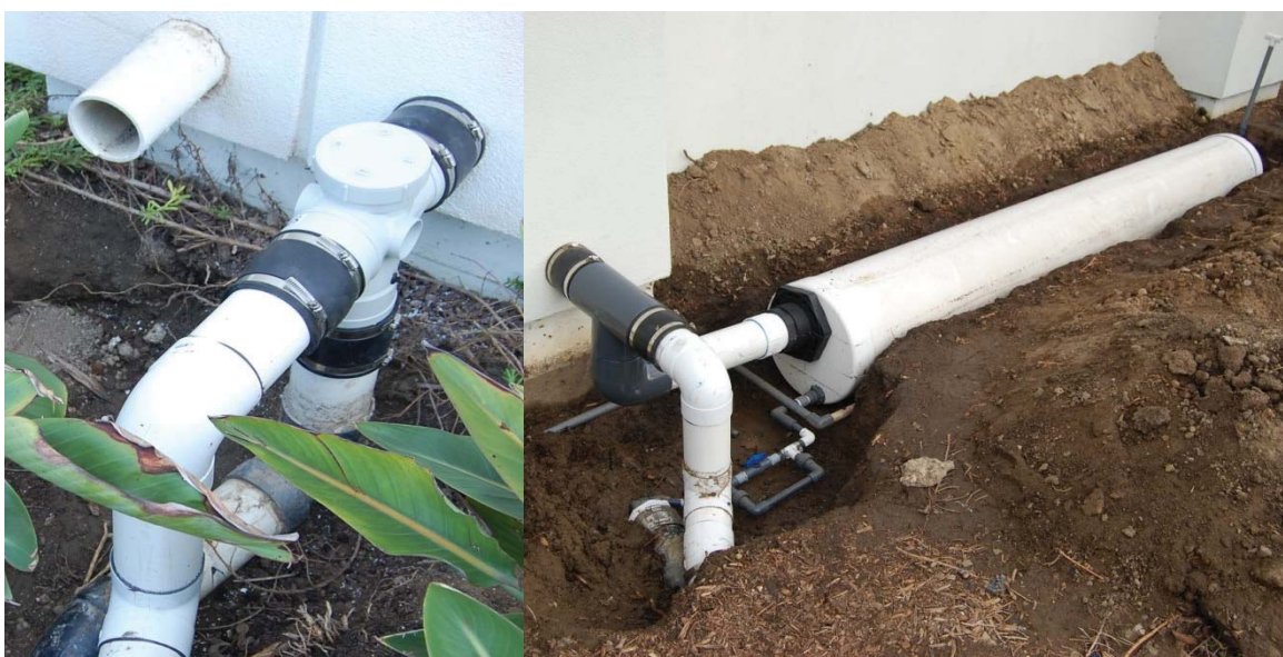
Figure 9. Diverter Valve and Constant Volume First Flush Diverters Installed at Base of Building 1100
