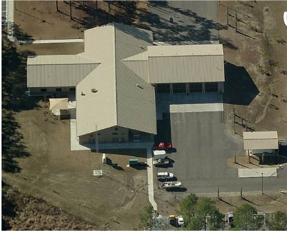
Figure 5.9. Building 2085, MCAS Beaufort.
