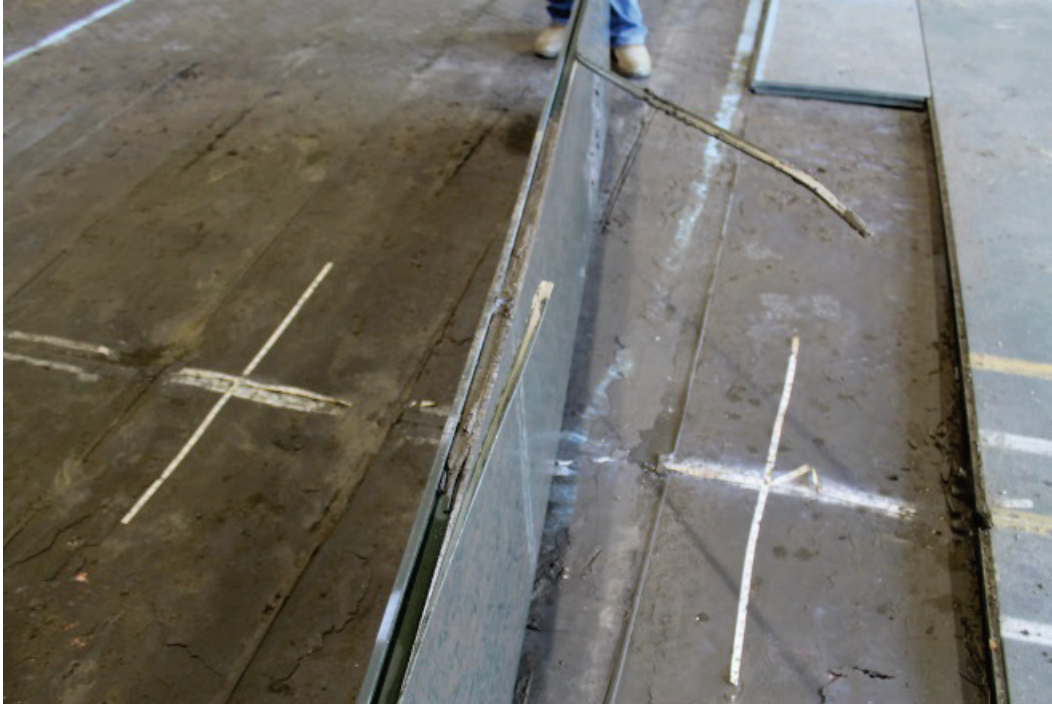
Figure 4.9. G65 after removing from test section.
