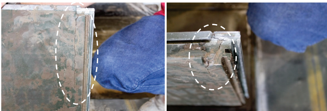
Figure 4.3. Broken end connector in F118.
