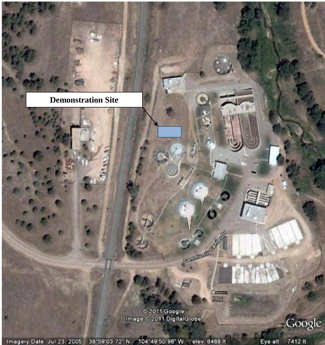
Figure 4. Aerial View of Demonstration Site.
