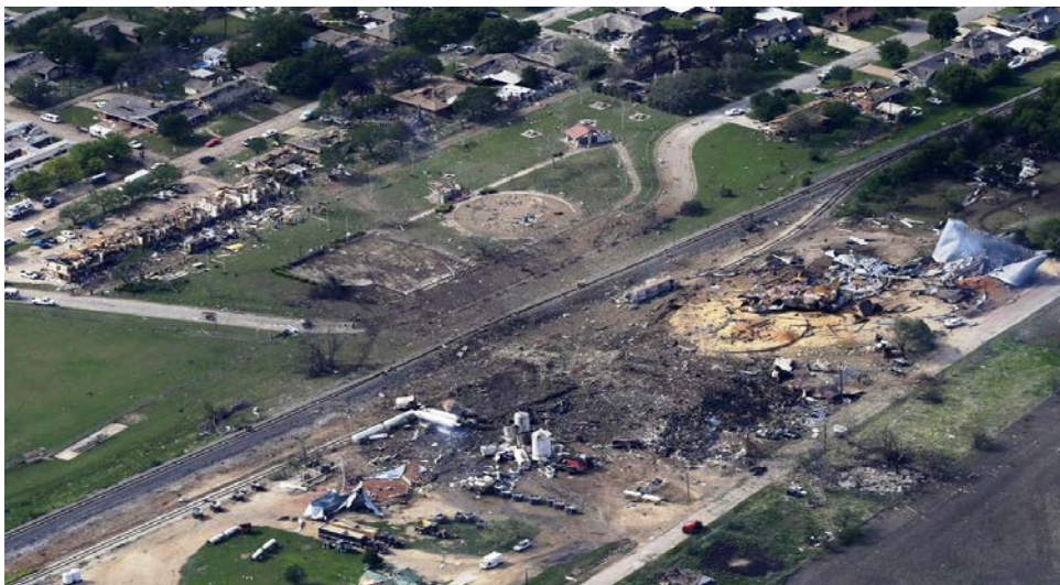
Figure 6. Impact Blast of the West Fertilizer Company Plant
