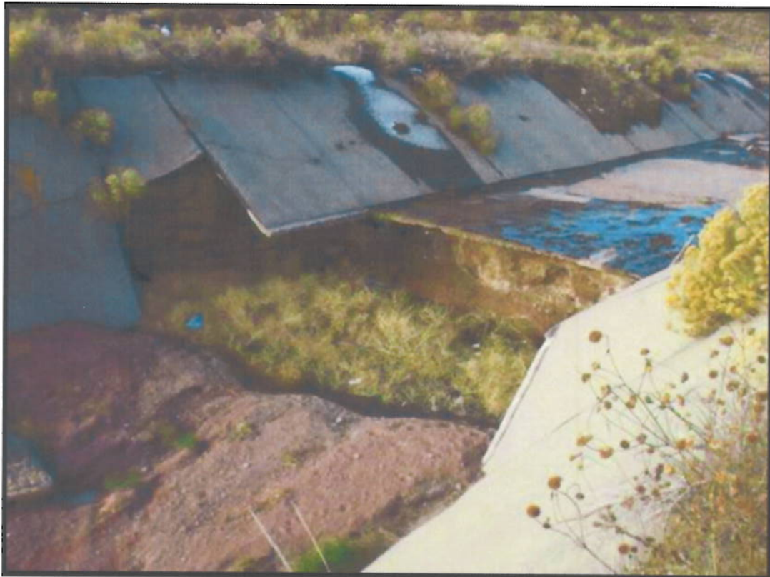
Figure 5. Drainage Channel in Colorado Springs Courtesy City of Colorado Springs
