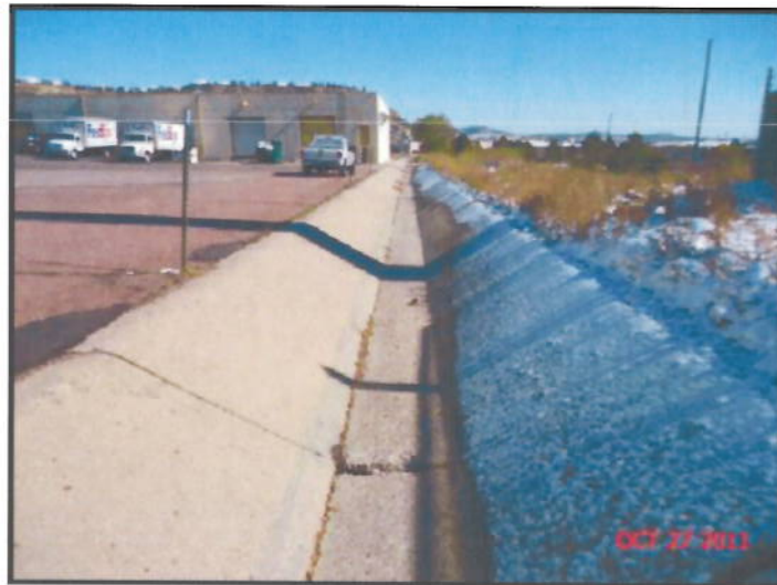
Figure 3. Drainage Channel in Northwest Colorado Springs Courtesy City of Colorado Springs
