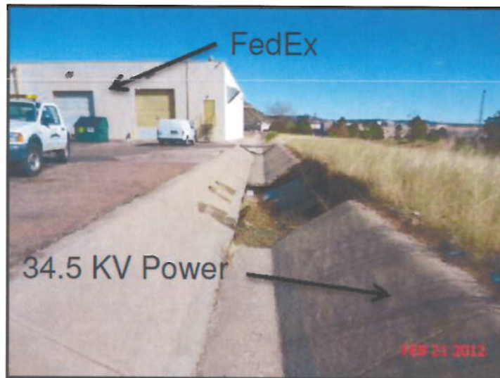
Figure 4. Same Channel Four Months Later Courtesy City of Colorado Springs
