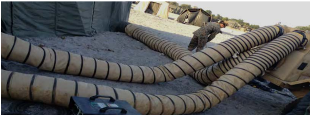
Figure 7. ECU Duct Losses
