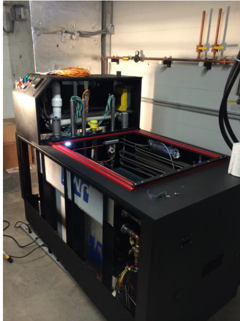
Figure 4-2: Pilot Test Setup at SGI
