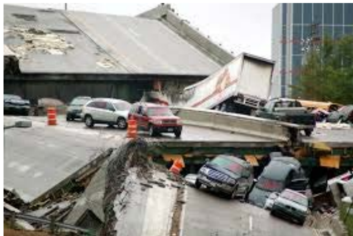
Figure 1. I-35 Bridge Collapse 7
