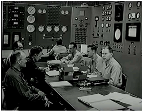
Control Room, Idaho National Laboratory 189
