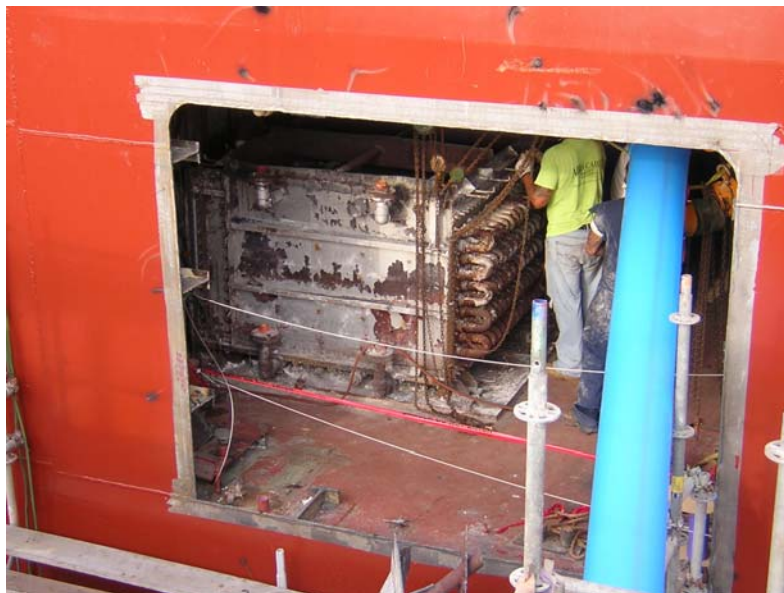
Figure 3. Waste Heat Boiler Being Removed from USS Hue City (CG 66). Source: [7].
